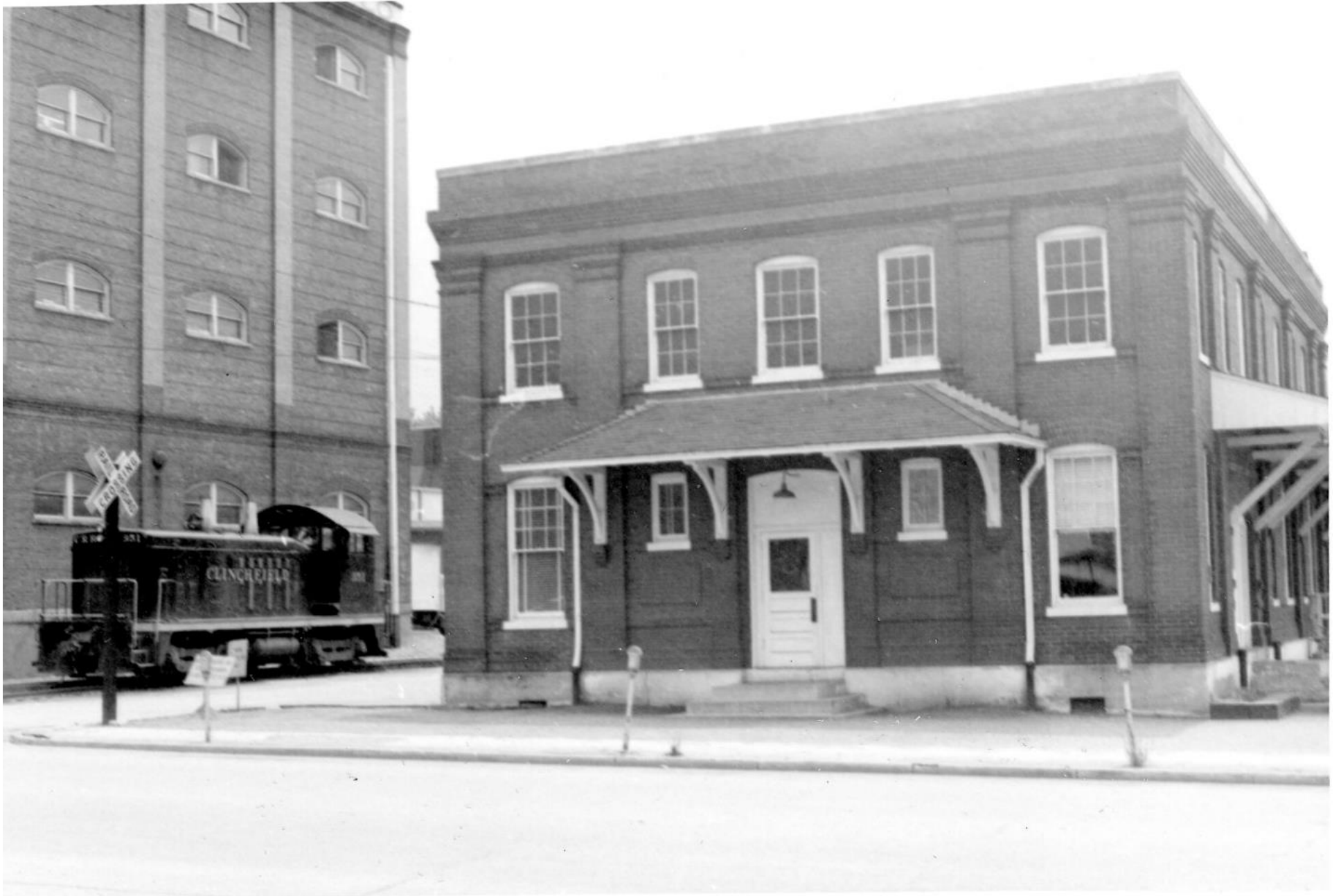
Figure 19. The Clinchfield Depot, with the Summers-Parrott Hardware building to the left. This photograph was dated July 1974. 45
