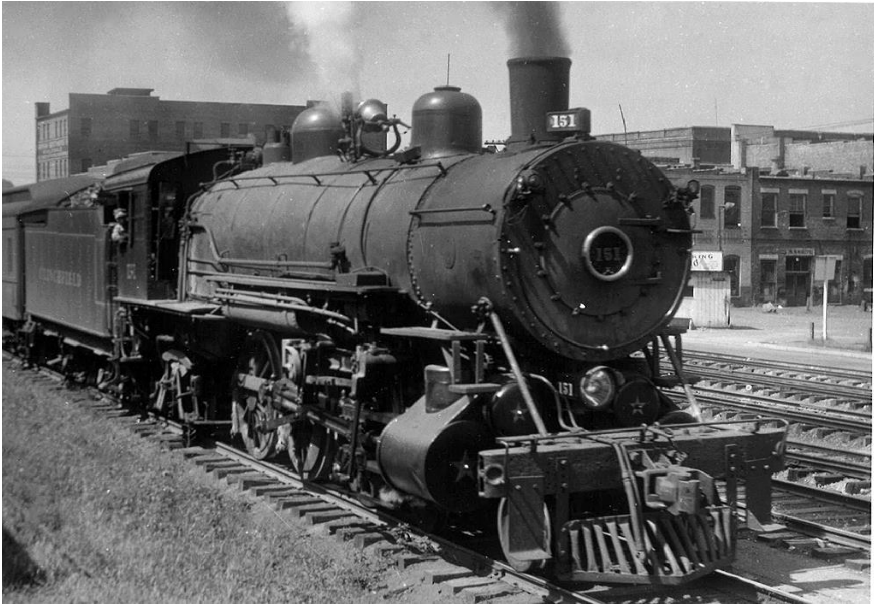
Figure 25. “4-6-2 Pacific steam locomotive No. 151 – Clinchfield locomotive No. 151 heads [passenger] train 37 at Johnson City, Tennessee, on August 31, 1941. The road had five Pacifics: Class P-1 Nos. 150 – 152 (Baldwin, 1910) and P-2 Nos. 153 – 154. Note the location of the headlight, tucked under the smokebox. Louis A. Marre collection”. 55 Note the Hannah Dossor building in the left background, as well as the dual-gauge trackage. The street coming in from the right is probably South Roan.
