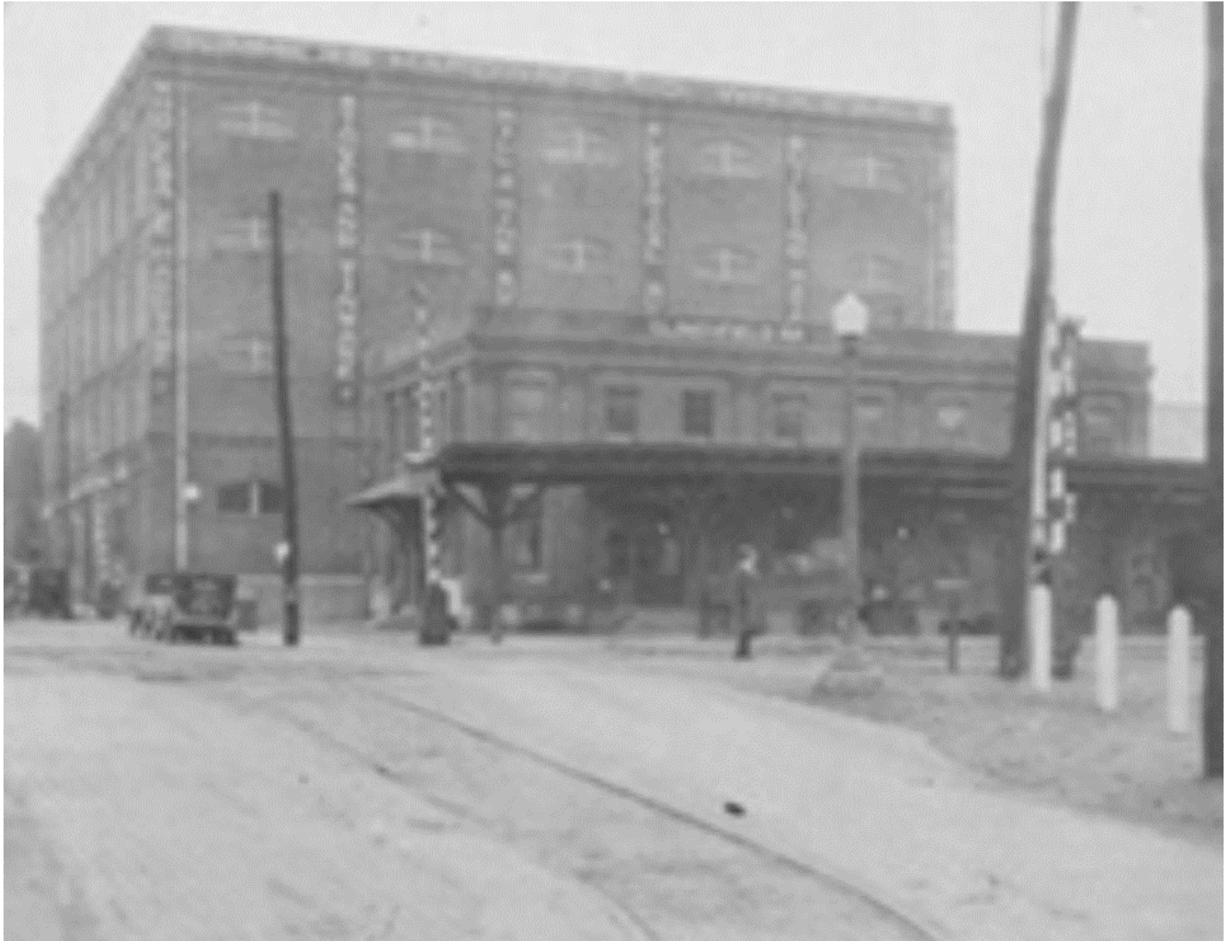
Figure 14A. A detail of the C.C. & O. Railway Depot.
