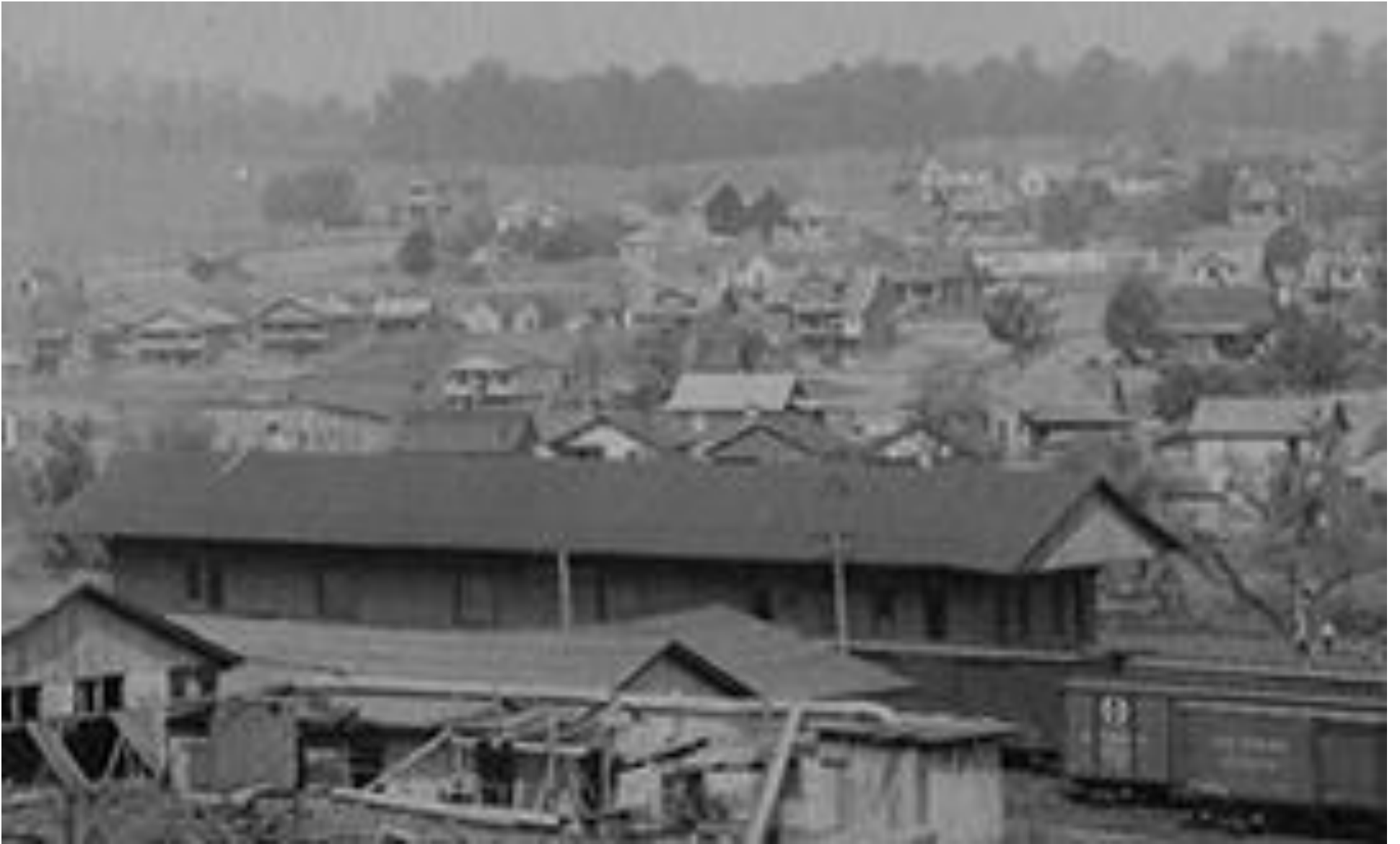
Figure 10A. A detail of the Old Clinchfield Freight Depot.
