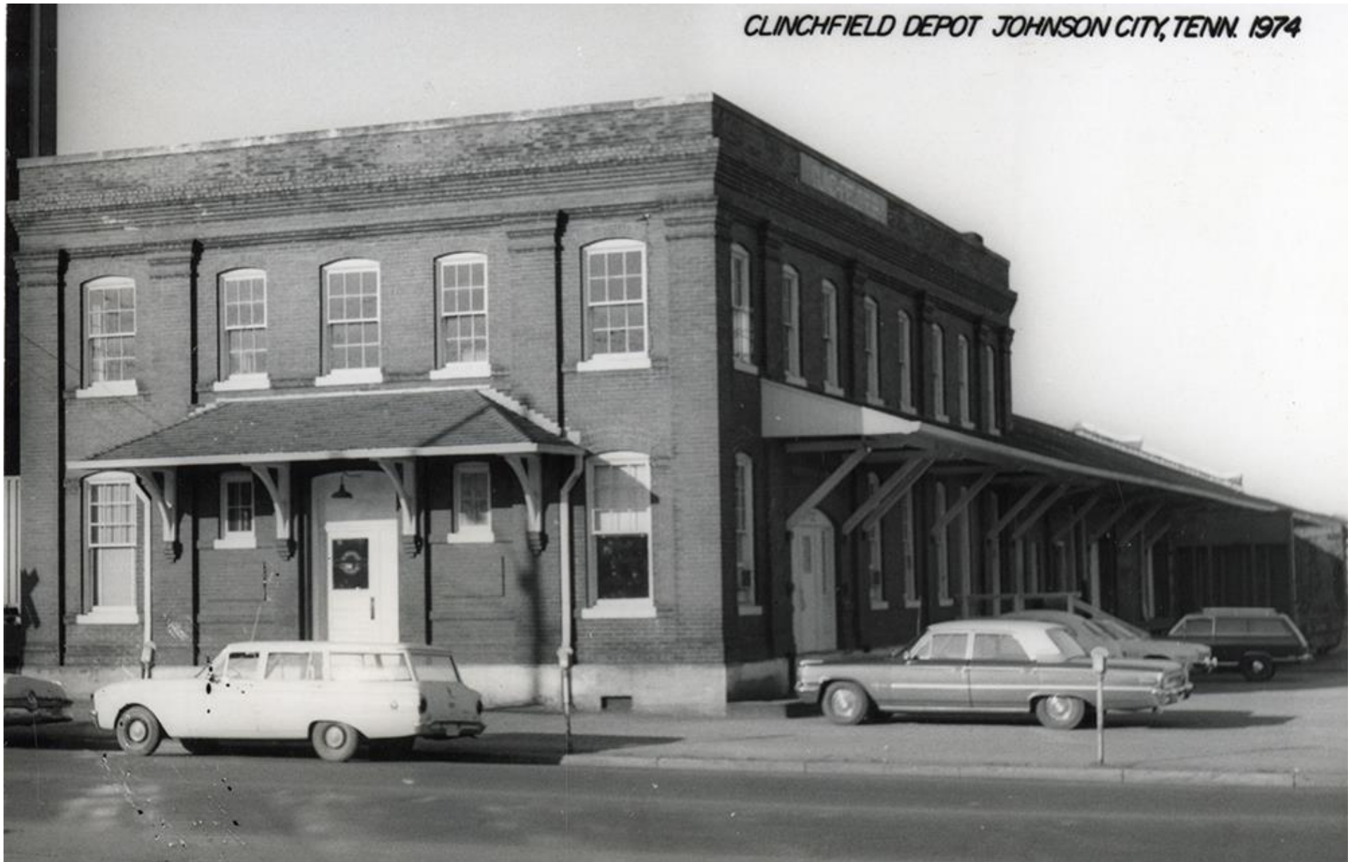
Figure 18. "Clinchfield Depot" in 1974. 44
