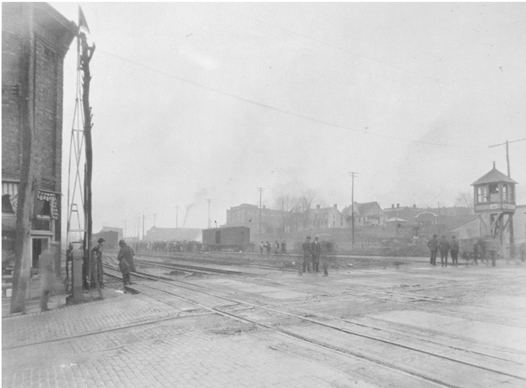
Figure 38. The intersection of Buffalo Street and the tracks of the E.T. & W.N.C. and Clinchfield railroads. The safety tower, built by the Clinchfield, is visible at the right and one of the gates is visible on the left. Note the trolley tracks running along Buffalo Street. 72
