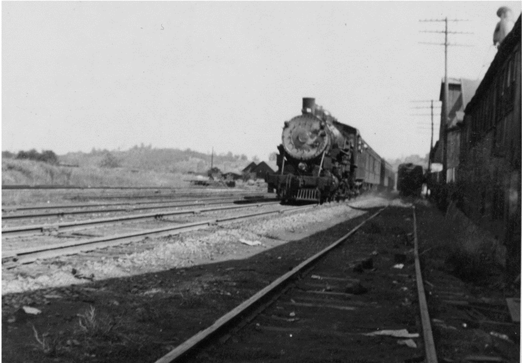
Figure 23. "Clinchfield Railway No. 150" pulling a northbound passenger train, apparently passing the Harris Manufacturing plant. Note that all of the trackage appears to be standard gauge. 52 Engine #150, a Baldwin 4-6-2 Pacific, was built in June 1910, with an empty weight of 117½ tons. The Clinchfield employed Pacific type engines in passenger service north of Erwin, Tennessee. This engine was retired in June 1951 and scrapped.
