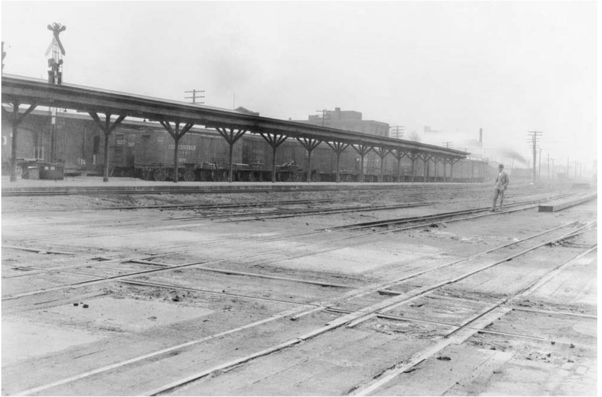
Figure 15. This photograph, looking southwest, shows the trolley tracks on Buffalo Street and dual-gauge trackage, with the Clinchfield platform in the background. 41 Note the Love-Thomas office building on the middle background of this photograph.
