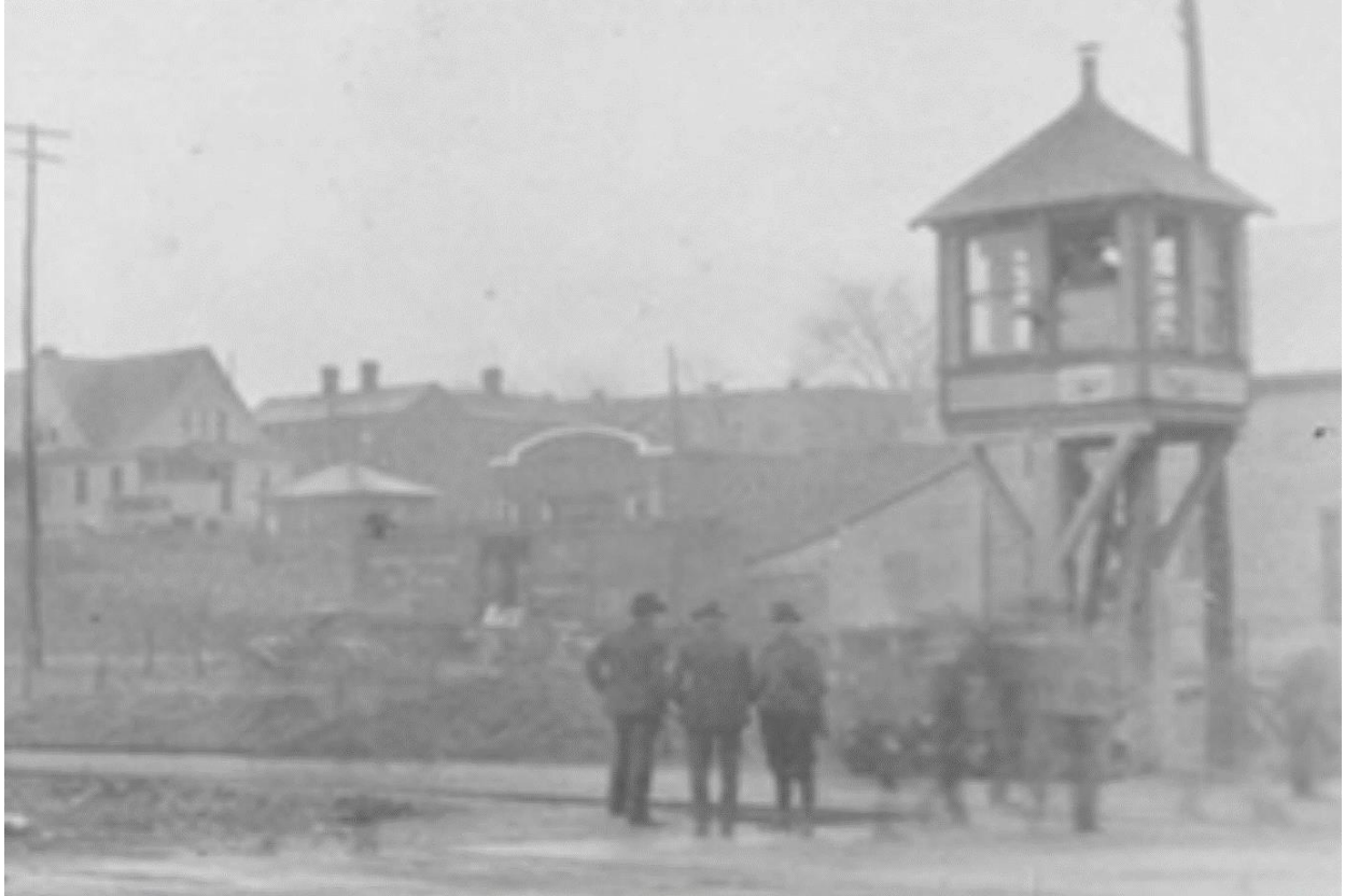
Figure 38A. A detail of the safety tower on Buffalo Street.
