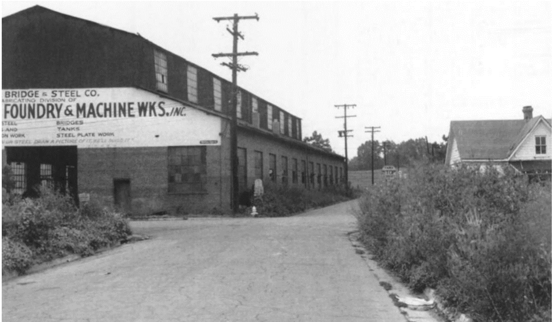
Figure 16. “The Johnson City Foundry & Machine Works, inc. built bridges, tanks, iron work, and steel plate work, among other things. Shown here is an end of the foundry building with their sign advertising, ‘iron or steel, draw a picture of it, we’ll build it.’ (Courtesy of Doug Thompson.)” 40 Note, the Sanborn map of February 1920 indicates that the foundry was in a different building; additionally, the sign on this building indicates that it was occupied by the Fabrication Division. The building on the right would be used by the C.B. Voncanon Company as their office, when they occupied this property from 1920 – 1928. This photograph looks north across West Walnut Street, along Tennessee Street, and appears to have been taken after Figure 15 and probably dates to after 1928.
