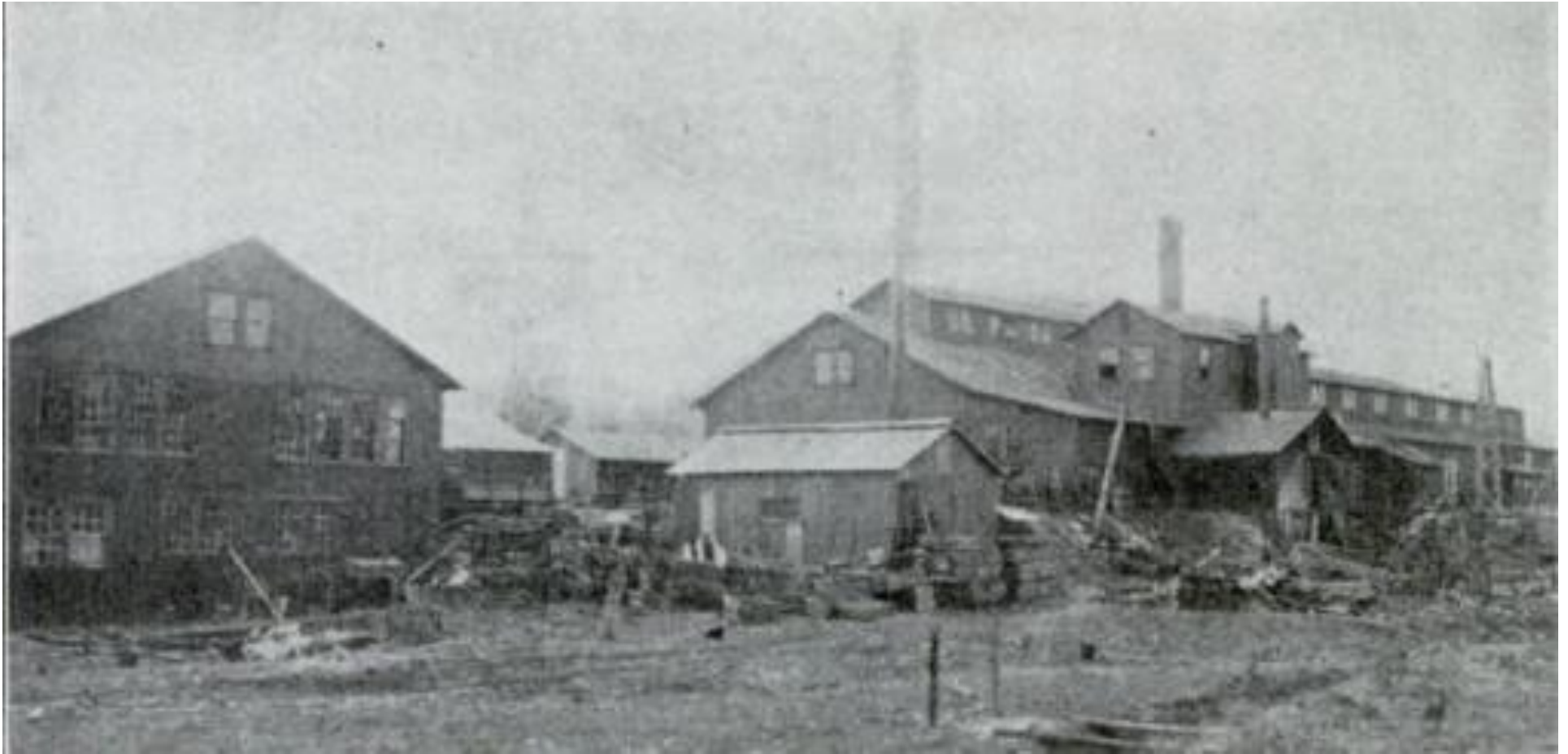
Figure 12. A view of the back side of the Johnson City Foundry and Machine Company published in 1909, also known as the “Dominion Iron Works” at this time. This photograph was taken from the north (back) side of the plant, looking south toward West Walnut Street. This photograph shows the pattern storage building, on the left, with the foundry and machine shop building on the right. The shed in the center of the photograph housed the boiler, but was reportedly not in use by July 1913. 36 See Figure 13 and Map 3A.
