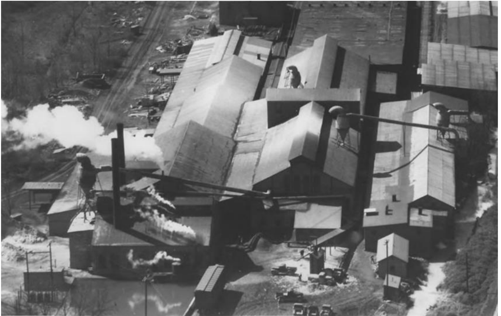
Figure 7A. A detail of the Miller Brothers Lumber Company. In the left foreground appears to be the “Open Concrete Reservoir” (note the reflection of the exhaust plumes), with the power house behind it. The building in the center appears to have previously been the “Barium Carbonate Department” of the Rollin Chemical Corporation, see Map 2.
