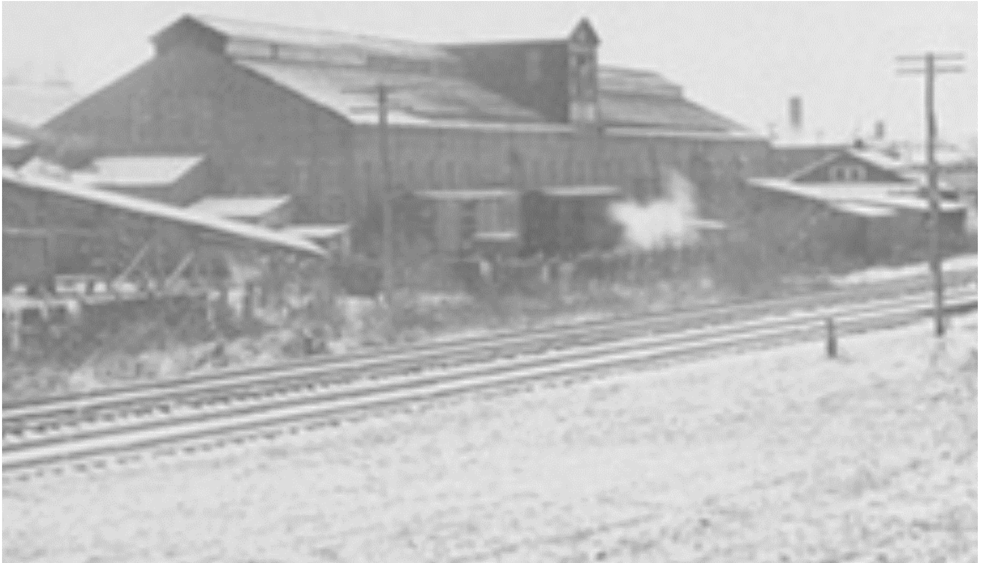
Figure 3A. The former “Barium Carbonate Department” building.
