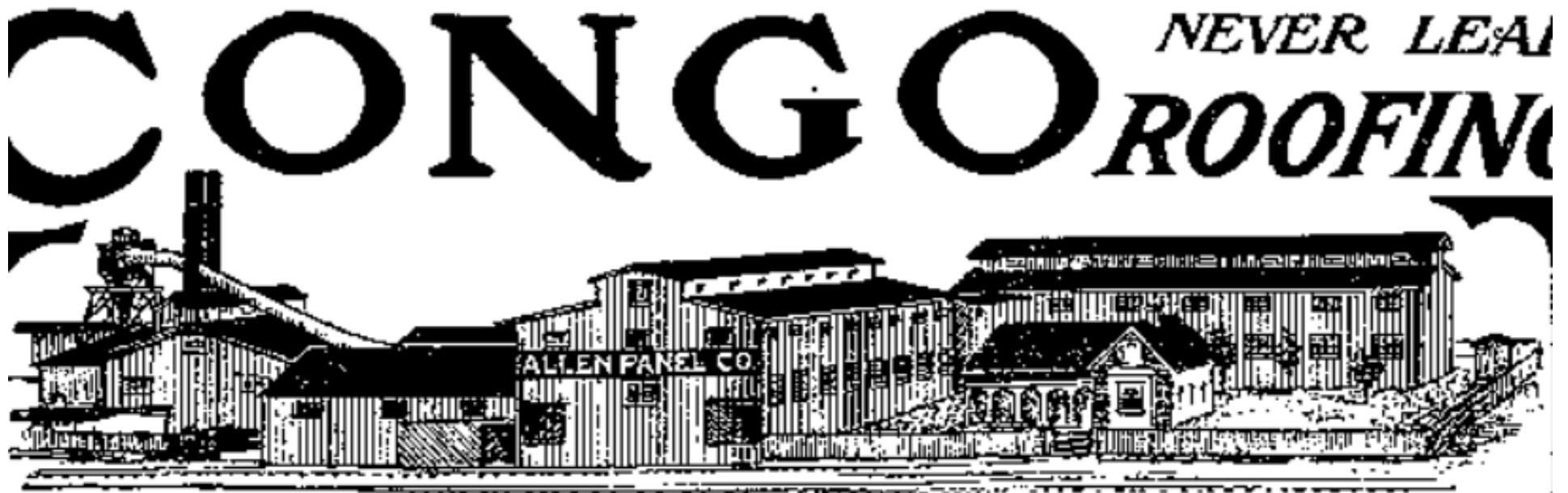
Figure 51. These two images of the “Allen Panel Co.” appear to actually be of the Interior Hardwood Company, looking south. The building at the left houses the boiler, the one in the center with the “Allen Panel Co.” sign is the Planing Mill, the long one on the right in the back is a storage facility, and the small one to the right of the Planing Mill is the office. See Map 10.
