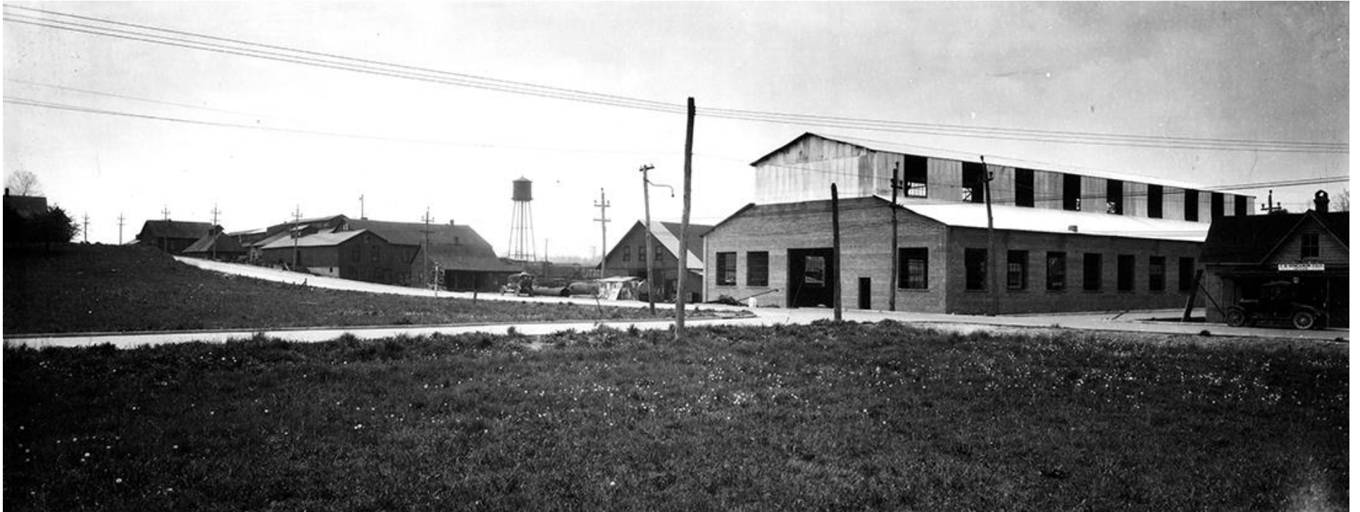
Figure 15. “Johnson City Foundry and Machine Company, 920 West Walnut Street” 39 Note the C.B. Voncanon office on the right, on the northeast corner of Tennessee and West Walnut streets. The water tower in the background probably belongs to the Rollin Chemical Corporation/Miller Brothers Company. The Fabrication Division Building was reportedly built by 1926, see Figure 14.
