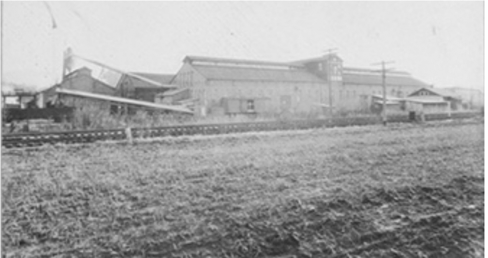
Figure 4. “Miller Brothers Company... Manufacturers of Hardwood Flooring, Johnson City, Tennessee.” 6 The large building, on the right, appears to have previously been the “Barium Carbonate Department”, and the building to its left, with the cyclone, is the power house. See Map 2.
