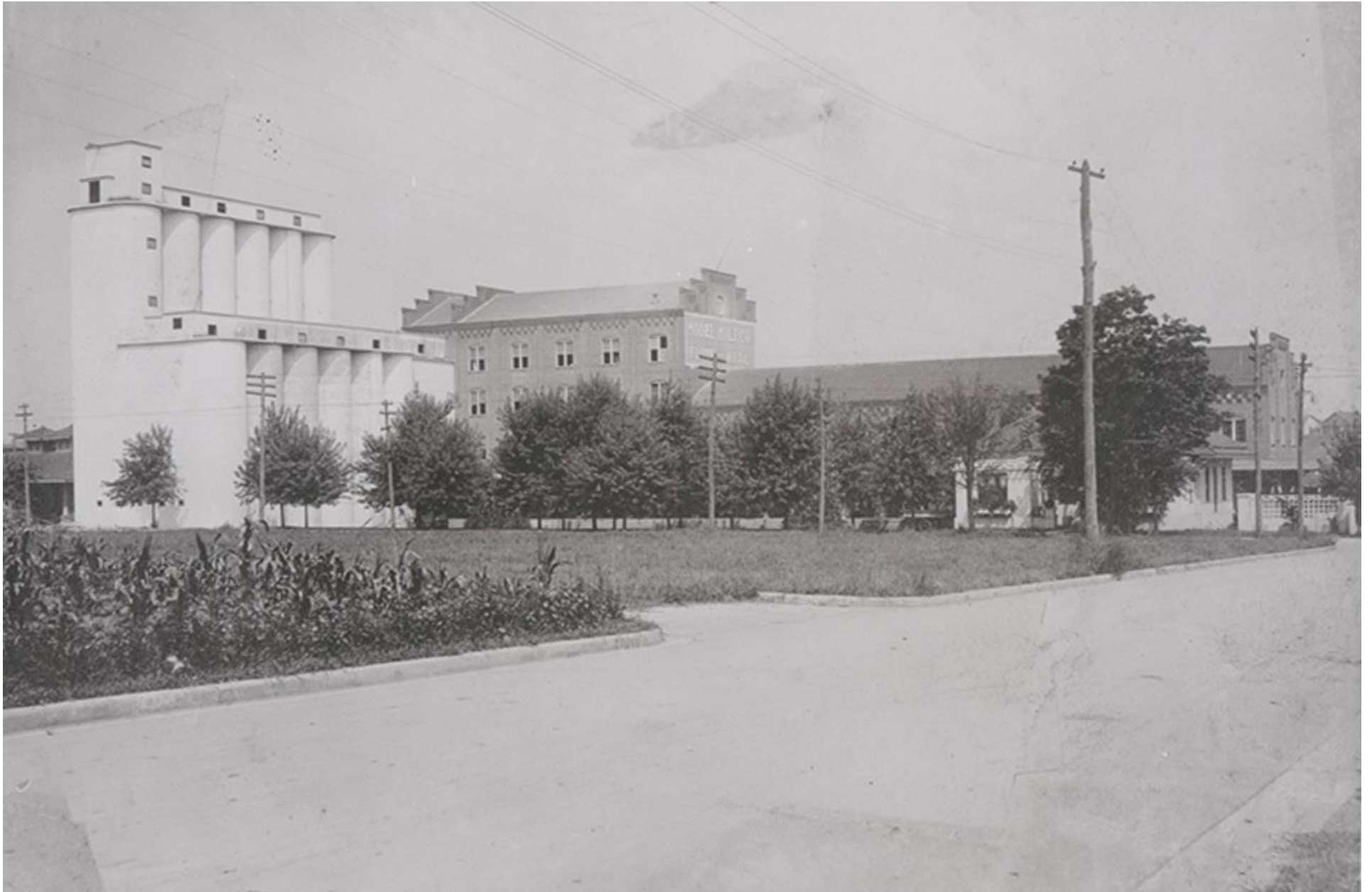
Figure 60. “Model Mills (Red Band Flour, also known as General Mills), corner of West Walnut and Sevier Streets”. 236 This photograph appears to have been taken from Sevier Street, south of West Walnut Street, looking northwest.
