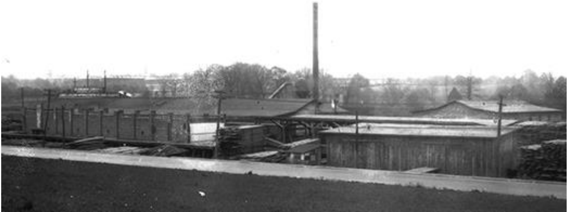
Figure 34A. A detail of the Voncanon Company plant. The building on the left appears to be the Steam Dry Kiln, with the sawmill and powerhouse, with the smokestack and cyclone, behind it. The two buildings on the right do not seem to match those depicted on the Sanborn map of February 1920. Behind the Steam Dry Kiln is a structure near three utility poles, which appears to be the sawmill of the Voncanon Company. Some buildings of the “Mountain Branch, National Home for Disabled Volunteer Soldiers” appear on the skyline behind the Steam Dry Kiln. See Map 5.
