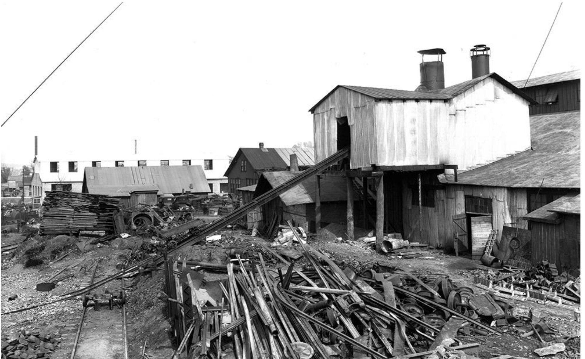
Figure 13. “Johnson City Foundry and Machine Shop, 920 West Walnut Street”. 37 This photograph shows the incline up to the foundry, as well as the standard gauge Clinchfield Railroad spur. The structure behind the incline appears to be the pattern storage building. The building to left of the pattern storage buildings should be the Boiler Shop, and the light-colored building in the background belonged to the Fabrication Division. The Fabrication Division Building was reportedly built by 1926, see Figure 14. See also Figure 12 and Map 3.
