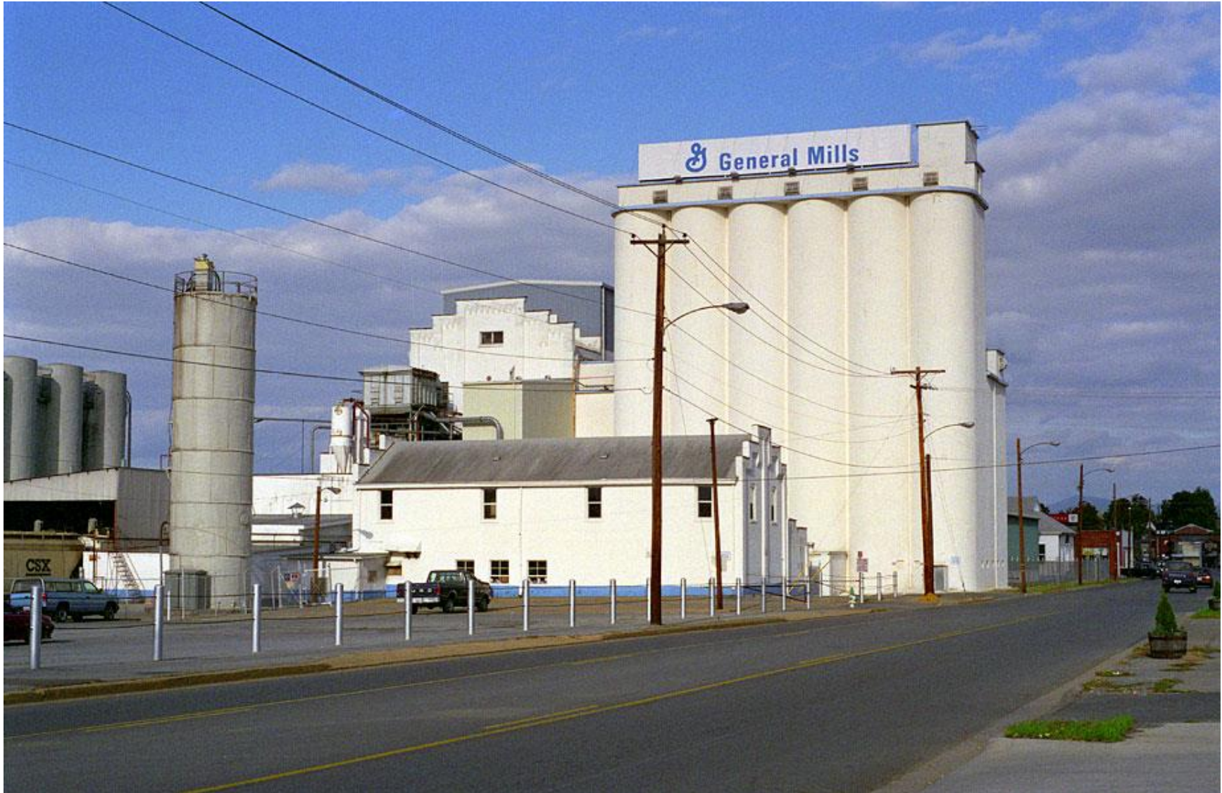
Figure 65. October 1995 – Model Mill Silos in Downtown Johnson City. Historian Chris Ford captioned this photograph: “Here is the old Model Mills complex just west of the ET station. It was served by the CC&O and the ET&WNC. Although a few new manufacturing structures have been added to it, the main mill buildings are the original old structures. The original silos are the shorter ones on the far side and are still in use...” 241
