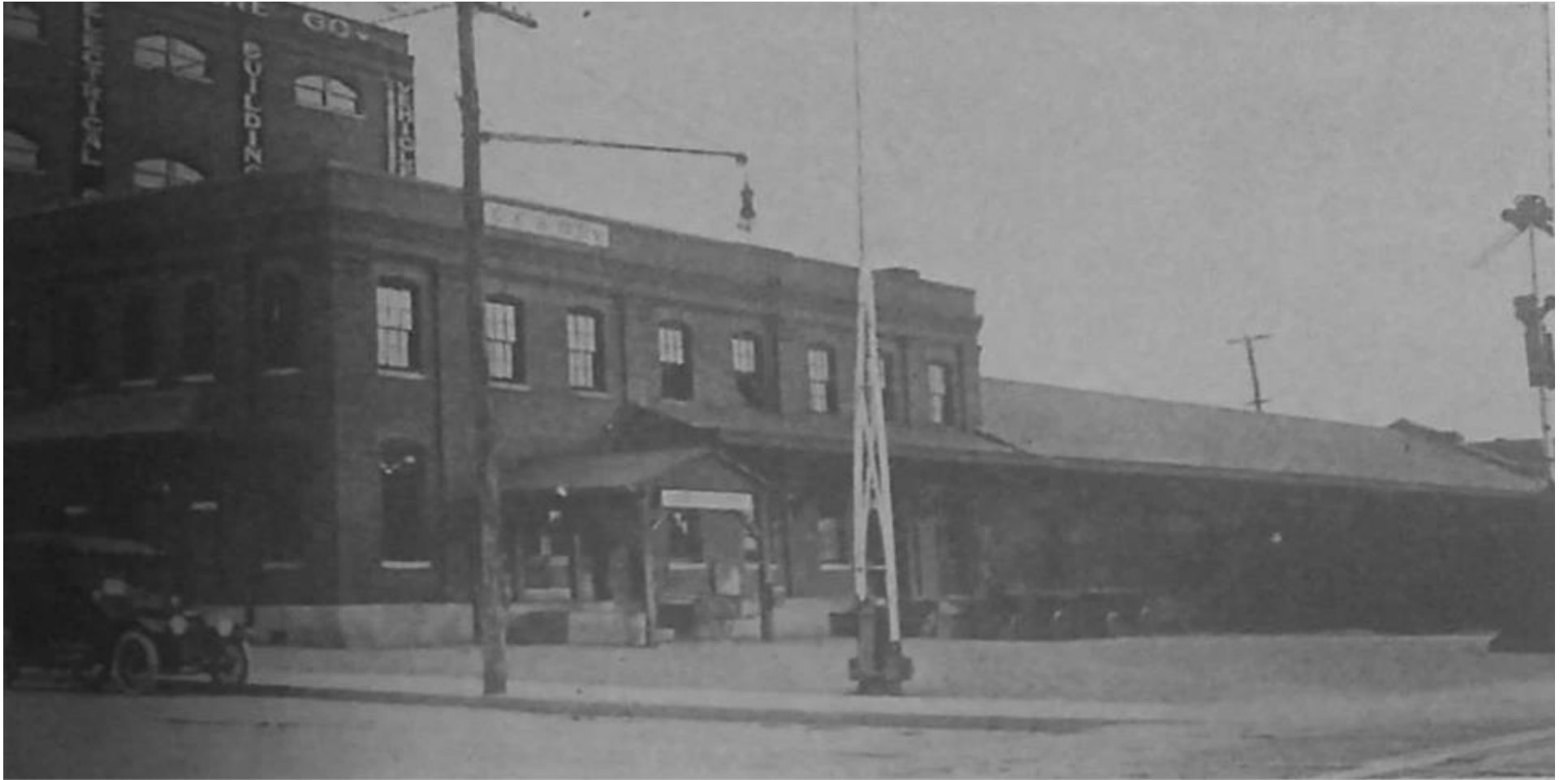
Figure 29. The Clinchfield depot, looking south across Buffalo Street. 58
