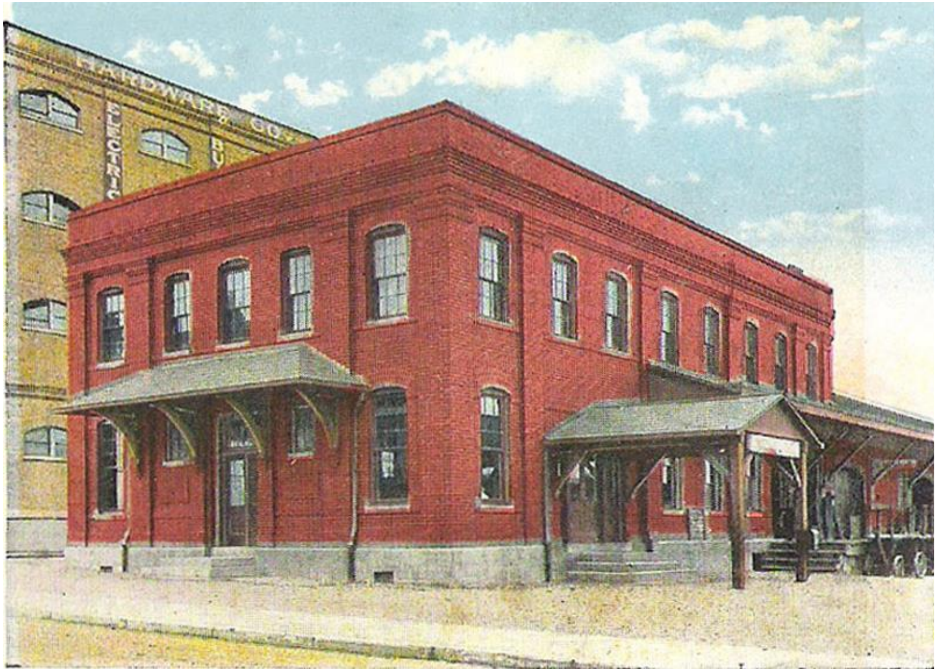
Figure 28. "C.C. & O. Depot." 57
