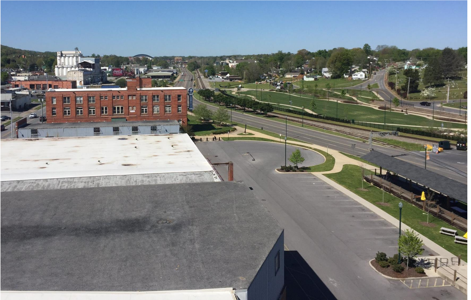
Figure 2. A modern photograph of the Love – Thomas Building, the large brick building on the left, taken from the Summers Hardware building. Note the Model Mill in the left background and the platform of the former Clinchfield depot on the right. 12 Also note the different windows of the Love – Thomas building, in comparison to those depicted in Figure 1A.
