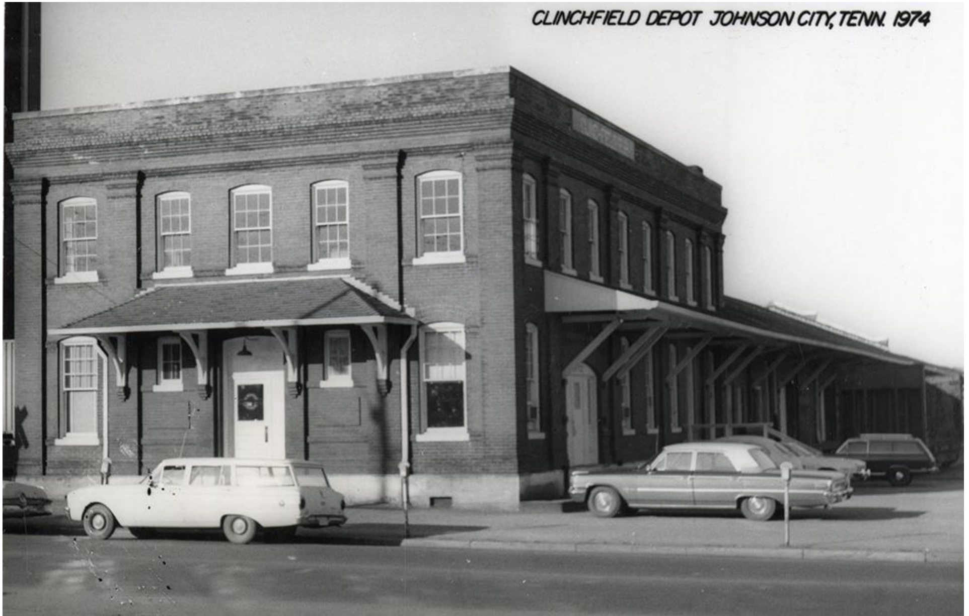
Figure 26. "Clinchfield Depot" in 1974, looking southwest across Buffalo Street. 55
