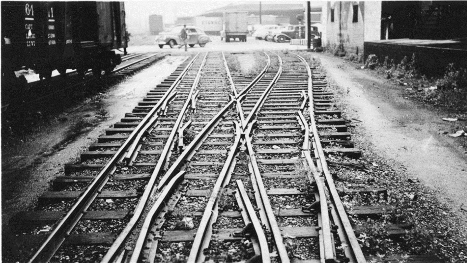
Figure 43. Dual gauge tracks crossing Buffalo Street, with the E.T. & W.N.C. Depot in the background. 157 Also note the Harr building on the right.
