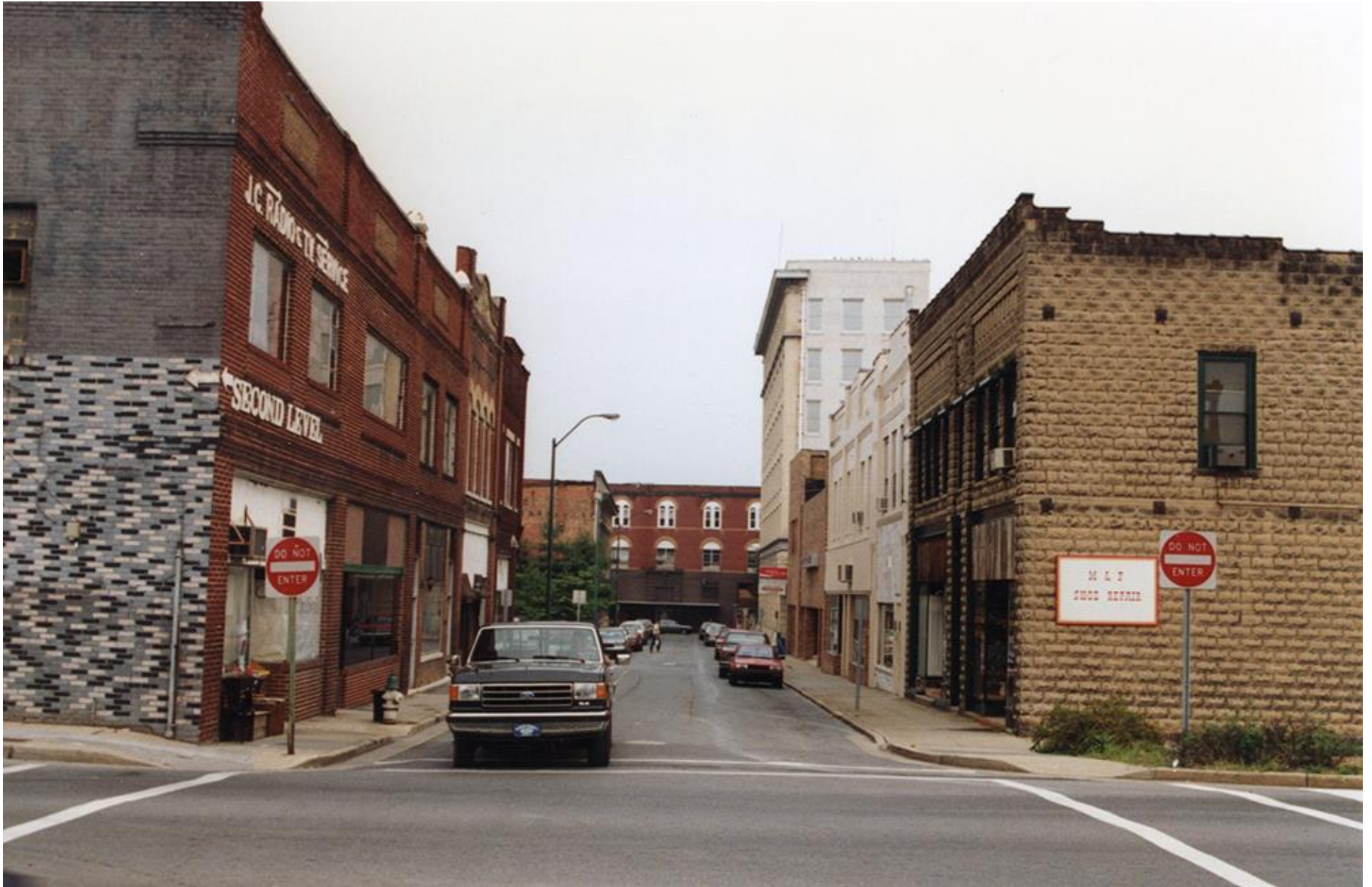
Figure 76. “Spring Street: J.C. Radio & T.V. Service [on the left] and M.I.T. Shoe Repair,” on the right in 1993. 189 The building occupied by the J.S. Radio & T.V. Service was reportedly built in 1925 and later was apparently occupied by the Ferguson Transfer Company.
