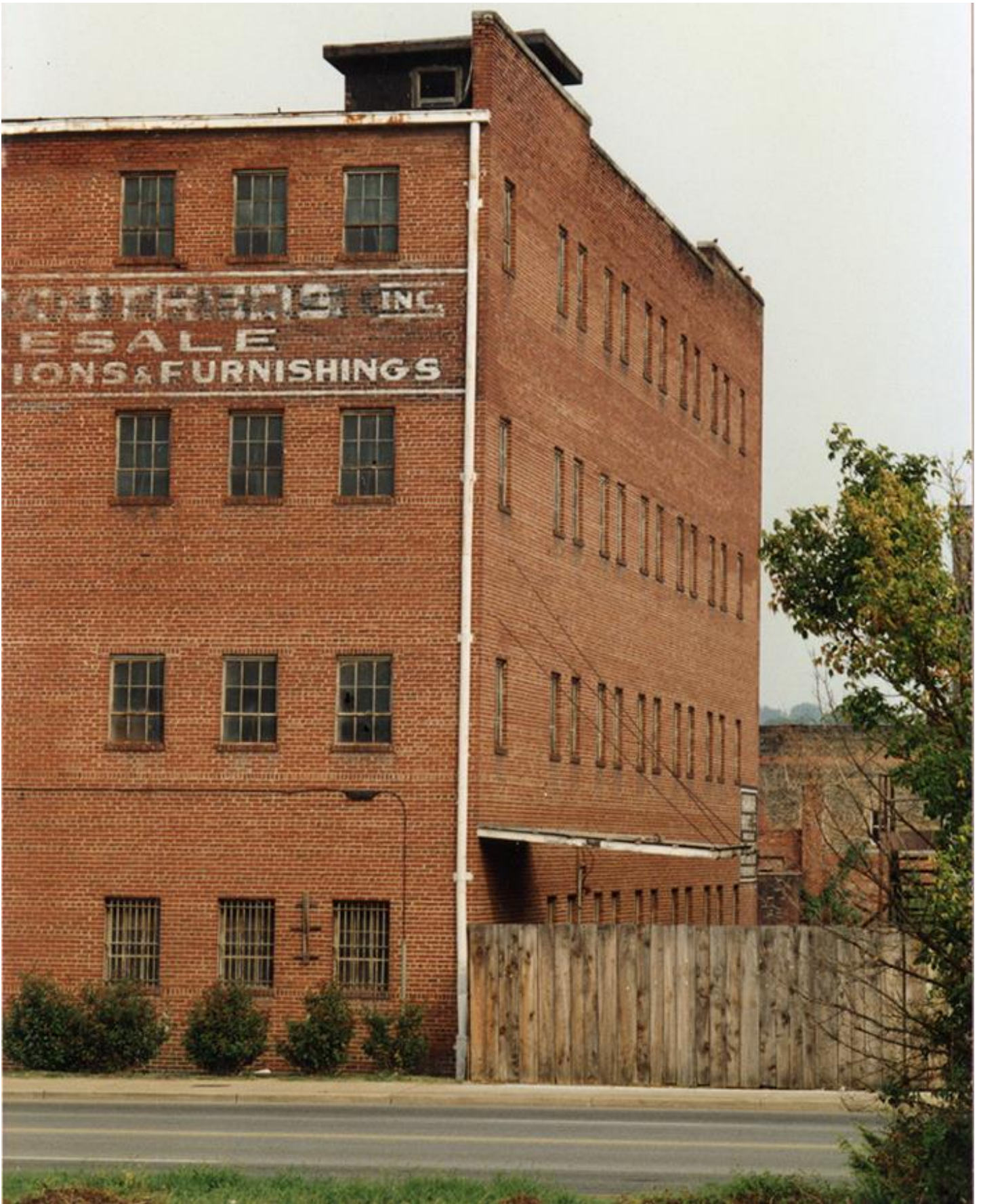
Figure 70. A 1993 photograph of the south and east sides of the Hannah – Dosser/Hannah Brothers building. 182
