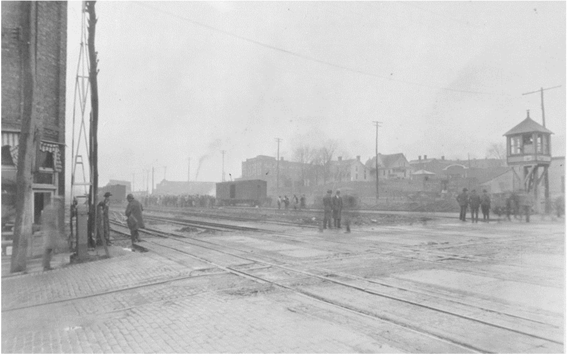
Figure 34. The intersection of Buffalo Street and the tracks of the E.T. & W.N.C. and Clinchfield railroads. The safety tower, built by the Clinchfield in 1910, is visible at the right and one of the gates is visible on the left. This safety tower remained until at least February 1920. Note the trolley tracks running along Buffalo Street, which were removed in 1931. This photograph appears to date to c. 1931. 144
