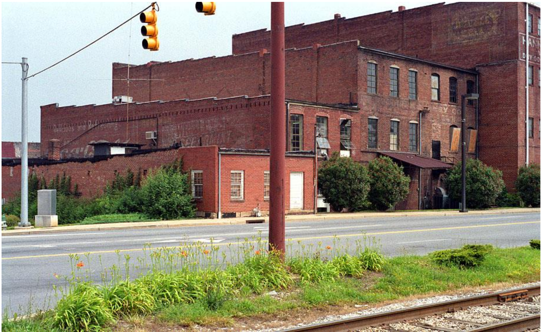
Figure 58. June 1989 – Downtown Johnson City, Tennessee. “The buildings behind the pole can be seen in many old photos of the steam engines working downtown Johnson City. Look in Mal Ferrel’s ‘Tweetsie Country’ for a few of them. The old ET station, now the Free Service Tire Company, is to the left of these buildings across Buffalo Street. ET&WNC and Clinchfield tracks, many of them dual gauge, once ran where I’m standing and where State of Franklin Street is now, right up to the back of those buildings.” 168 The one-story building was the “American Meat Stall,” the two-story building was the Taylor Feed Company, the three-story building was McCown – Mahoney building, and the one on the right was the four-story Hannah – Dosser/Hannah Brothers building. Note the faded Double Cola sign on the west side of the Hannah Brothers building.
