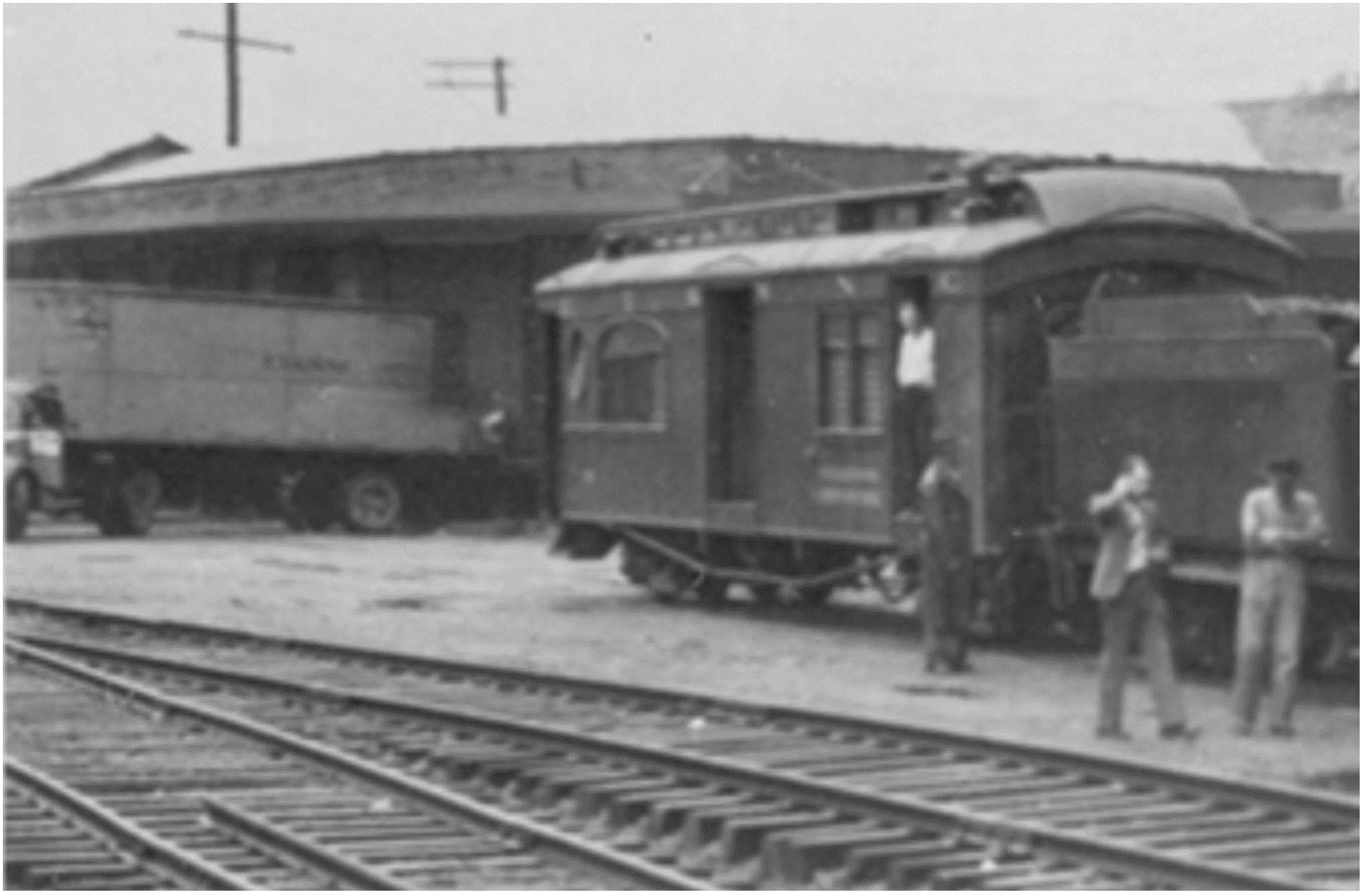
Figure 11A. A detail of the freight section of the E.T. & W.N.C. depot with an E.T. & W.N.C. tractor-trailer on the left.
