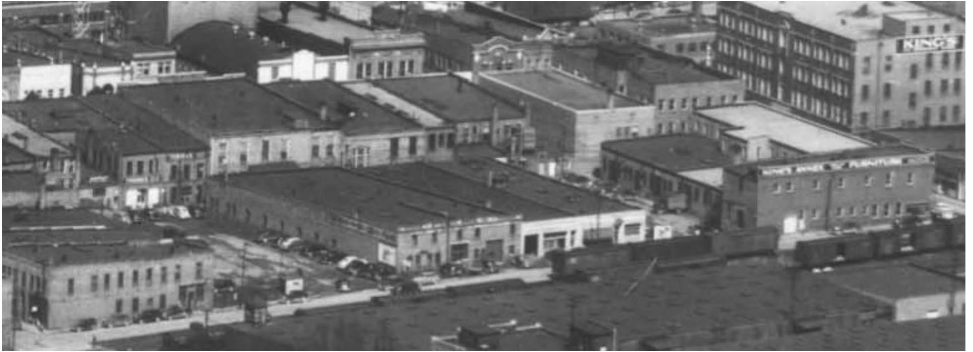
Figure 74B. A detail of the Seaver building and the Sterchi Furniture Company warehouse, from left to right along Jobe Street. Also note the building formerly occupied by the Sells – Brading Lumber Company and the King Department Store building on the right. The author has not been able to identify the building to the right (east) of the Sterchi Furniture Company warehouse. This photograph was taken on 1 March 1947.
