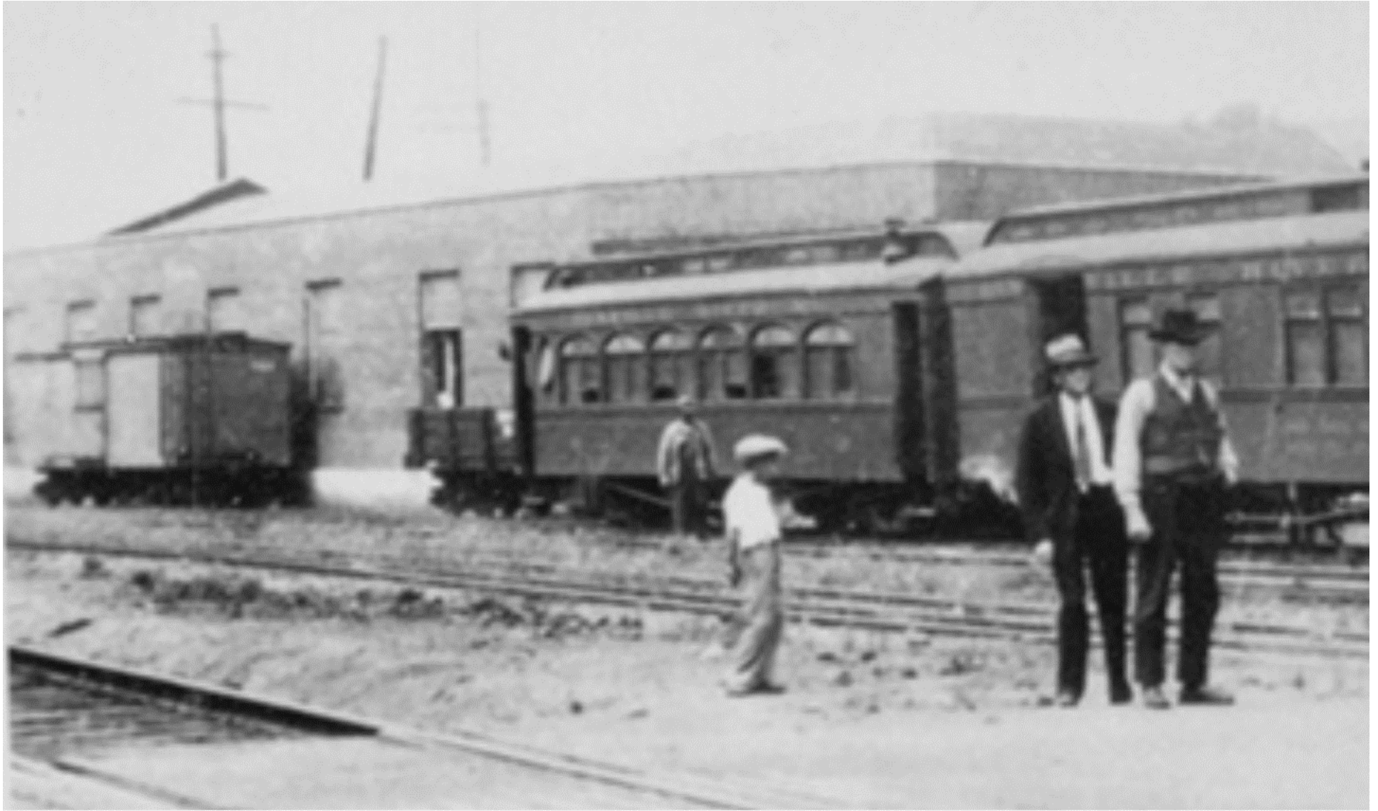
Figure 9A. A detail of the freight section of the E.T. & W.N.C. depot. Historian Johnny Graybeal noted: “In November [1927], a basement was excavated under the freight area 18’ x 24’ x 7’, and a hot water and heating system installed. By this time, the Transportation Company was also expanding into the trucking business. The freight portion of the depot was enlarged in December 1927 by the construction of a large brick addition and turned into a shipping point for trucks. A gasoline storage tank was installed to provide fuel for truck and buses, and the concrete paving was expanded even further.” 36
