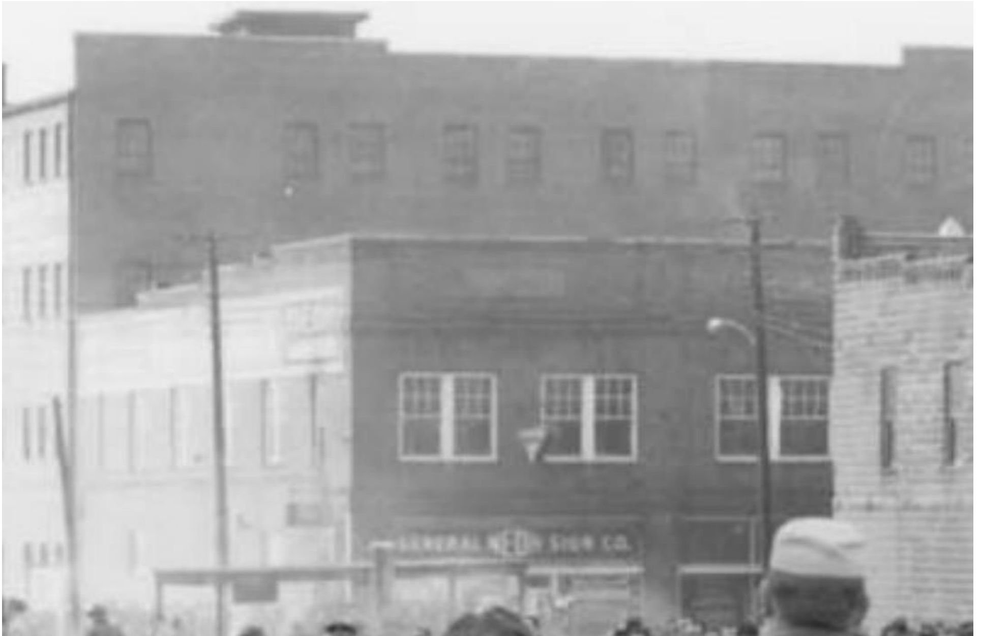
Figure 82B. A detail of the front (east side) of the Ferguson Transfer Company building, with a sign reading “General Neon Sign Co.”
