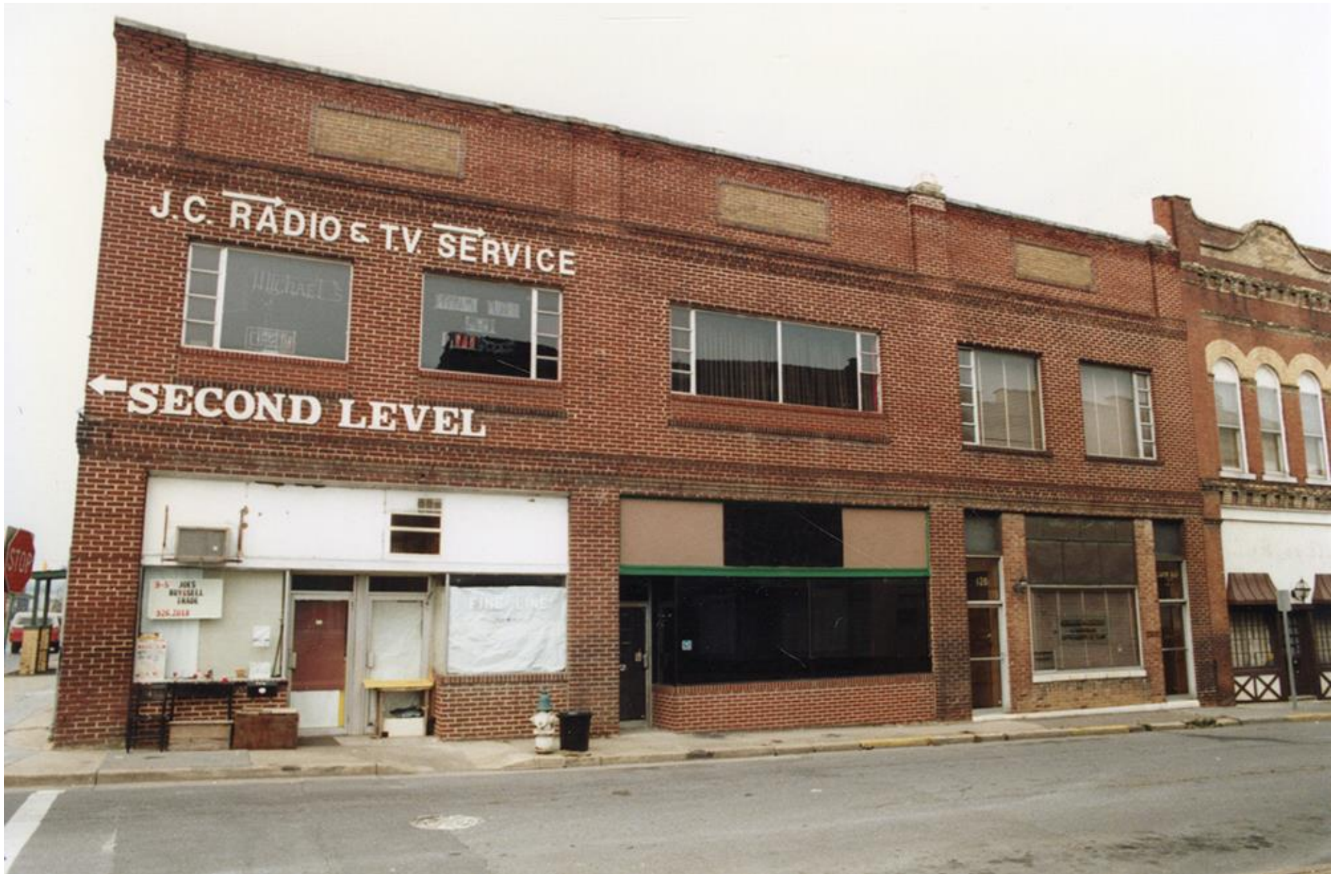
Figure 77. “Spring Street: J. C. Radio & T. V. Service”, front (east) side, looking west from Spring Street in 1993. 190 This building was reportedly built in 1925 and was occupied by the Ferguson Transfer Company.
