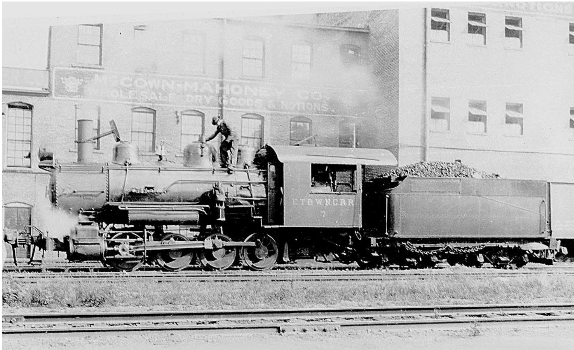
Figure 66. This “is the 7 after Cap Allison gave her a new frame, wheels, and changed the tender to hold more water. This 1930s photo was taken down between Spring Street and Buffalo Streets Johnson City.” 177 Historian Johnny Graybeal captioned this photograph: “Switcher 7 works the interchange with the Southern Railroad on July 20, 1931. By this time the only regular engine jobs on the ET&WNC were the Mixed train from Boone and the Switcher...” 178
