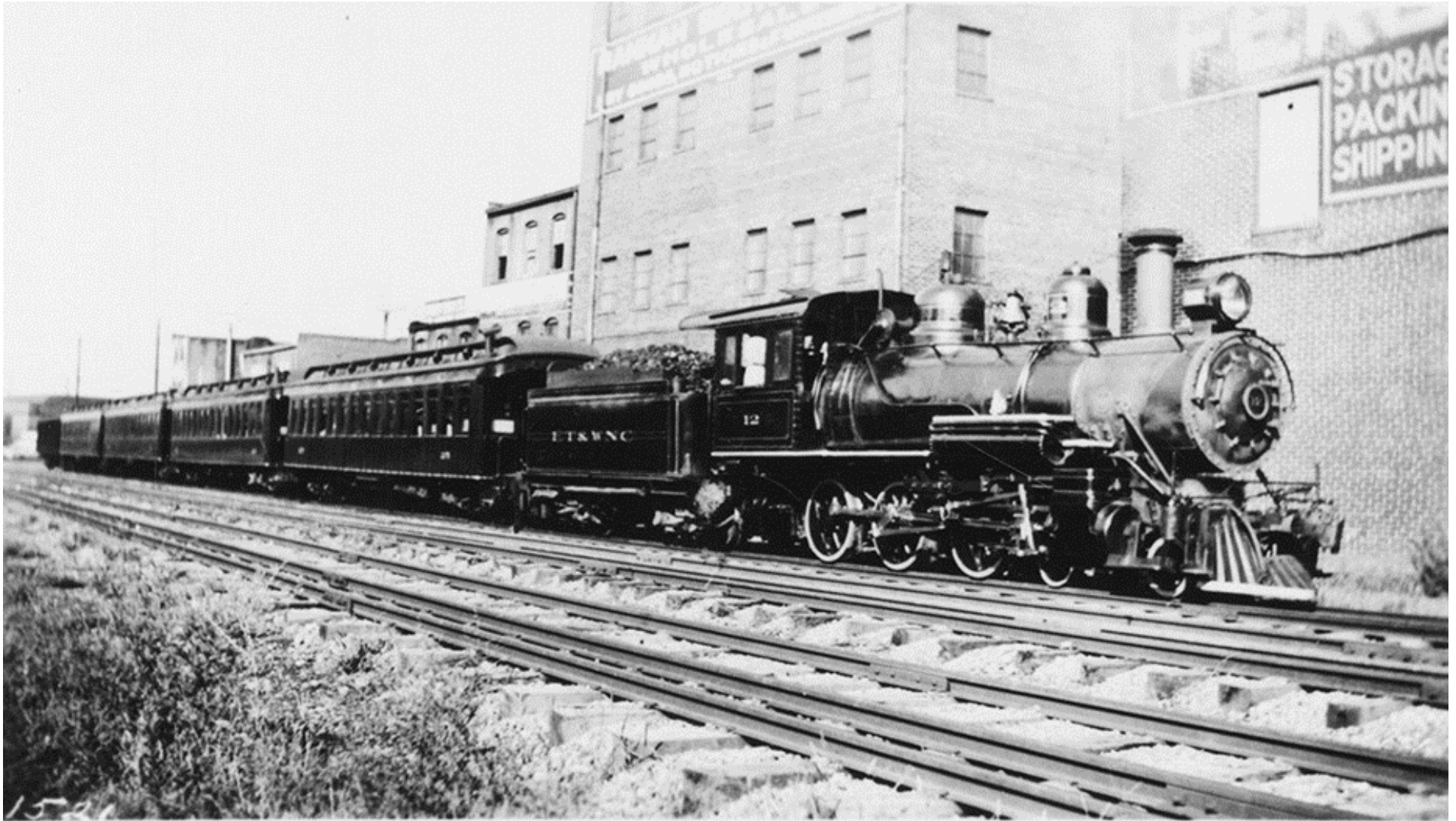
Figure 71. Historian Johnny Graybeal wrote of an apparently related photograph: “original ‘Hobbs’ lettering scheme in 1936, the No. 12 photo dated August 30 th . The striping on the cab has sharp corners and so does the stripes on the tender, except for the stripe on the coal board. Striping also adorns the sand and steam domes, the steam chest, and cylinder casings... L.L. Norton photo via Roy McLain Collection...”, which also showed that the sign on the building on the right read: “Ferguson... Storage, Packing Shipping”, apparently in reference to the Ferguson Transfer Company. 183 Also note the buildings of the McCown – Mahoney Company and the Hannah Brothers Company, from left to right, in the center background of this photograph.
