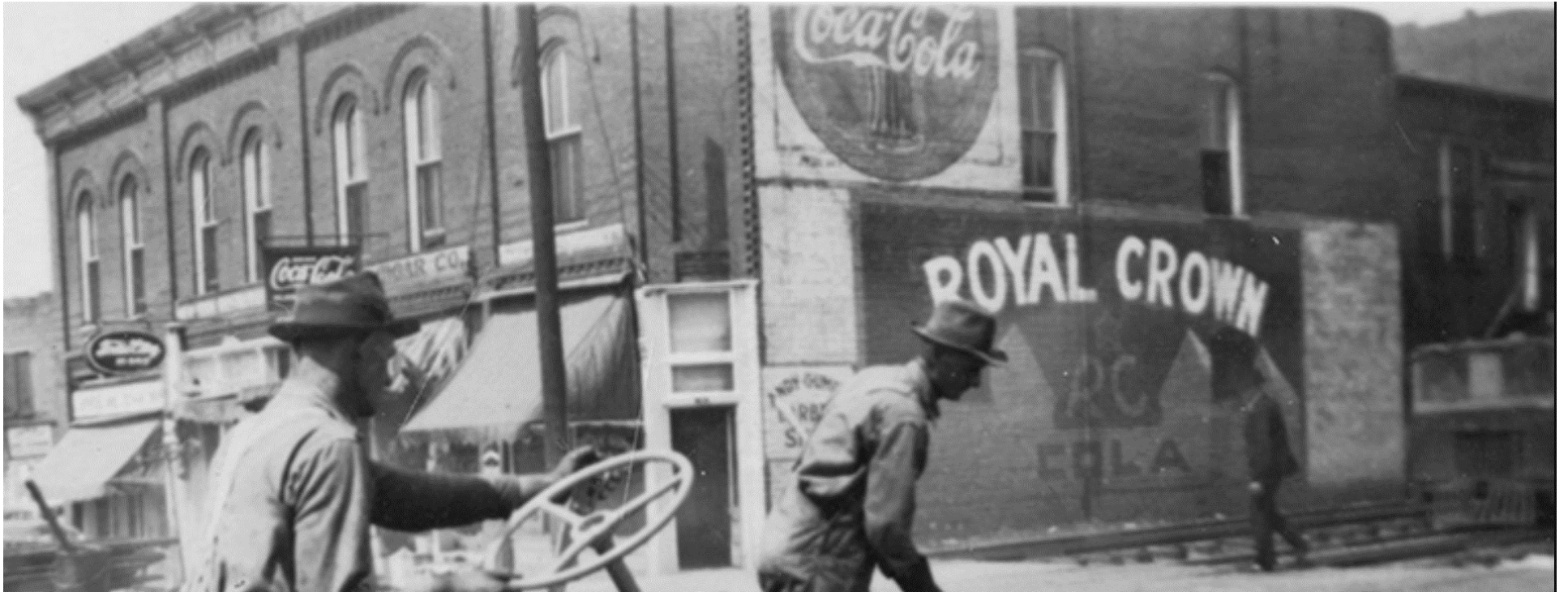
Figure 37A. A detail of the Harr building, note the E.T.&W.N.C. speeder on the right side of this photograph. The sign on the west side of the Harr building, by the Coca-Cola sign, appears to read “Cigar Co.”
