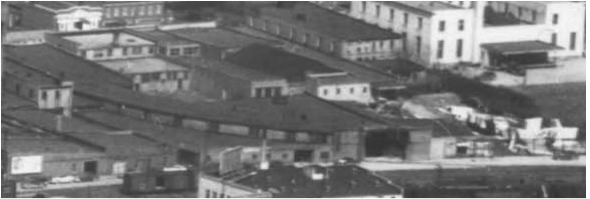
Figure 98A. A detail of the Brading – Marshall/Marshall Brothers building, on 1 March 1947. Note the lumber yard to the east (right).
