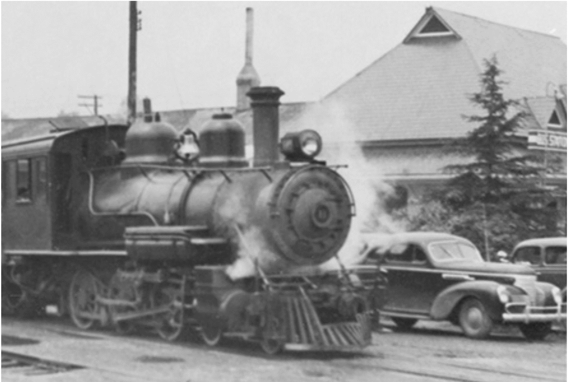
Figure 11B. A partial detail of the south side of the station, which has a sign reading “Bus Station”.
