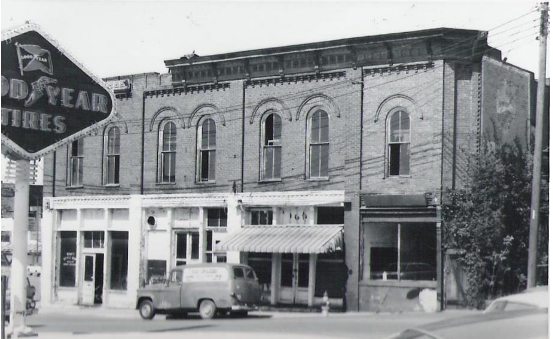
Figure 33. A photograph of the Harr building on looking east across Buffalo Street. This photograph appears to date to 1950s or 1960s. 143 Note what appears to be a Pepsi-Cola sign on the right (south) side of the building and the missing section of the cornice along the top of the building on the left. Also note the slightly lighter brick color of the addition to the building on the right, this section was added between 1908 and 1913.
