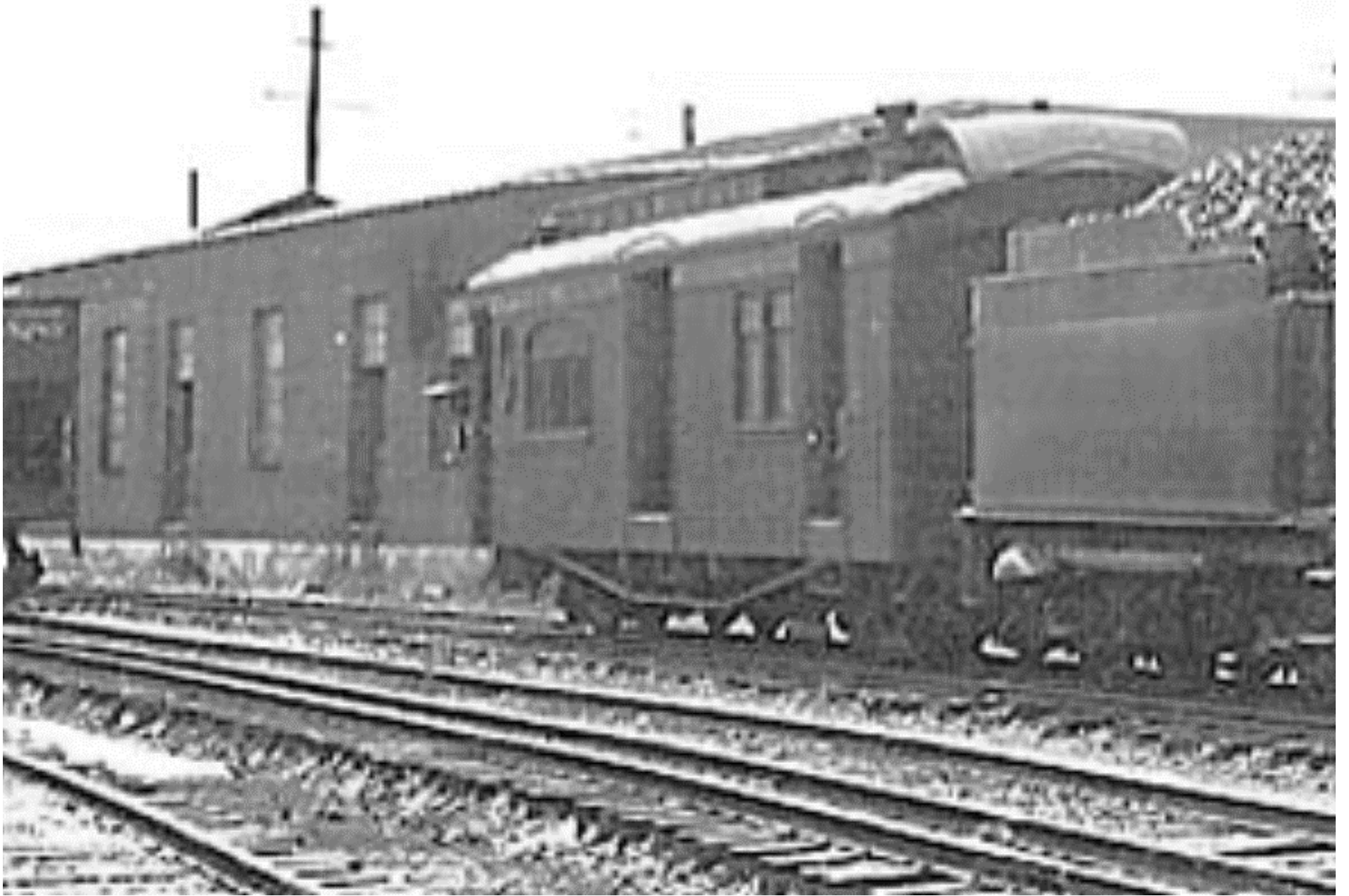
Figure 10A. A detail of the freight section of the E.T. & W.N.C. depot.
