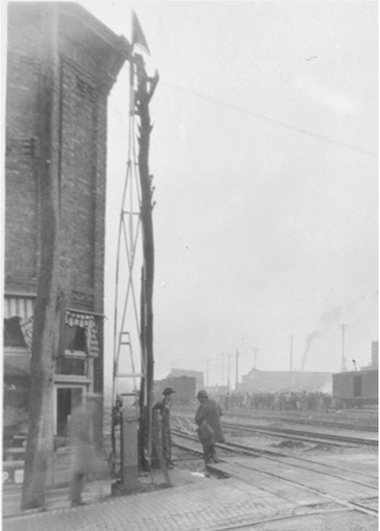
Figure 34A. A detail of the southwest corner of the Harr building.
