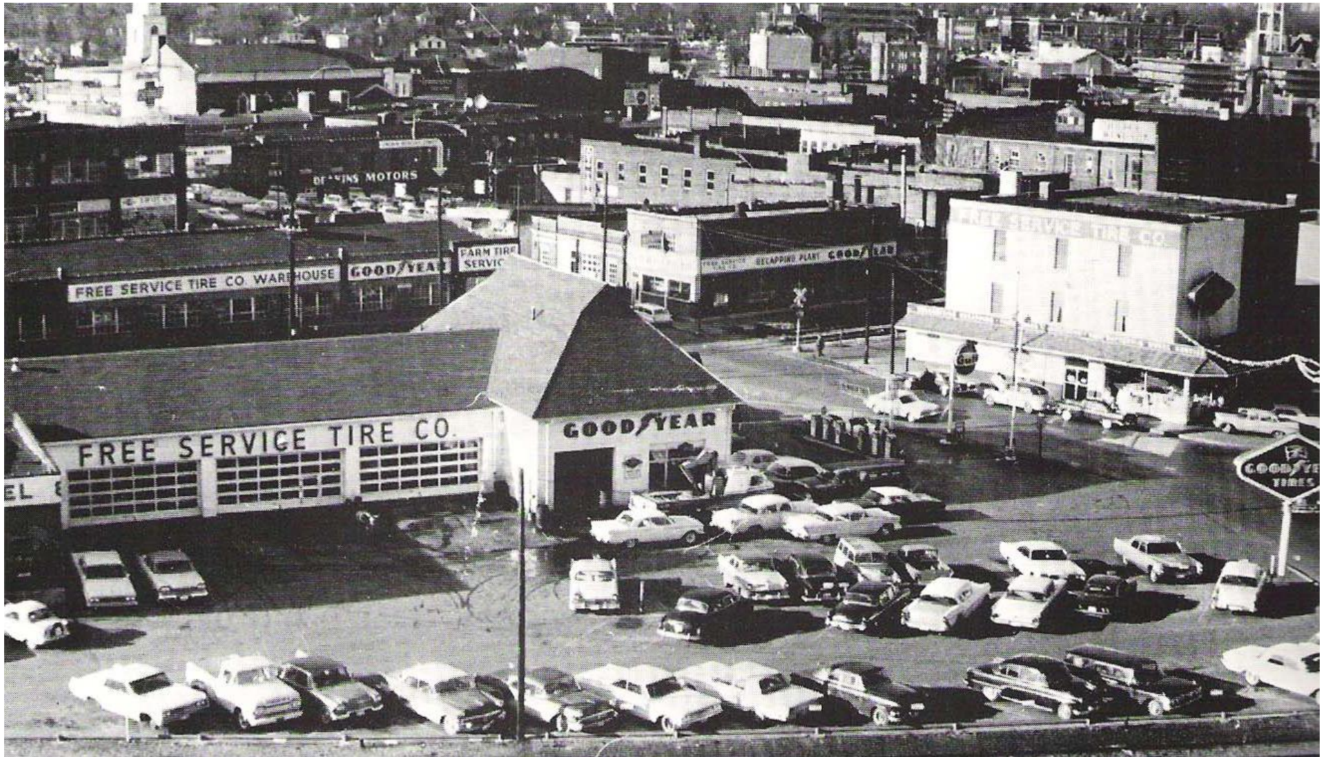
Figure 16. This photograph shows the former E.T. & W.N.C. depot, now occupied by the “Free Service Tire Co.,” apparently in the 1950s or early 1960s. 45
