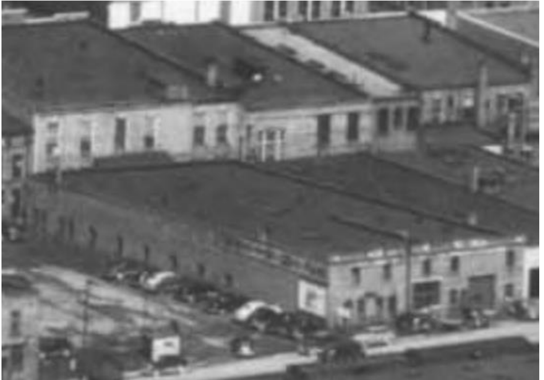
Figure 74C. A detail of the J.D. Sterchi Furniture Company warehouse on 1 March 1947.
