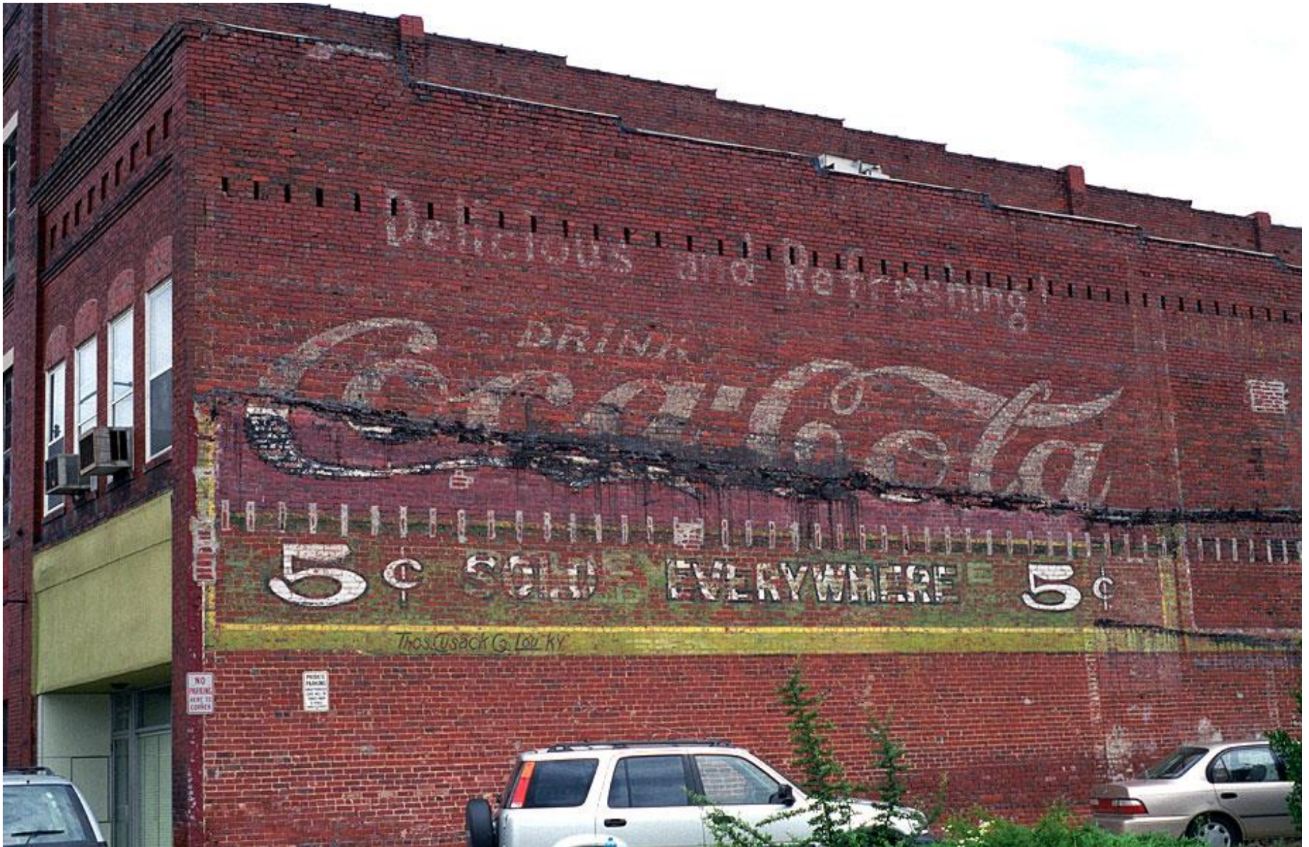
Figure 52. June 1998 – Downtown Johnson City “Tear down an old building [which housed the American Meat Stall for a time] and you never know what you’ll find on the next door wall”, see Figure 51. 162 The building in this photograph was occupied by the Taylor Feed Company from 1918 to 1921 (?).
