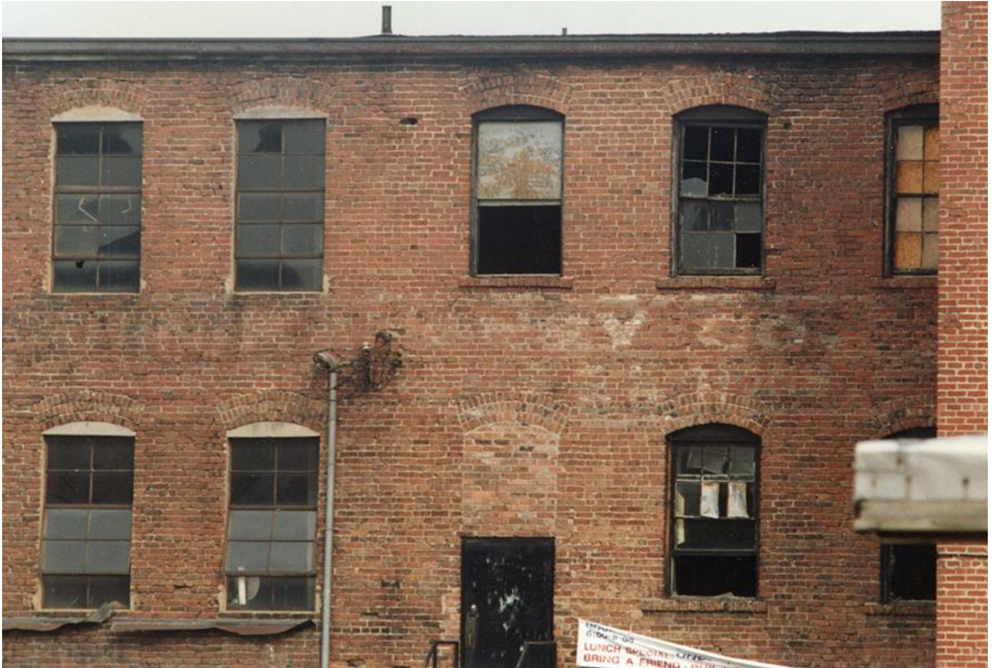
Figure 67. A 1993 photograph of the McCown – Mahoney building. 179
