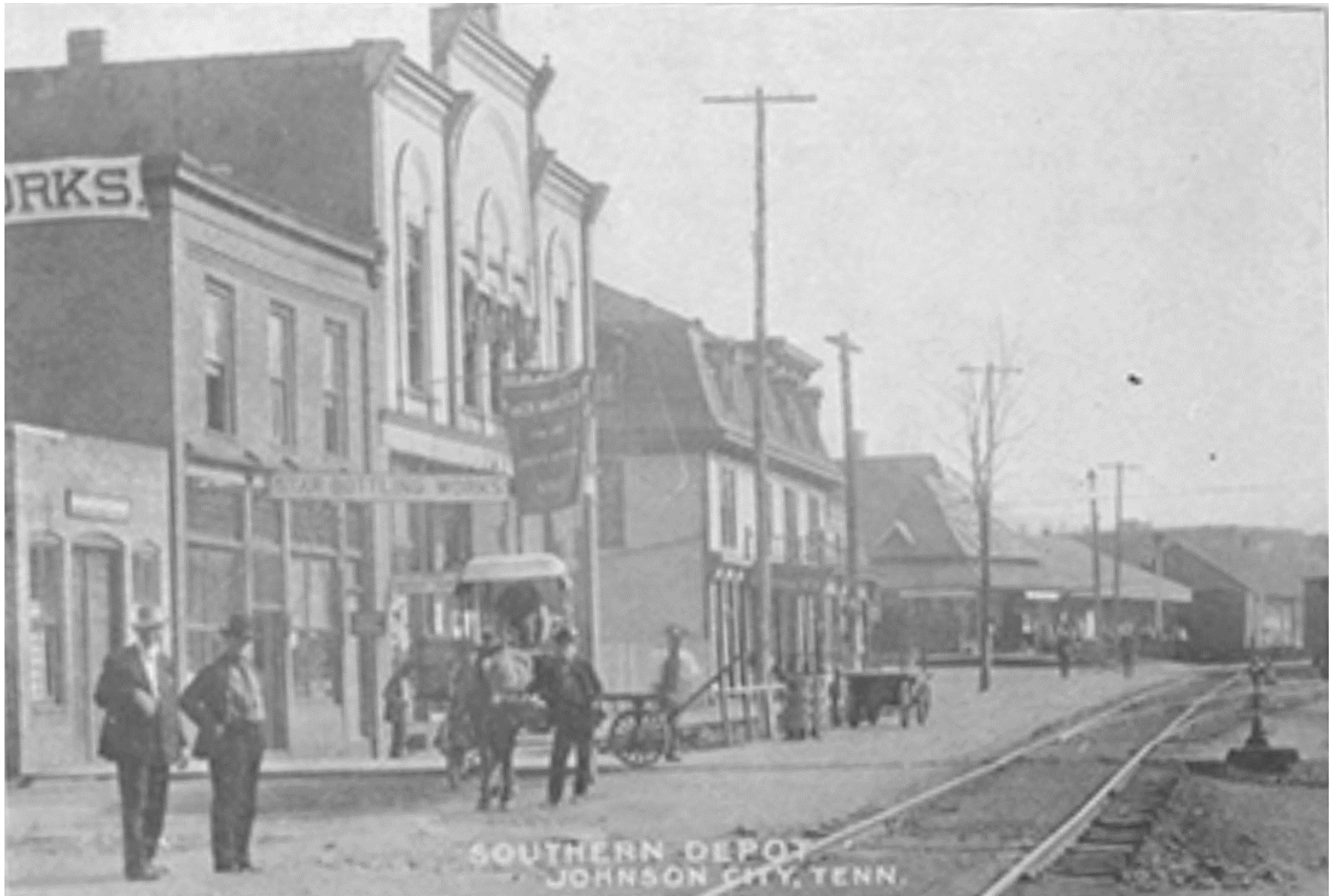
Figure 3. On the right side of this photograph is a portion of the union passenger station and freight depot. Map 15 indicates that the other buildings (from left to right) in this photograph are the 'Southern Express', "Box Ball Alley" (occupied by the "Star Bottling Works" according to the sign), the next building was occupied by a barbershop (on the left) and a pool hall (on the right), a gap of about 35 feet, and then the "Planters Hotel". Out of sight beyond the hotel are another pool hall and a boarding house. Of note, the "Star Bottling Works" only operated from 1908 to 1909. 26
