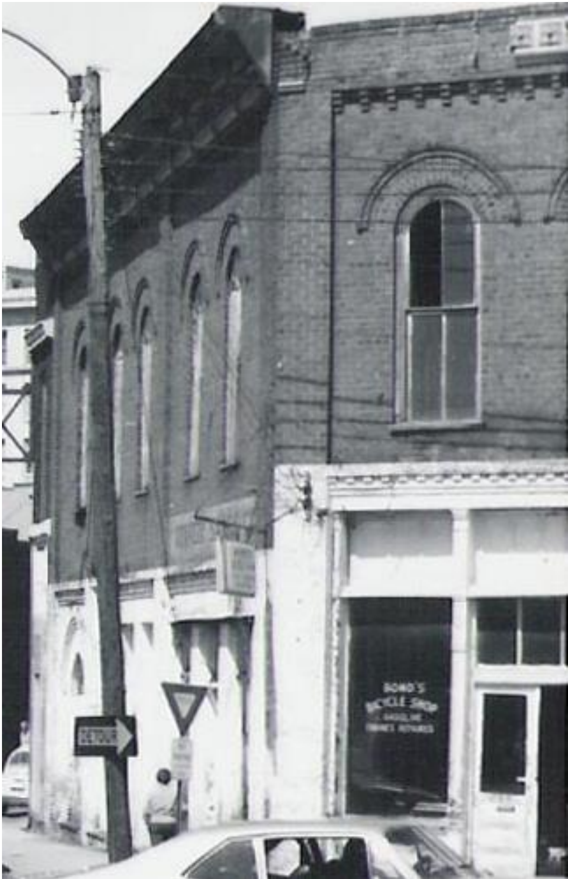
Figure 28A. A detail of the Harr building of the rarely photographed northwest side.
