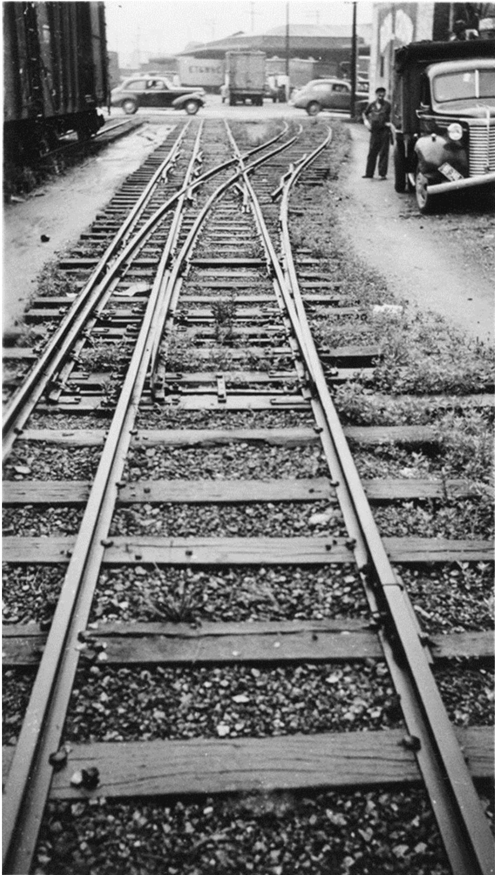
Figure 44. "Double gauge turnout at Johnson City, July 1940." Note the Royal Crown sign on the Harr building. 158
