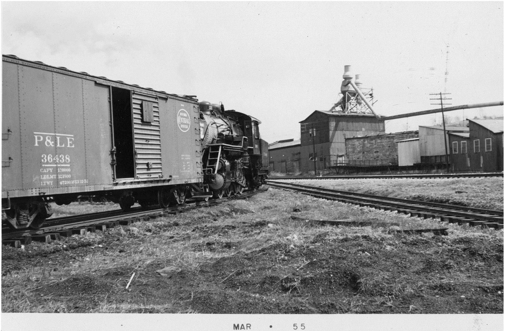
Figure 52. This photograph, dated March 1955, shows the Harris Manufacturing Company in the right half of this image. Note that the two-story “Main Mill” building has been removed or significantly remodeled, see figures 47, 48 and 49. 159
