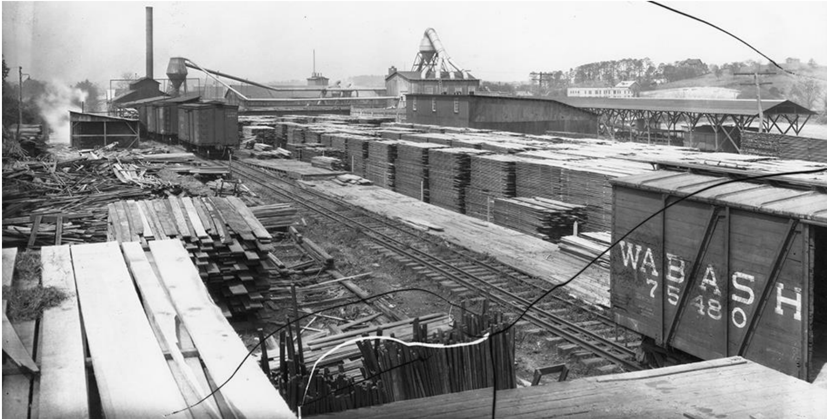
Figure 58. This photograph of the Harris Manufacturing Company appears to have been taken from near the junction of Afton and East Walnut streets, looking northwest. 165 The dual-gauge trackage in this photograph was a spur that ran west from the Clinchfield mainline into the Harris plant along East Walnut Street. Note configuration of the cyclone on the building near the center of this image. This indicates that this photograph predates those in figures 56 and 57. Also note the “Dust Conveyer” that connects the 2-story building to the building with the smokestack, which appears to have been the concrete block building that housed the “Dutch ovens,” see Map 17B. The building with three windows, in front of the two-story building with the cyclone appears to be the “Saw Mill,” with its covered “tram way” extending to the right. The low building between the two-story building with the cyclone and the “Saw Mill” appears to be the dry kilns (if correct, this building has been extended to the south). The building between the two-story building with the cyclone and the building with the smokestack appears to be the building composed of “Ware Hos” No. 2 and No. 3, if correct, this building has also been enlarged to the south. It also appears that “Mouldings & Lumber War Ho. No. 4” and “Ware Ho. No. 1,” as well as the houses on the south side of East Walnut Street, which appear on Map 17, have been removed by the time this photograph was taken. Finally, note the Franklin Apartments in the right background, as well as what appears to be the top of the Sevier Hotel (built in 1924), behind the “Main Mill” building. The cyclone on the roof of the “main mill” indicates that this photograph was taken prior to 13 October 1937, see Figure 56. Consequently, it appears that this photograph dates to between 1924 and 1937.
