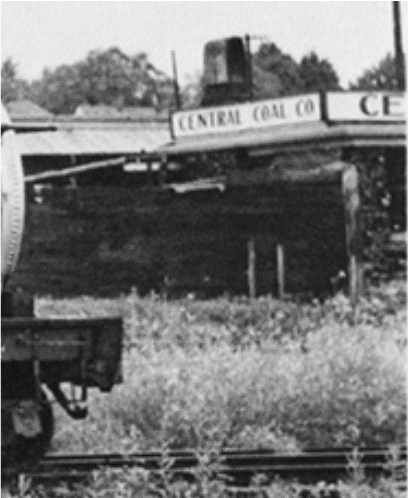
Figure 32A. A detail of the Central Coal Company, located adjacent to the plant formerly operated by the American Cigar Box Lumber Company.
