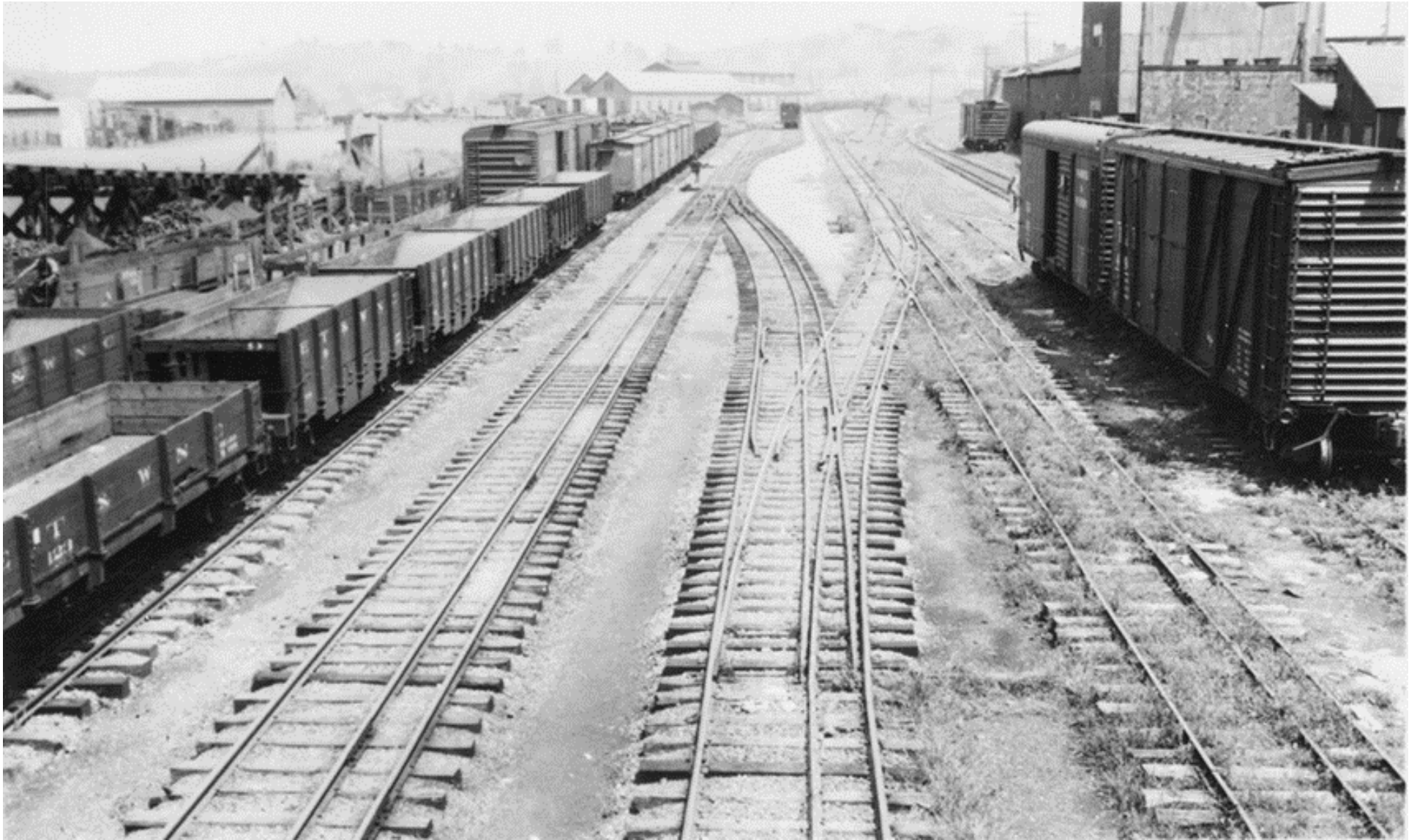
Figure 50. This photograph looks east toward the E.T. & W.N.C. shops (in the center background), with the Harris Manufacturing Company in the right background and the E.T.&W.N.C. coal transfer trestle on the left. 157 Note the presence of dual-gauge trackage, the third rail of which was removed in 1946, and the truck repair shop, which was completed in 1937.
