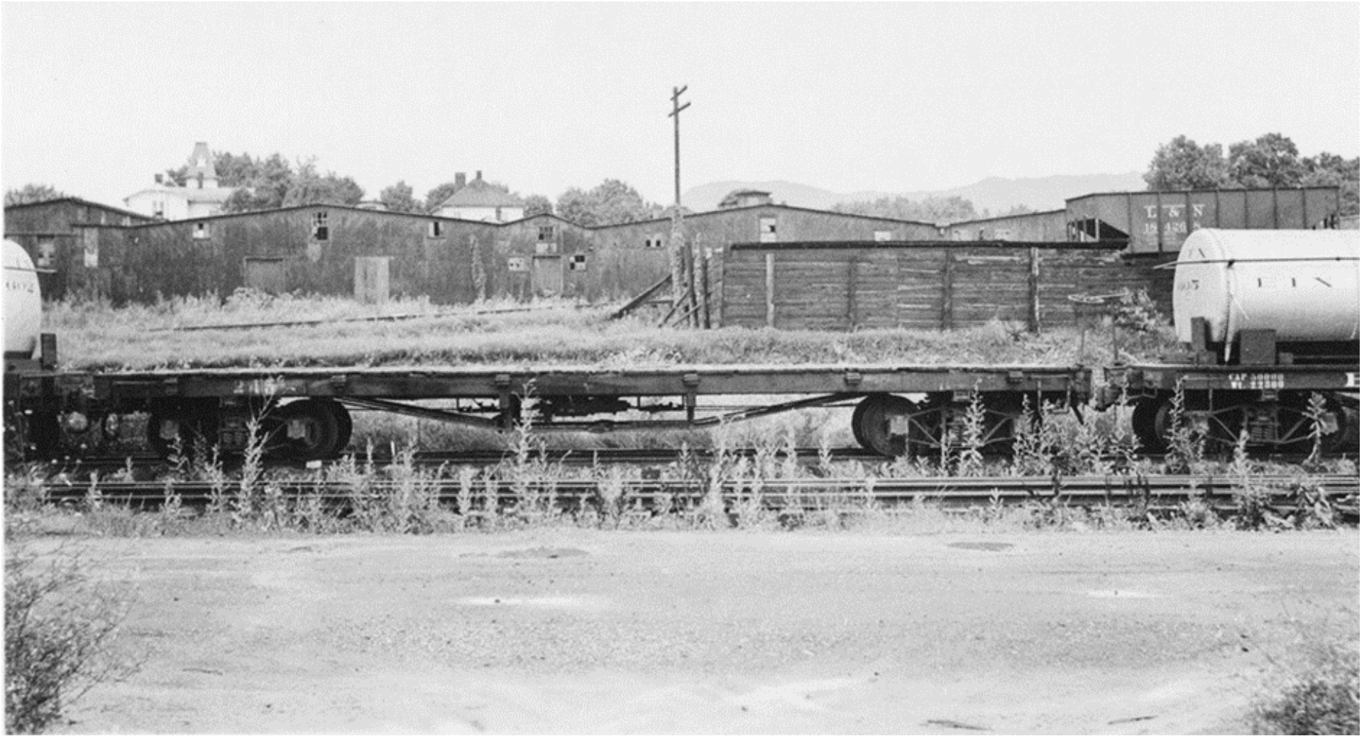
Figure 33. American Cigar Box Lumber plant in the background. Note the wooden enclosure and the L&N hopper car (#184268) behind it, on East Cherry Street in the right background. The wooden enclosure probably serves as a coal bin for the Central Coal Company. It appears that this photograph was taken in July 1940. The flat car is #245 and the tank Cars are #602 (left) and #605 (right).” 93 From left to right, the buildings depicted in this image appear to be the corrugated iron “Ware Ho.”s “C” and “B” depicted on Map 9B, see also Figure 34B. Based on Map 9B, it appears that these buildings had been modified after 1920.
