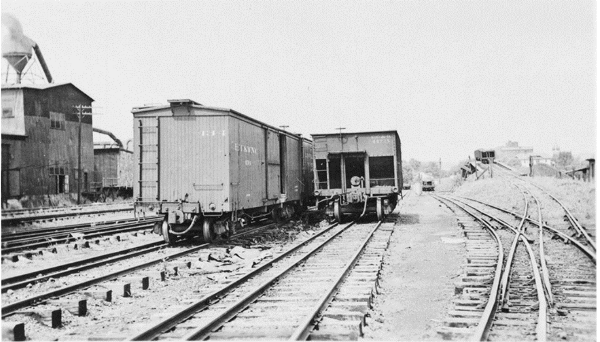
Figure 53. "Comparison Shot. Narrow gauge box car [E.T. & W.N.C. #434] same height as standard gauge hopper. Narrow gauge hopper on trestle. Taken at Johnson City, Tenn. Two tracks next to the lumber mill (left) Clinchfield R.R. July 1940." This photograph looks west toward downtown Johnson City. The Harris Manufacturing Company is on the left and the E.T.&W.N.C. transfer trestle on the right. 160 Note the presence of dual-gauge trackage.
