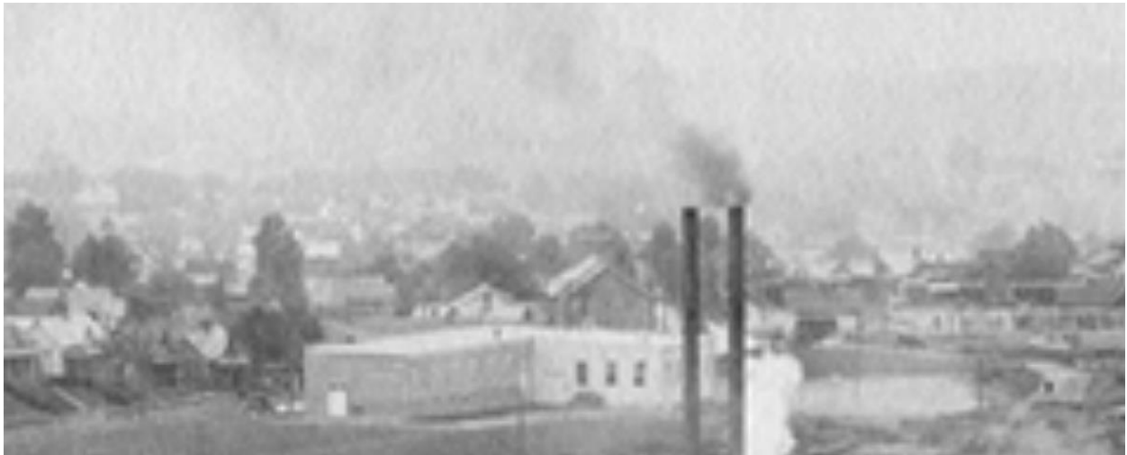
Figure 67B. Another detail of what appears to be the building occupied by the “H.M. Yost Shuttle Block Factory”/“Dealers Supply Co. Inc. Plant”/S.E. Guinn Manufacturing Company, this time looking southwest. It appears that this photograph was taken in 1924.
