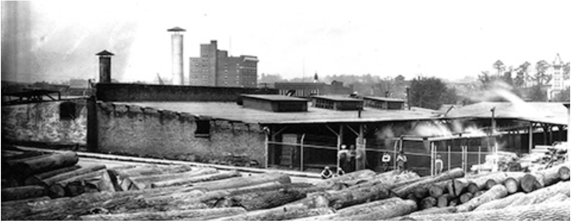
Figure 36A. A detail of the Cutting and Shaping Mill, see Map 9C and Figure 25B. Note that the more lightly covered portion of the building on the left of this image appears to have been added after 1920.
