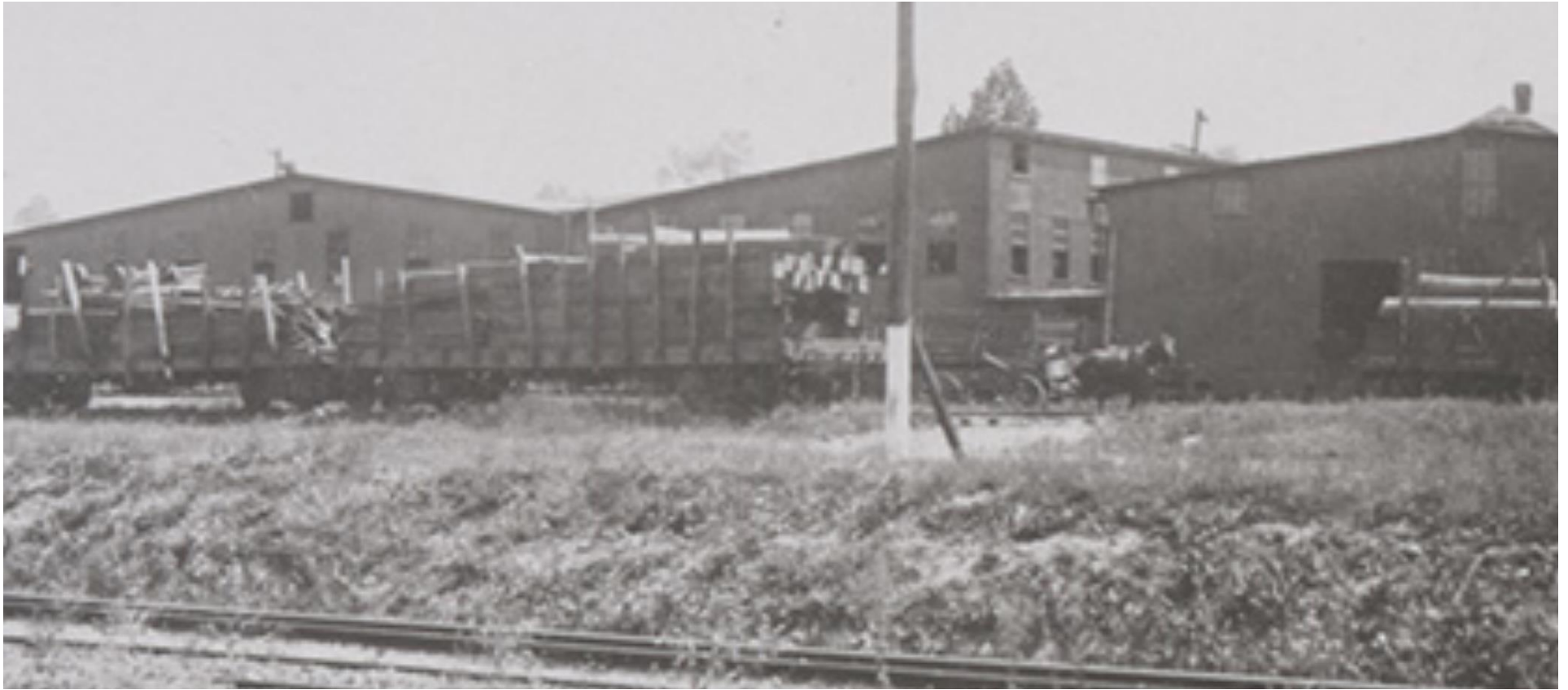
Figure 34B. Another detail, this appears to depict buildings “E,” “D,” “C,” and “B” (from left to right), all of which were “iron clad.” Note that “D” and “E” appear to actually comprise a single building, and that “B,” “C” and “D” were used as warehouses. Also note the horse and wagon between buildings “B” and “C”.
