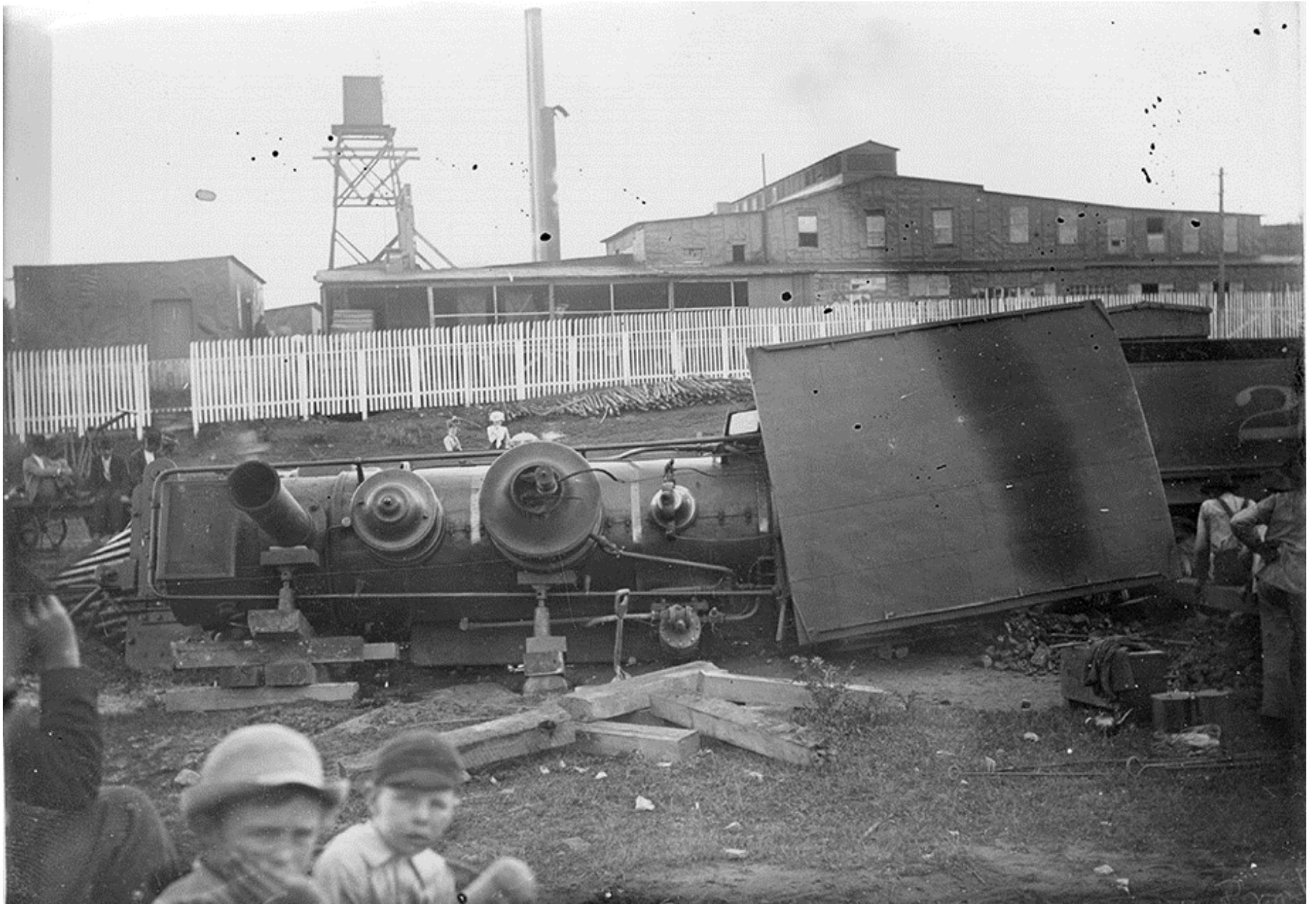
Figure 21. Another view of the wreck of Engine No.2 and the American Cigar Box Lumber Company mill. 60 Note the hand car in the left background.
