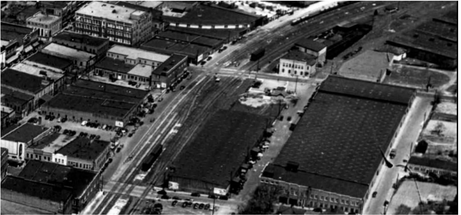
Figure 8B. A detail, with what appear to be some of the buildings previously occupied by the American Cigar Box Lumber Company in the top left corner of this image, taken 19 April 1941.
