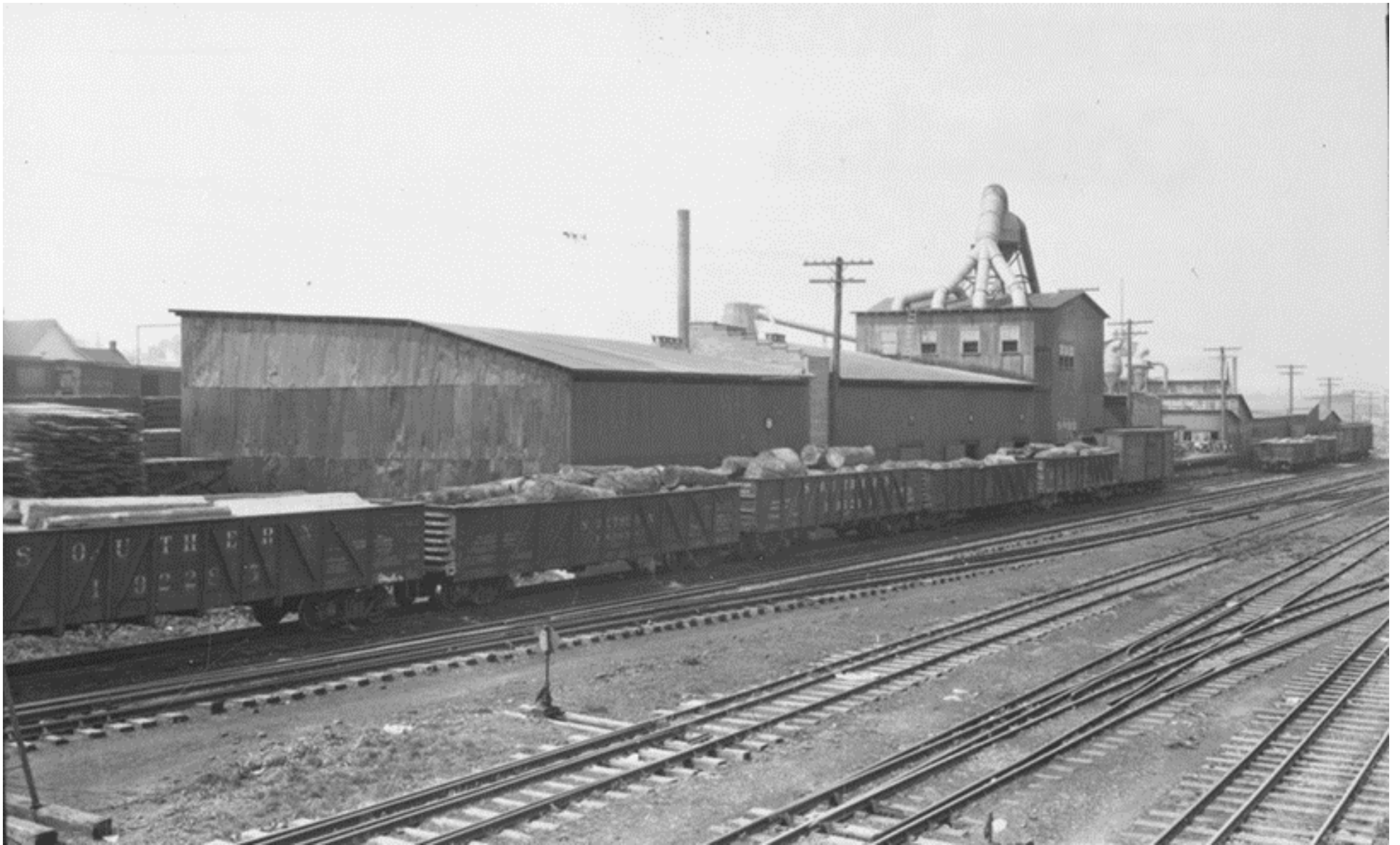
Figure 54. Harris Manufacturing Company, looking west. Note the boxcars in the left background, which would have been on the dual-gauged East Walnut Street spur. The configuration of the cyclone on the roof of the building in the right half of this image indicates that this photograph was taken prior to 13 October 1937, see Figure 56. 161
