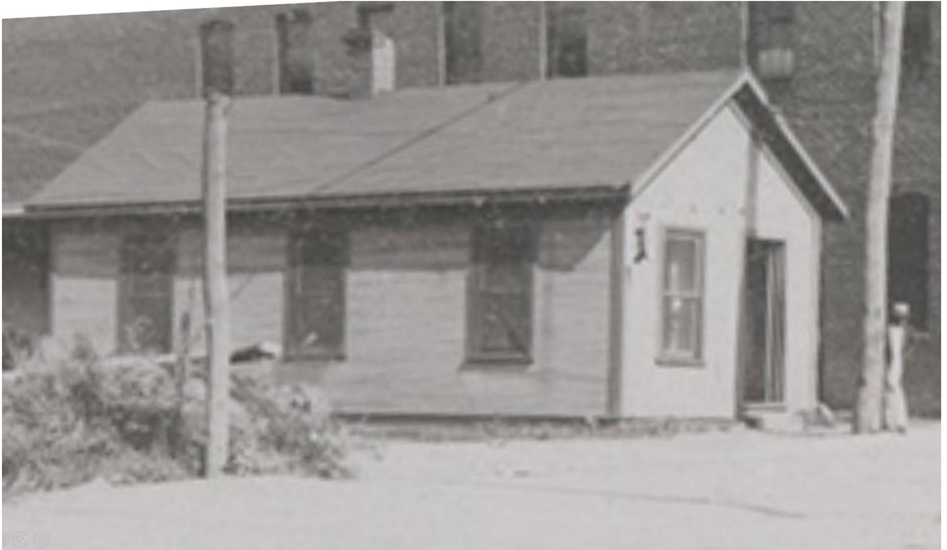
Figure 3A. This detail appears to show the building that was the office of the C.L. Bolton company, on the northeast corner of South Roan and Cherry streets. This photograph was taken during the period in which the “Johnson City Coal, Ice and Cream Company” occupied this property and appears to date to between 1920 and 1923, see Figure 3. 10 This building measured about 33’ x 14’.
