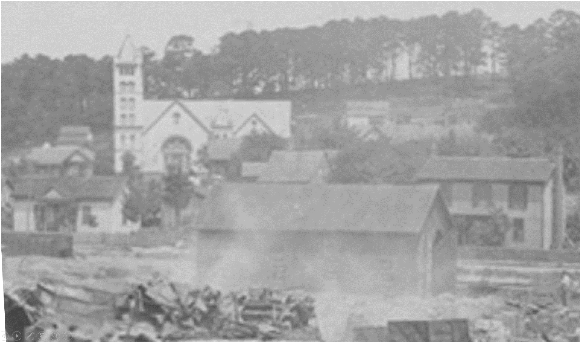
Figure 25A. A detail of the E.T. & W.N.C. “Locomotive Ho.” near the William E. Uptegrove & Brother Vener Mill,” apparently after the fire of 12 July 1906. Note what appear to be three or four windows on the south side of the locomotive house. The addresses of the two residences behind the “Locomotive Ho.” along the north side of E.T. & W.N.C. mainline appear to be at 1409/119 and 1411/123 Jobe Street, see map 2 and 3.
