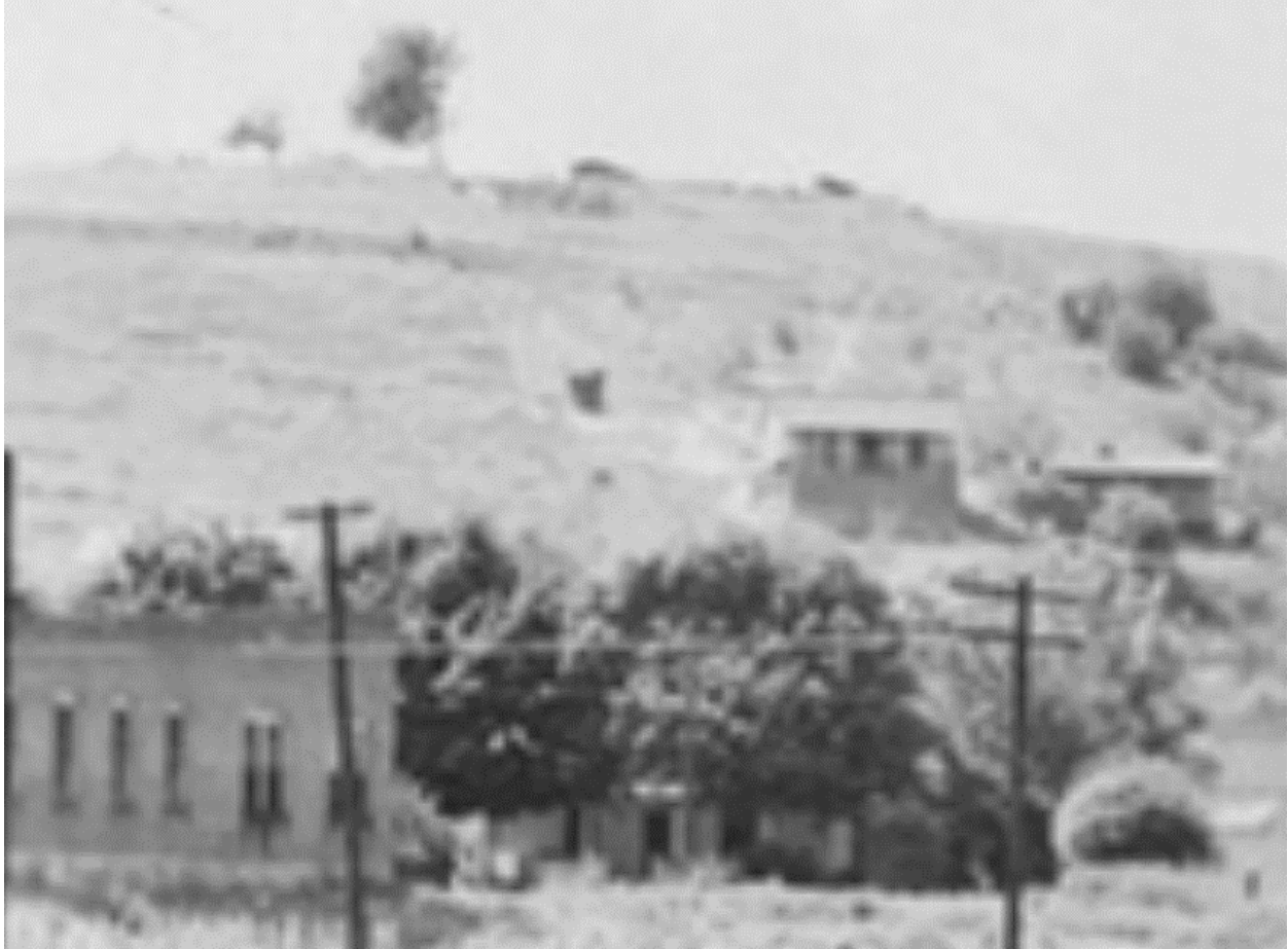
Figure 65A. A detail of what appears to be the west side of the building occupied by the “H.M. Yost Shuttle Block Factory”/“Dealers Supply Co. Inc. Plant”/S.E. Guinn Manufacturing Company, on the left.
