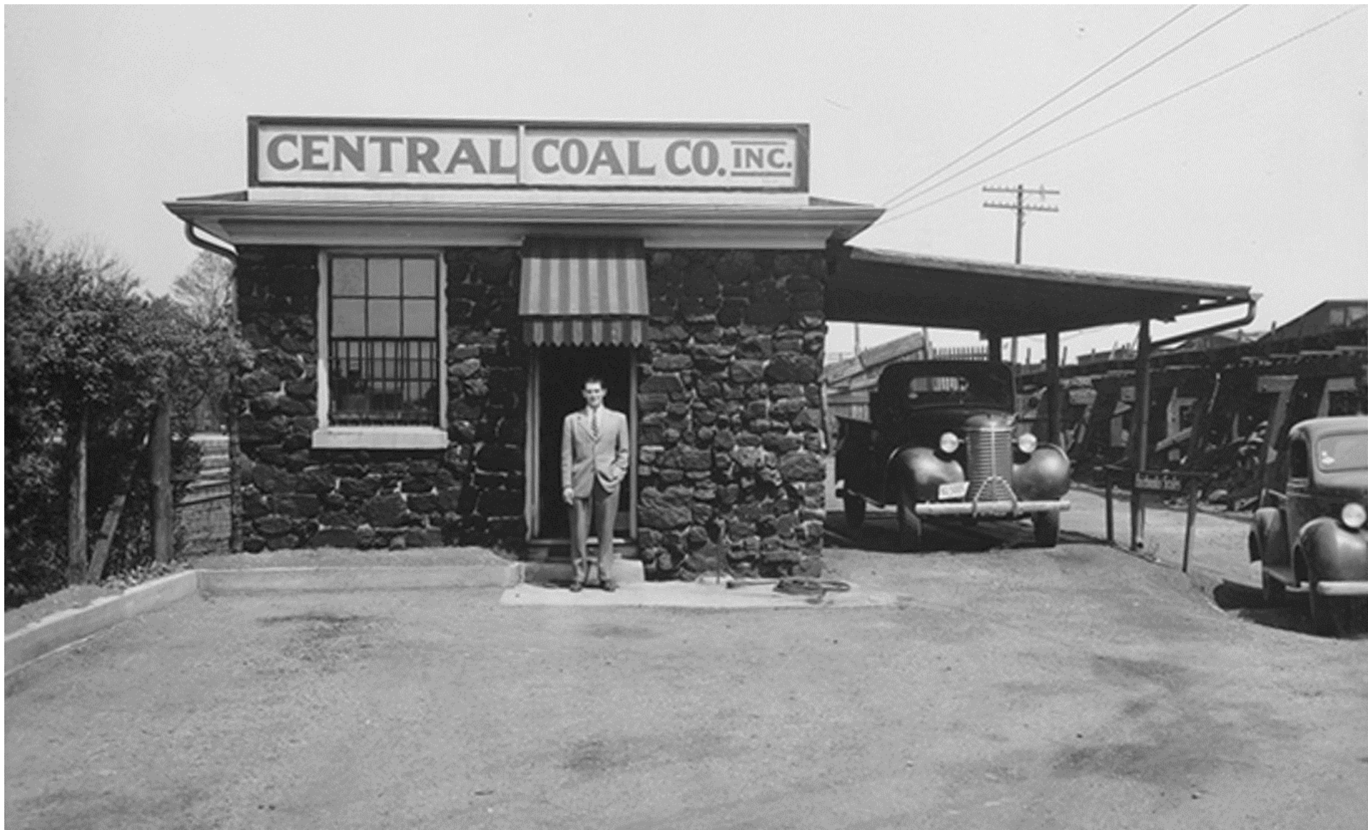
Figure 10. “Central Coal, Oil and Equipment Company”. “This office building was built from blocks of coal for $1,000 in 1931. The building, 20 x 30 feet, had three rooms and a bath. Several inches of concrete between the coal and the plaster made the building fireproof. Needless to say, the proprietor, Mr. Jim Morris, Jr. (standing in the doorway), sold coal. His competitors often chided him, saying that his coal wouldn’t burn because he made an office from it. The building was razed in 1979 for a public parking lot. Photo courtesy of Jim Morris, Jr.” 46 This photograph looks west, note the railroad tracks visible through the bushes on the left and the roofs of the American Cigar Box Lumber Company on the right.
