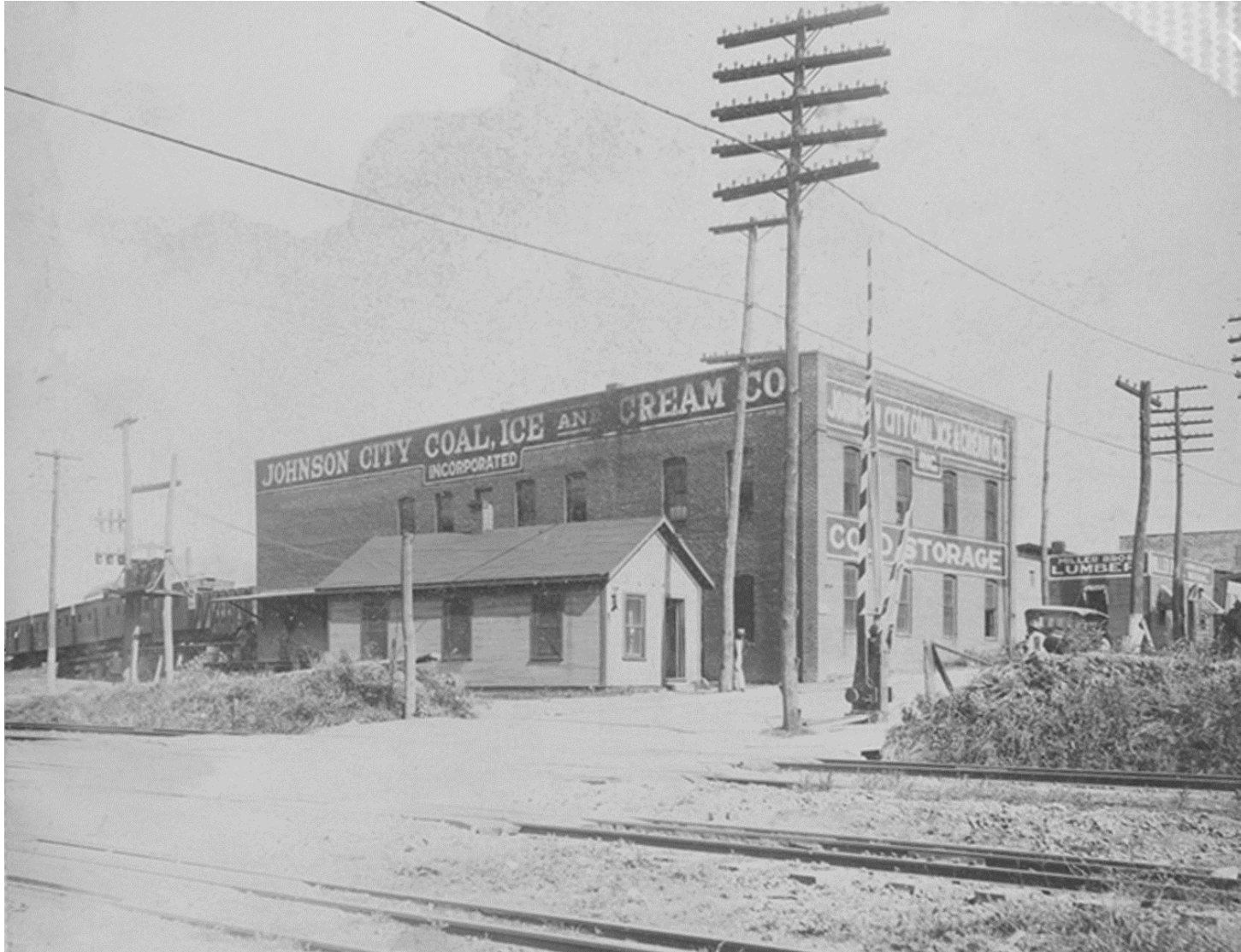
Figure 3. “Johnson City Coal, Ice and Cream Company”. The large brick structure was originally built for the “Clinchfield Ice & Coal” in 1914, on the northeast corner of South Roan and East Cherry streets. 17 It was acquired by the “Johnson City Coal, Ice and Cream Company” in 1916 and was used by this company until about 1923. Note the Miller Brothers Lumber Yard office in the right background. Also note the coal trestle on the left and the dual gauge track in the foreground, as well as the railroad crossing guard. The transformer set in front of the coal trestle did not appear on the Sanborn Insurance Company map of 1920, perhaps indicating that this photograph dates to between 1920 and 1923. Perhaps also of interest, the brick building has had an extension added to its rear (south side).
