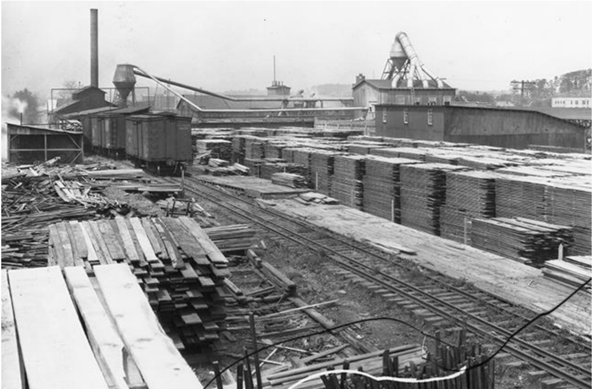
Figure 58A. A detail of the Harris Manufacturing Company.
