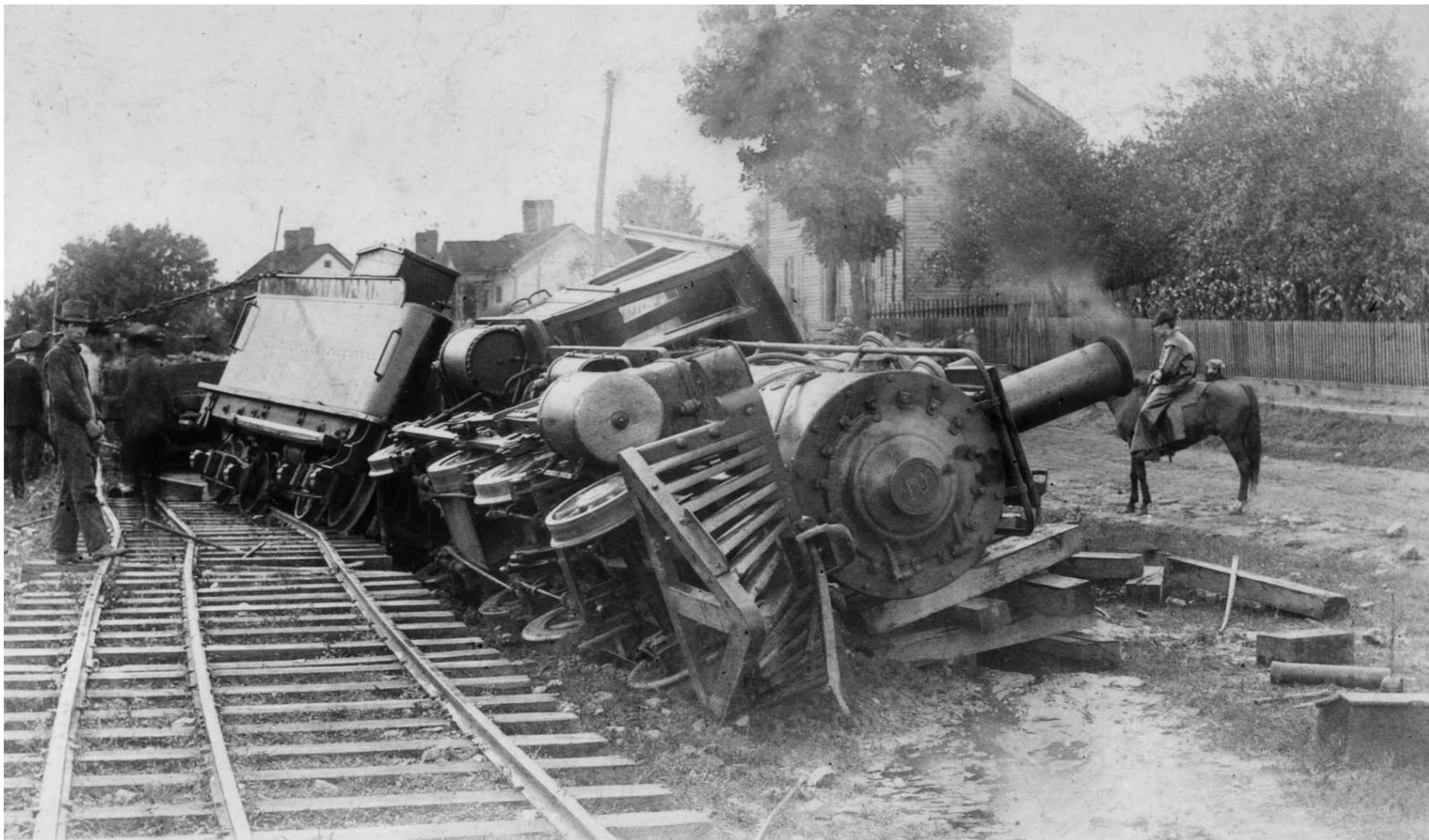
Figure 22. This photograph, of the same accident as depicted in figures 20, 21 and 23, “shows Engine 2 (with its fragile headlight removed) in the process of being hoisted to an upright position.... Original photos attributed to the collections of photographer Burr Harrison.” Historian Johnny Graybeal captioned this photograph: “This photo shows where No. 2 derailed in Johnson City around 1902, It offers an excellent opportunity to see underneath the engine. Parts of the Stephenson valve gear are visible, as well as the brake rigging and the inner strength of the cowcatcher. The wooden cab is warped but not broken. Photo courtesy Ed Bond Collection.” 61 Note the homes in the background, which appear to correspond with 1408/117, 1409/119 and 1411/123 Jobe Street, from left to right, see maps 2 and 3. Also note the link-and-pin coupler.
