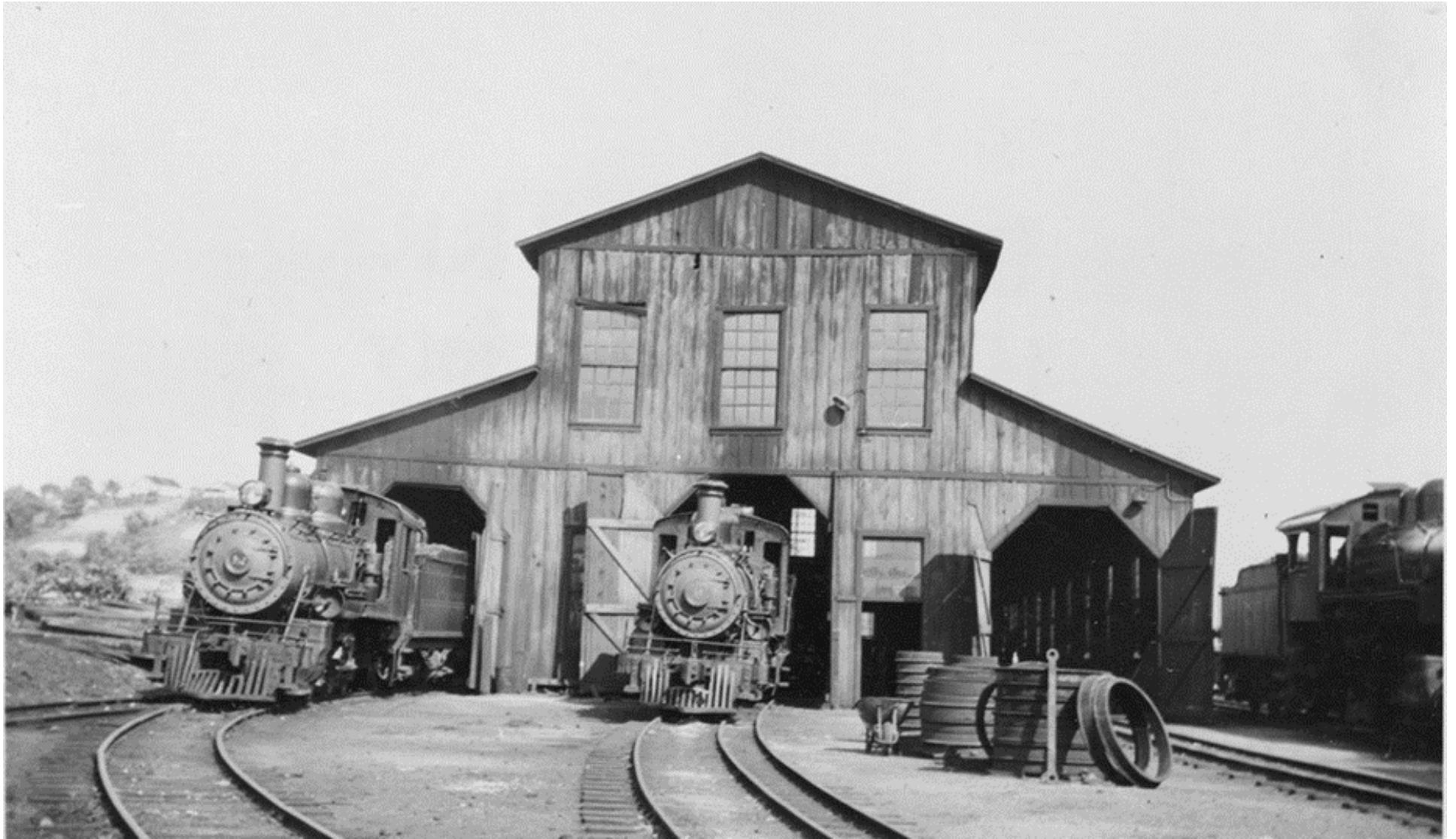
Figure 51. George Allison captioned this photograph: “Narrow gauge locomotives, #12 on the left track and #9 on the center dual track, sit idle outside the Johnson City enginehouse in 1935. Photo from the Cornwall – Martin collection, courtesy of Doug Walker.” 61 Also note the standard gauge engine on the right, which is probably engine #828.
