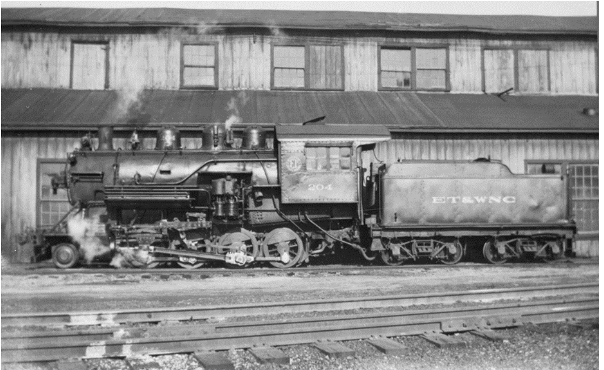
Figure 55. Standard gauge “Engine #204 at Johnson City Engine House,” 7 February 1944. This Lima-built 2-8-0 engine was bought from Alabama, Tennessee & Northern in 1939. 66
