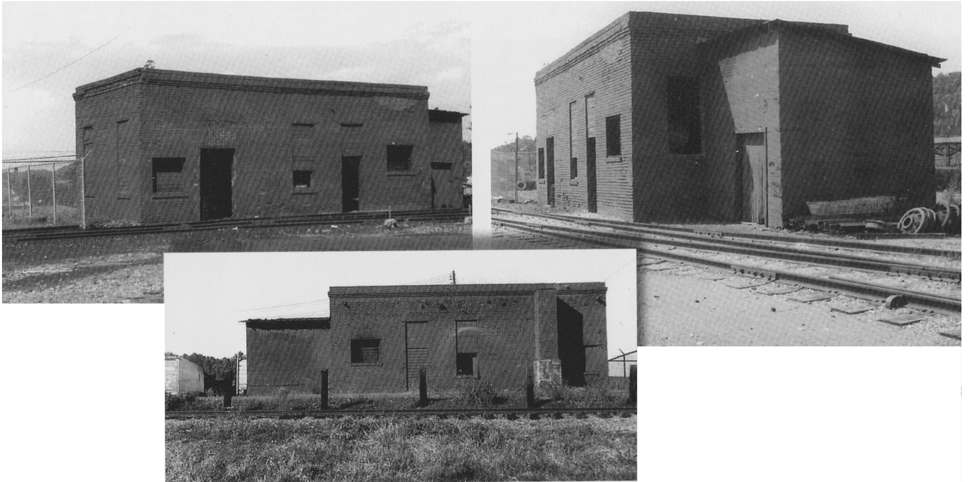
Figure 47. "The Johnson City sand house. Photos from the Allen Curtis Collection." This set of photographs provides interesting views of the east, west and north sides of this building.
