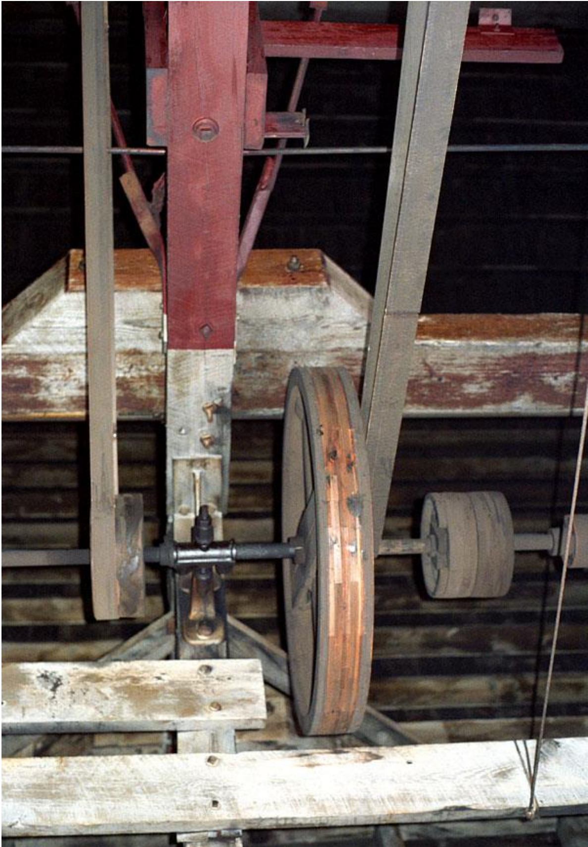
Figure 63. Chris Ford wrote of this photograph: “June 1991... Detail of one of the wooden pulleys on the overhead beltdrive system...” 74
