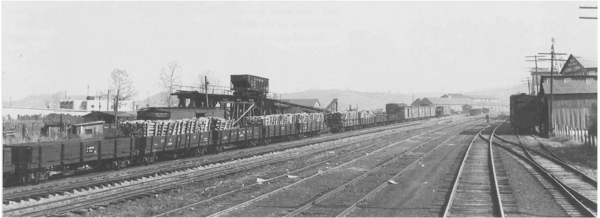
Figure 4. "A string of narrow gauge gondolas loaded with pulp wood sits in the Johnson City dual gauge yards on November 19, 1942. Pulp wood is being loaded from one of the gondolas into Southern boxcar #156424. The dual gauge transfer trestle is in the background and the car shops and engine house can be seen in the distance. The top of the coach house is just beyond the transfer trestle and a coal conveyor is between the transfer trestle and the yard tracks. Photo by Robert W. Richardson." 4 On the right of the photograph is the Harris Manufacturing Company plant. Also note the building in the left background of this image, see Figure 23.
