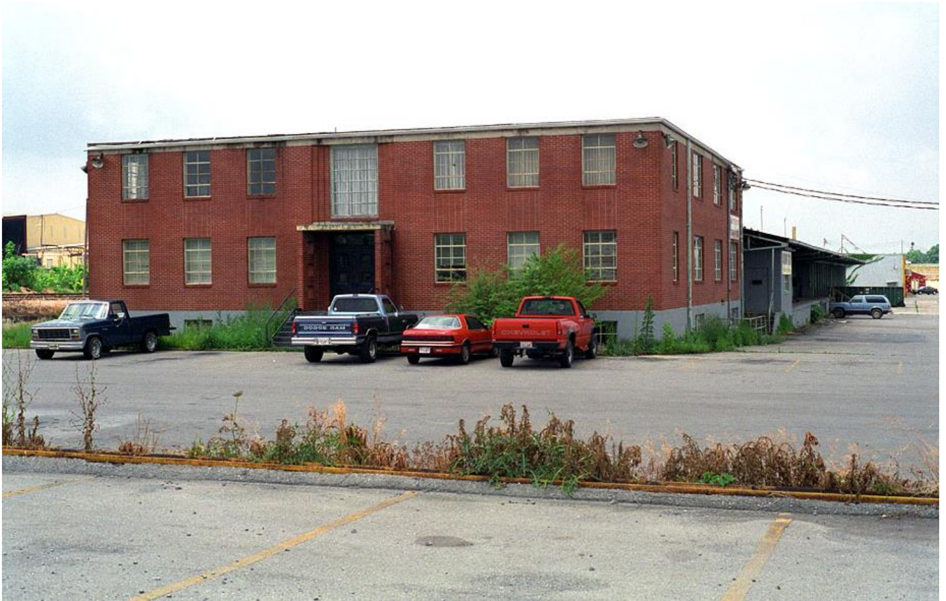
Figure 25. Chris Ford wrote: “June 1997... The old ET&WNC Trucking Company office and transfer building is next door to the old yard office. The original wye and passenger car shop were on this piece of property.” 27 Also note the building in the left background, which appears to have been part of the Harris Manufacturing Company.
