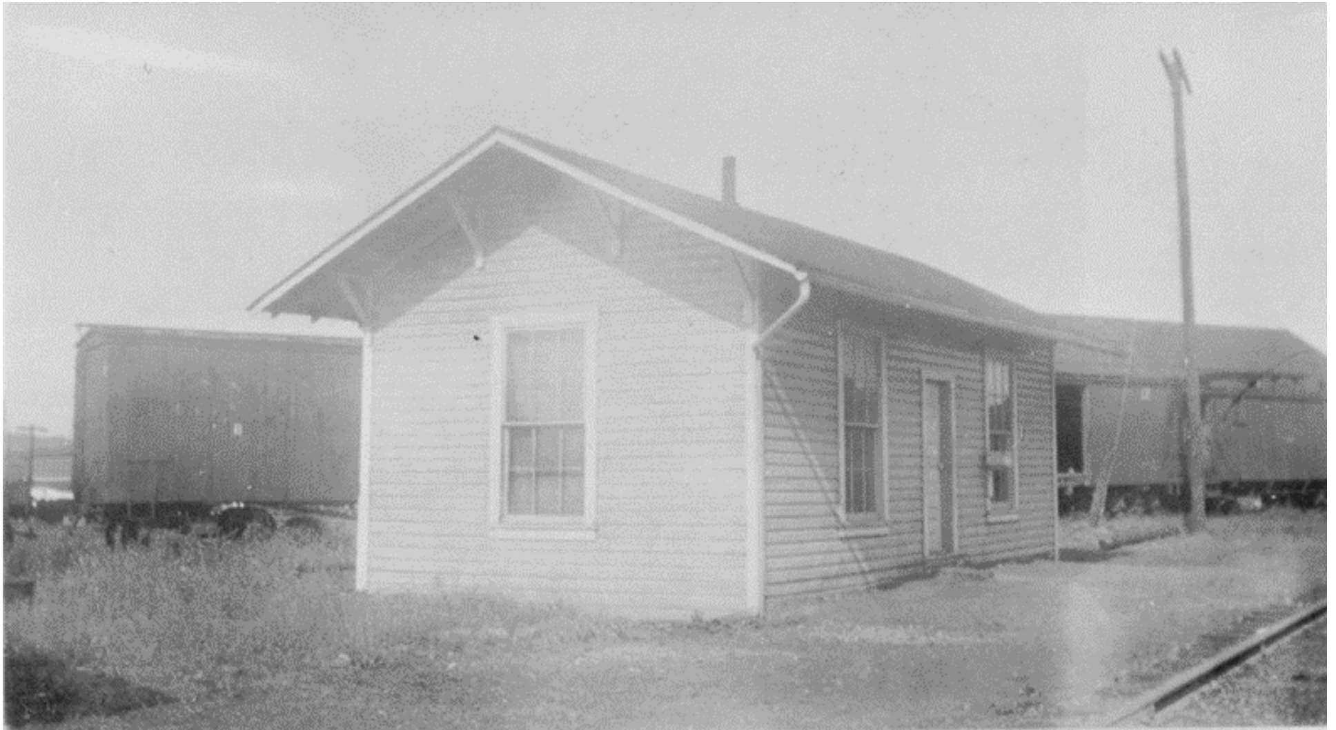
Figure 32. The E.T. & W.N.C. Yard Office at Johnson City was built in 1922 and measured 14' x 30. It was retired in 1937. 40 Note the caboose in the right background.
