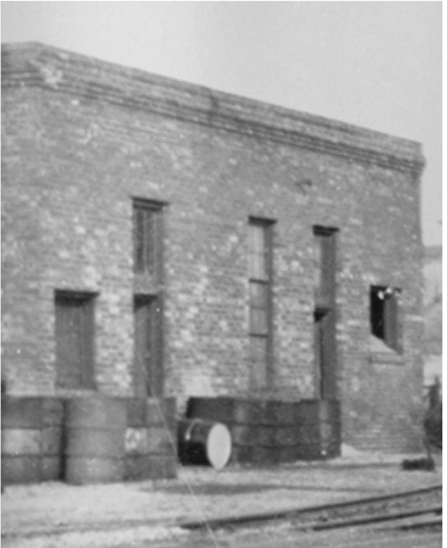
Figure 46A. A detail of the Oil and Sand House.
