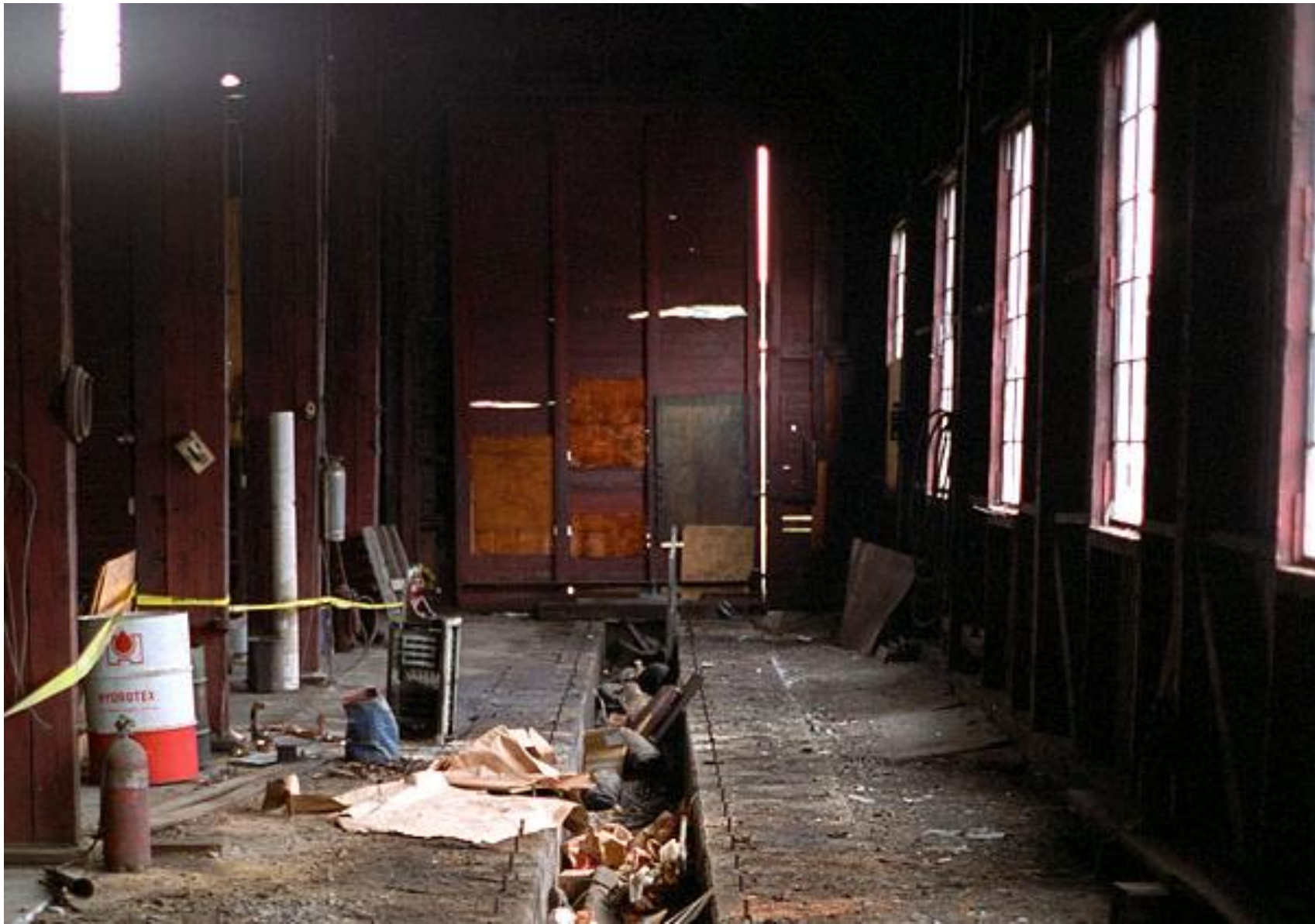
Figure 66. Chris Ford wrote of this photograph: “June 2000... Here’s the old narrow gauge pit on the north side of the ET engine house. We’re looking toward the front doors. They’ve pulled up all the tie sections for the rail and are using the pit for...uhhh...storage it looks like. Note the bolts left in the floor that were holding the tie sections down. Old engine houses just have a certain character and smell to them that says ‘railroad’...” 77
