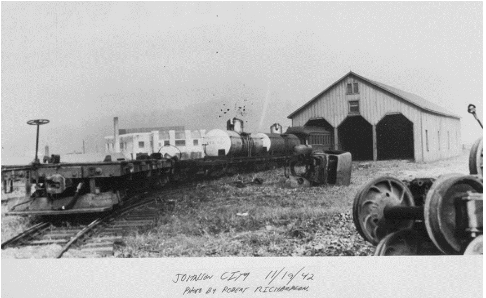
Figure 29. The E.T. & W.N.C. three-stall “Car Barn” was built in 1907 and measured 40’6” x 100’. This photograph was taken on 19 November 1942. Note that, according to google maps, the light-colored building behind the flat cars still exists (although boarded up) and is located at 122 Legion Street. It appears that the Car Barn may have been removed in order to clear space for the new ET&WNC Transportation Company facilities in the early 1950s. 37
