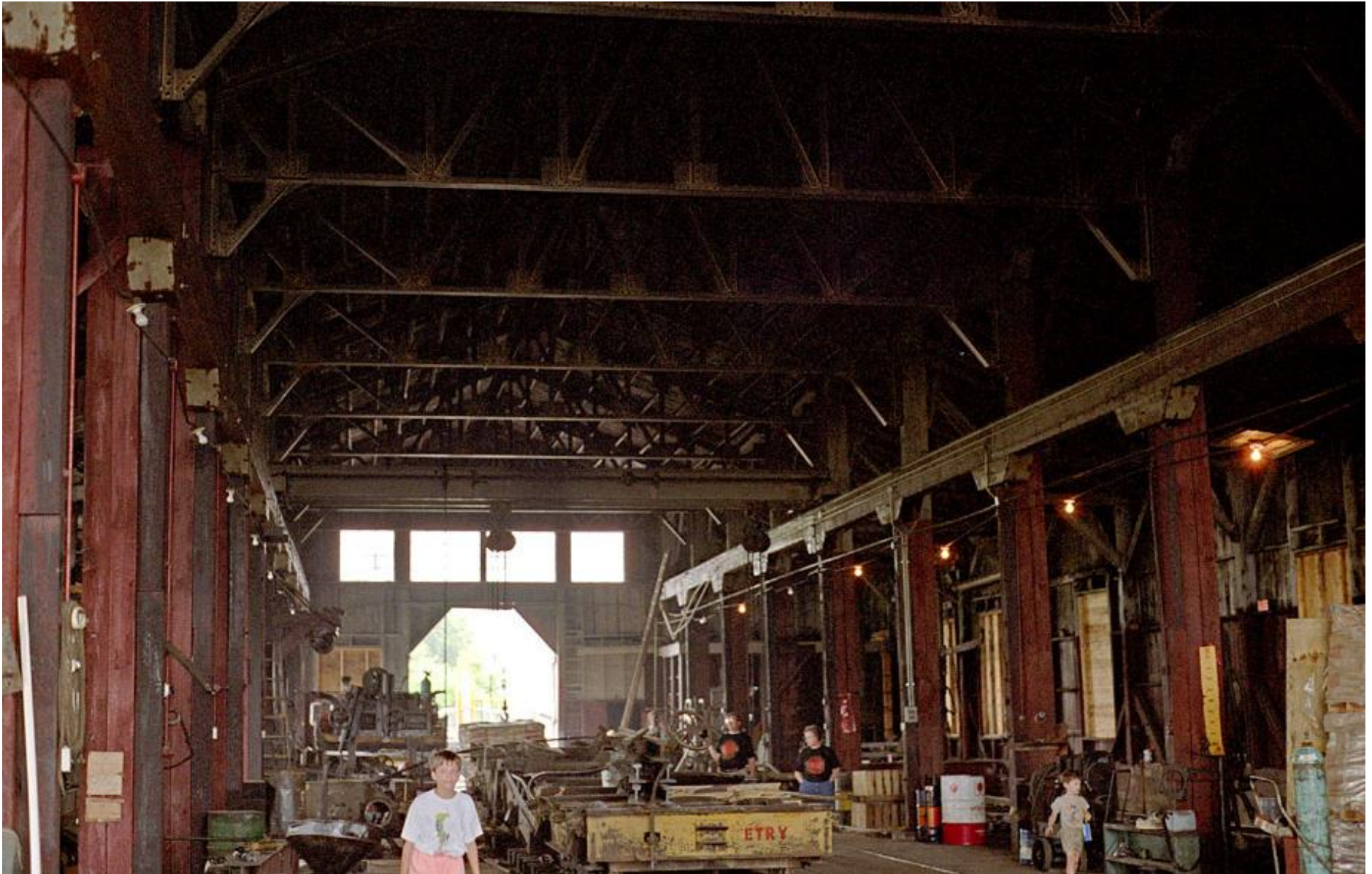
Figure 59. Chris Ford wrote of this photograph: “June 1991 – Johnson City Enginehouse Interior – Impressive is the word of the day for this rare tour of the old ET&WNC enginehouse in Johnson City. I don't think this structure has changed much inside over the years except for the clerestory roof being removed. Everything had such a wonderful color and patina that only time, steam and grease can produce. We're looking toward the back of the building in this photo. The blacksmith area is on the back right. The overhead pulley drive is on the left.” 70
