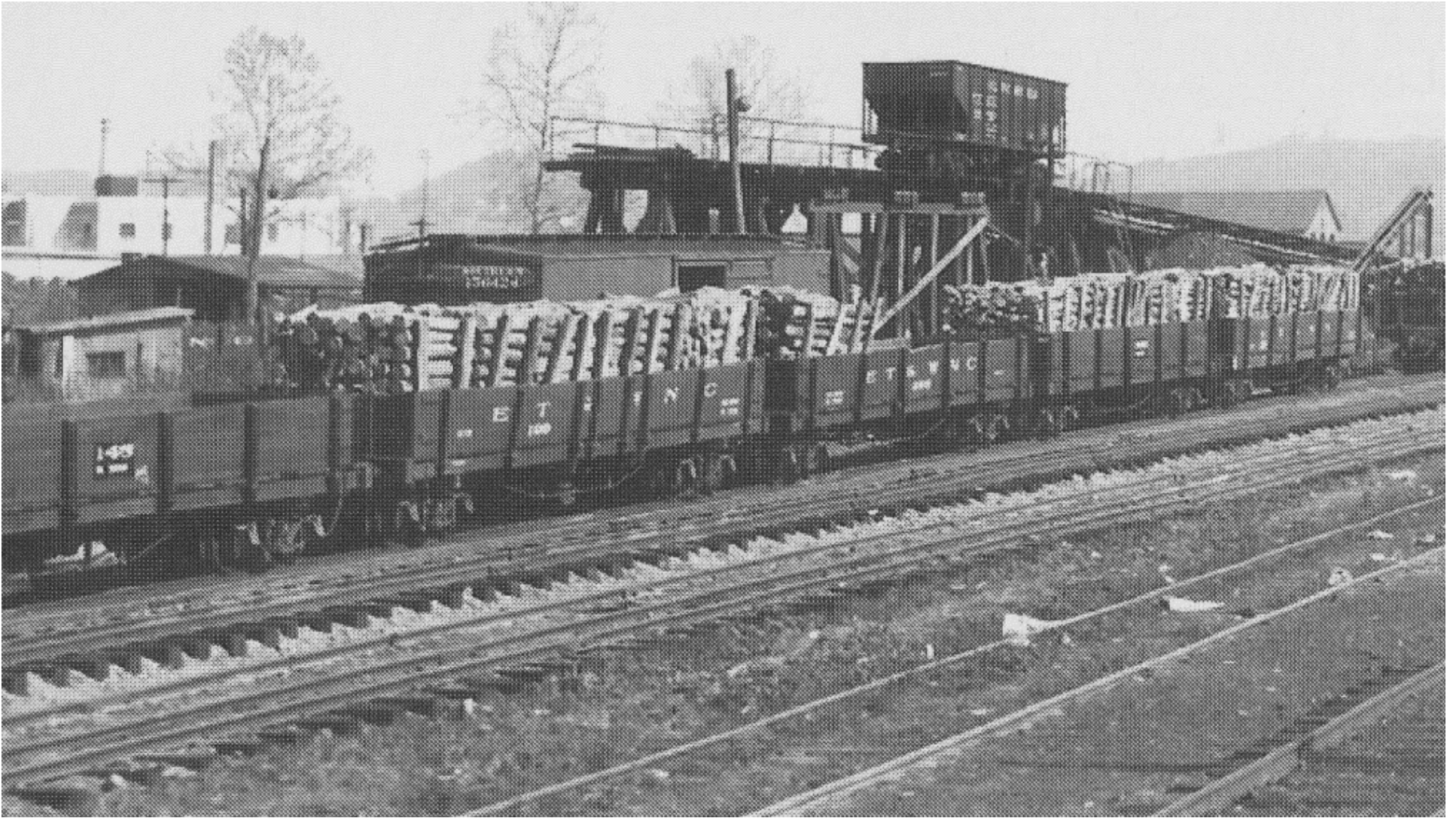
Figure 4A. A detail of the Coal Transfer Trestle, which shows some detail of the structure.
