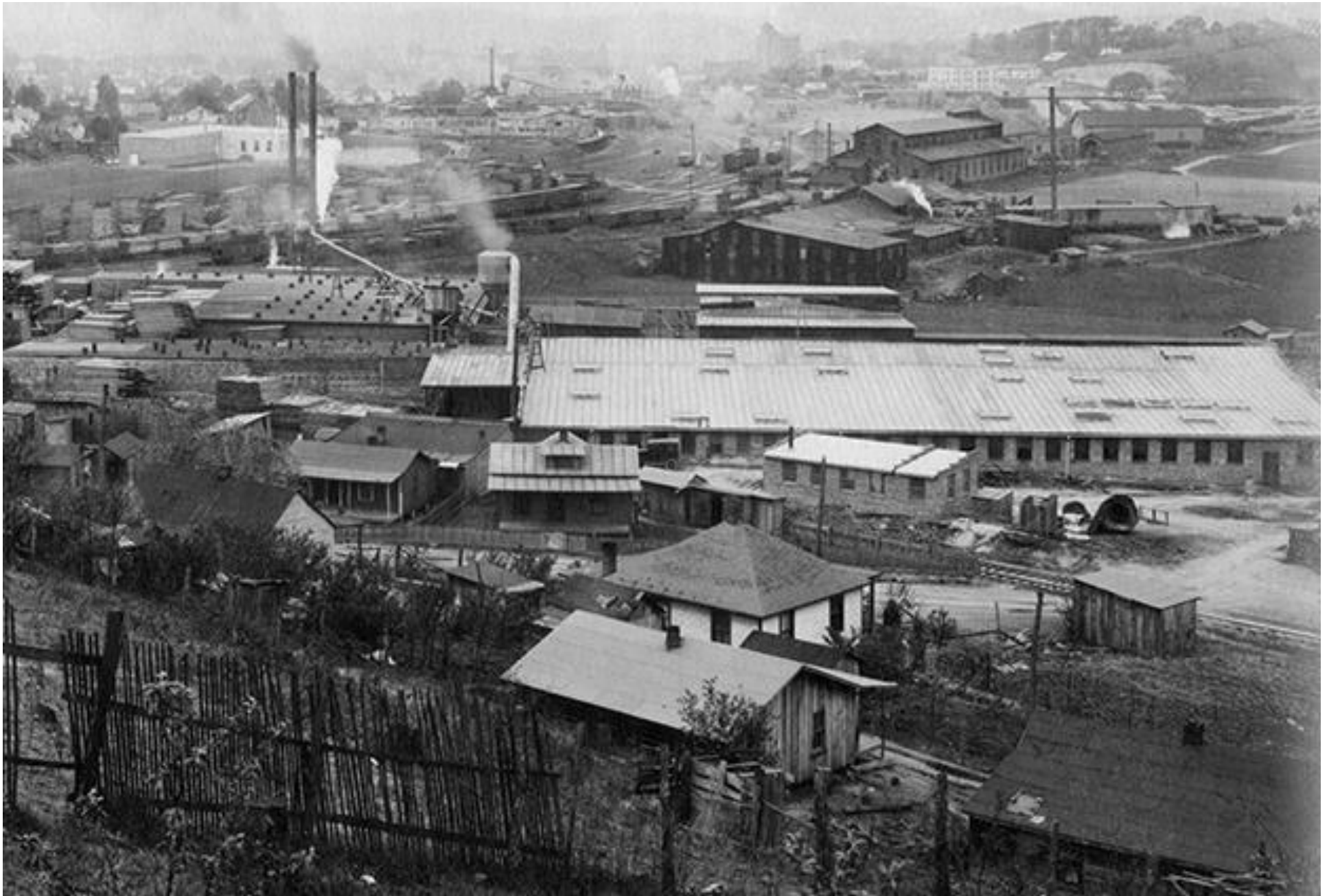
Figure 76C. A detail of the Sells Manufacturing Lumber Company, which is the large building near the center of the photograph.
