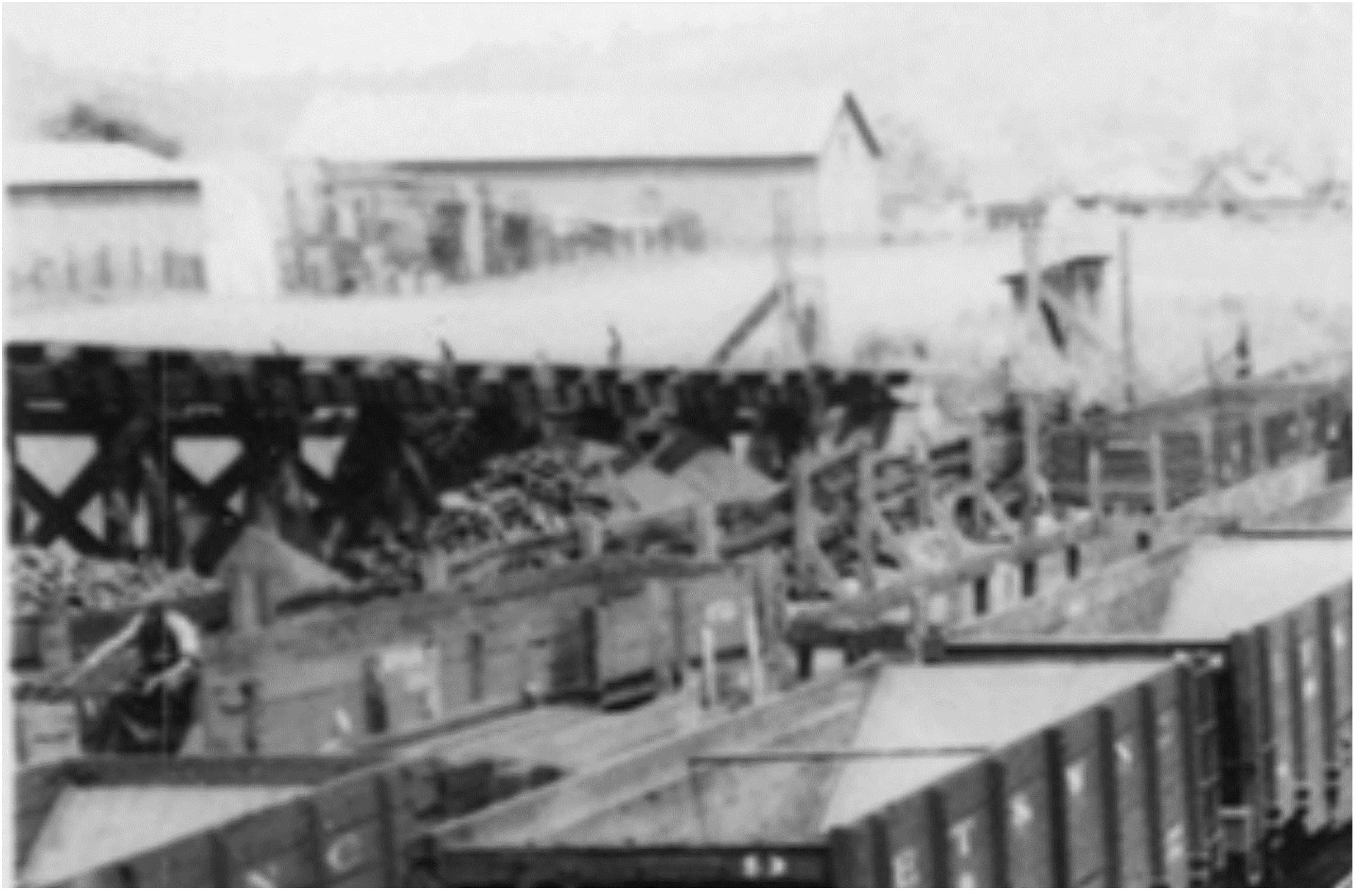
Figure 9A. A detail of the coal transfer trestle. Apparently, the building in the middle background is the Car Barn of the E.T. & W.N.C.
