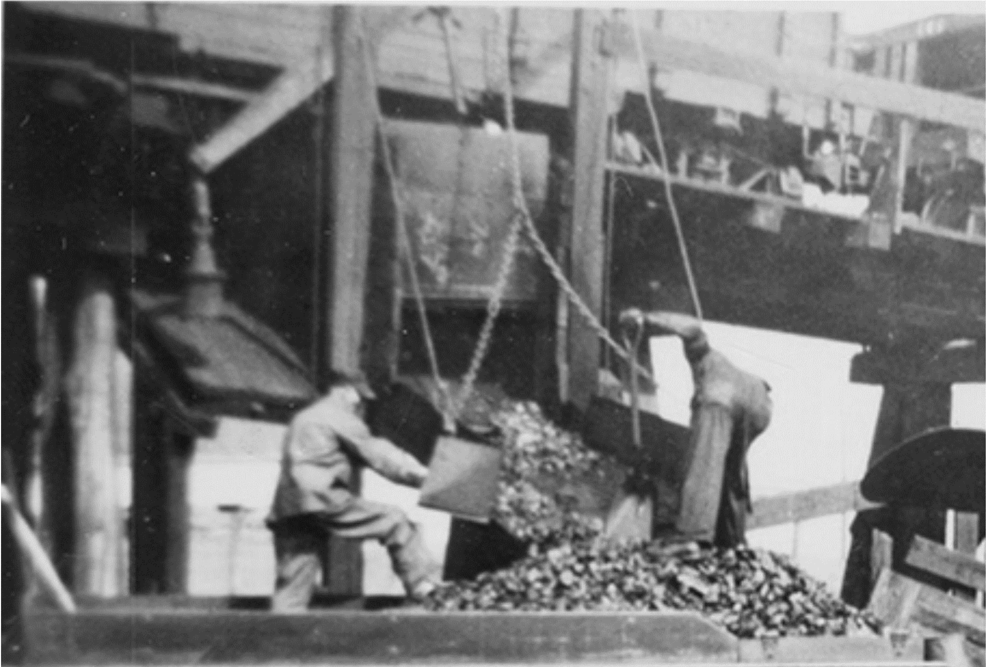
Figure 6A. A detail of the coal transfer chute.
