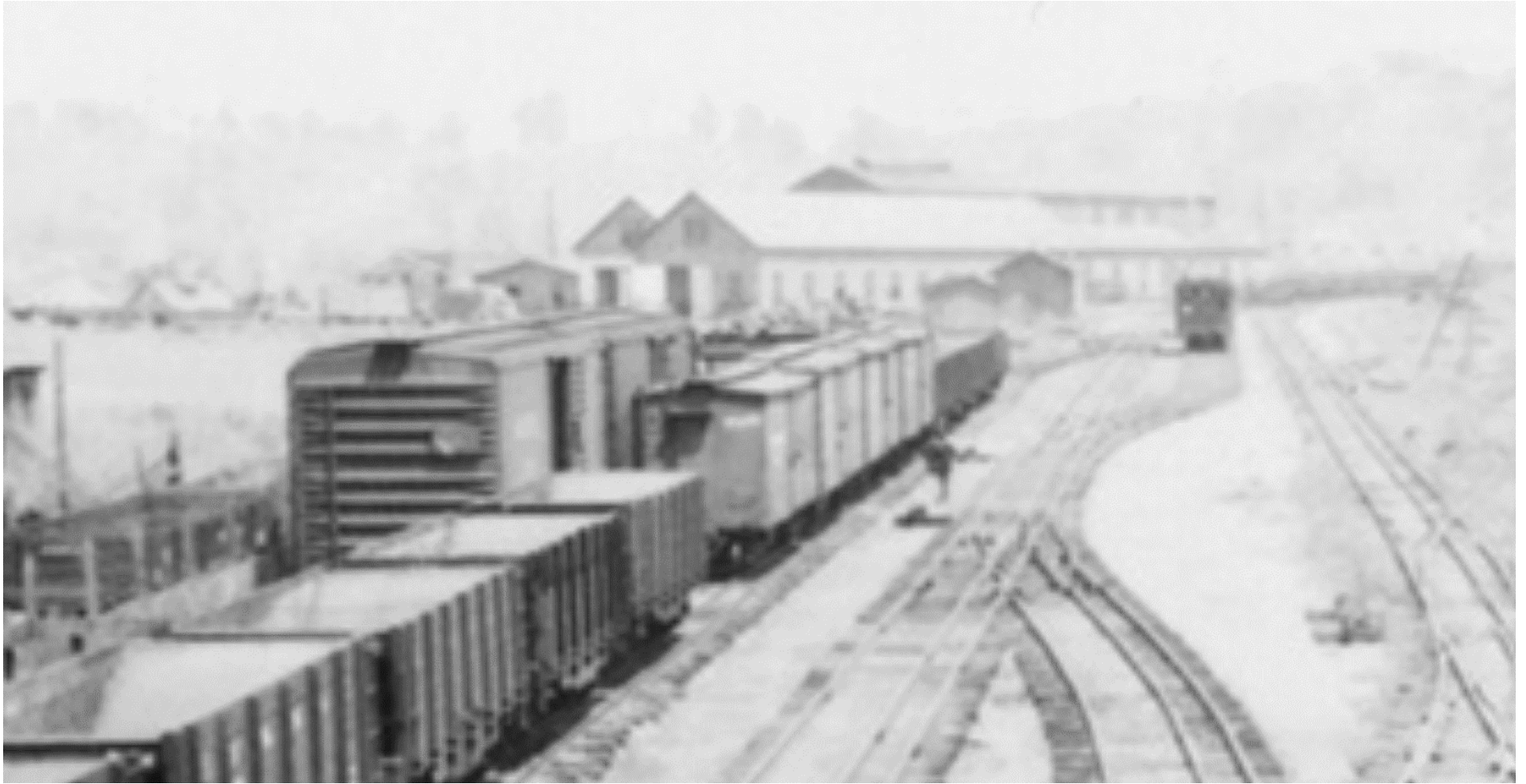
Figure 9A. A detail of the E.T. & W.N.C. shops. Note the Truck Repair building (completed in 1937), with the Yard Office in front of it, and the Engine House in the background. It appears that five tank cars are to the right of the Engine House. Also note the size difference between the narrow gauge and standard gauge box cars, near the center of this image.
