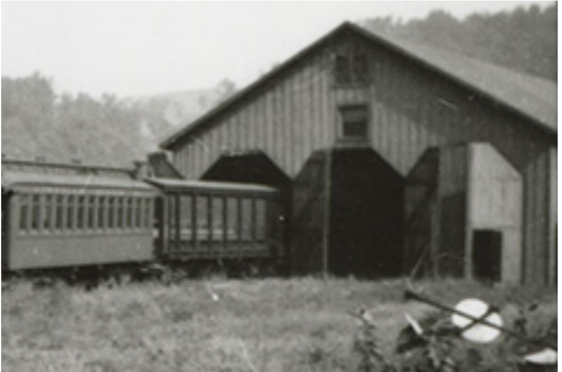
Figure 30A. A detail of the Car Barn/Coach House.
