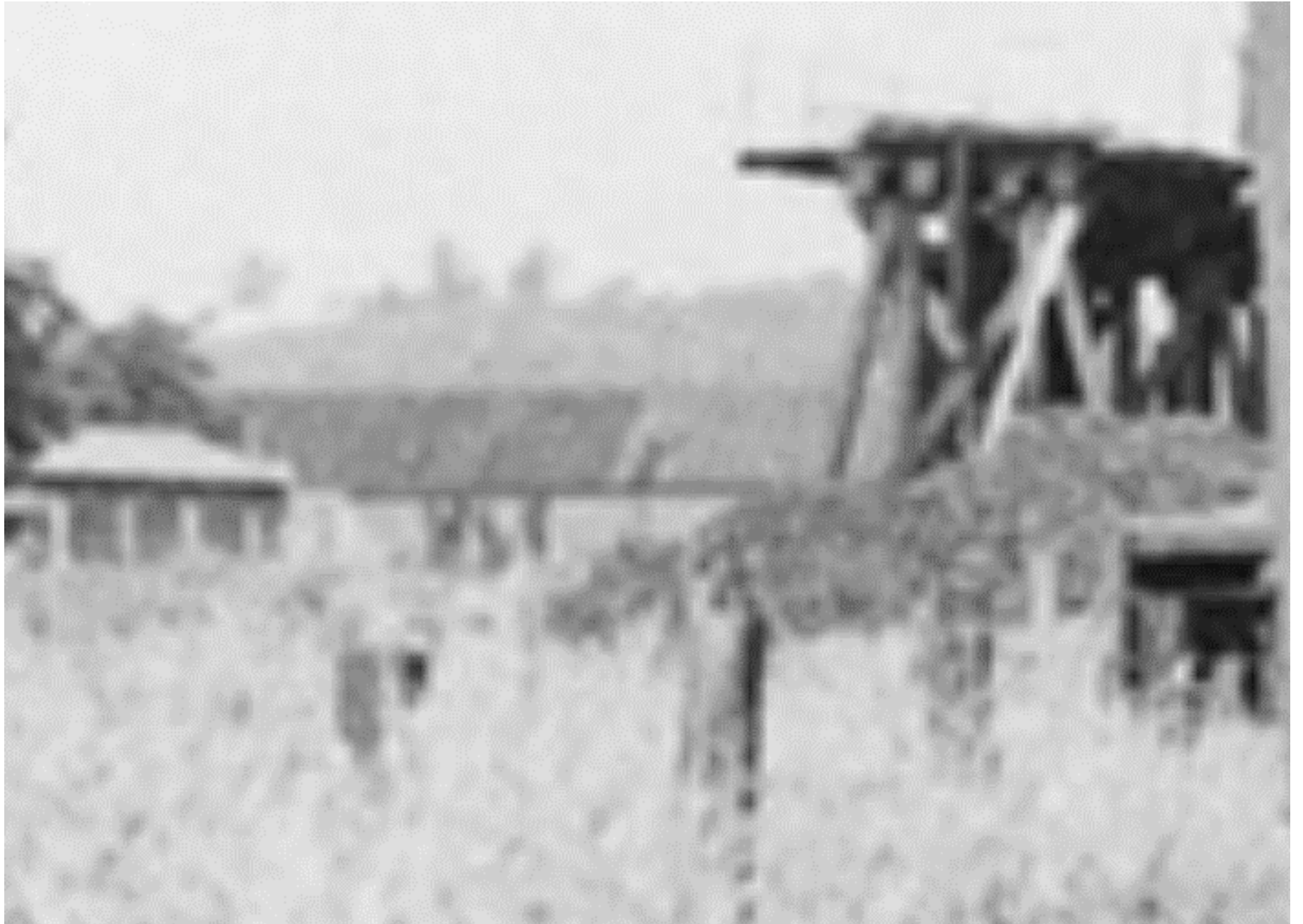
Figure 3A. A detail of the west end of the coal transfer trestle.
