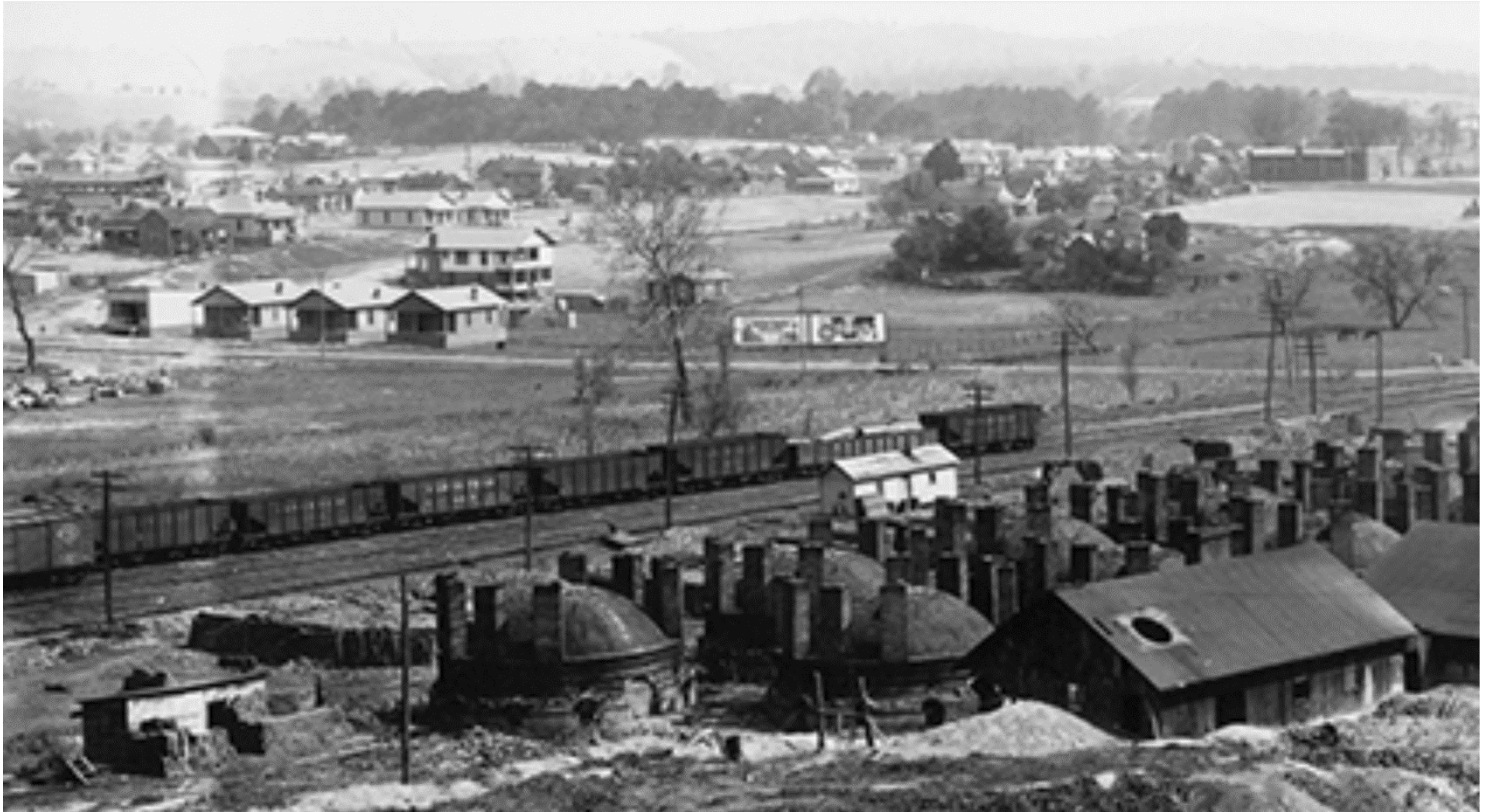
Figure 36B. A detail. This image appears to include 13 “Down Draft Kilns”, which matches the number shown on Map 16.
