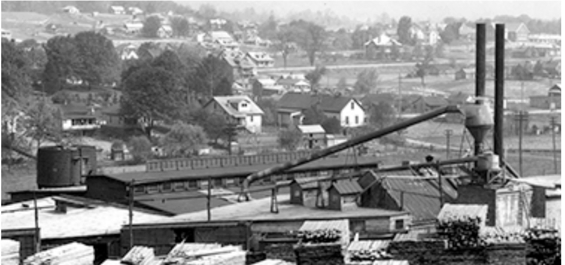
Figure 23B. Another detail of the Tennessee Box Company. Note the railroad water tank on the left. The building with the clerestory roof appears to still be the “Box Factory” and the building with the two smokestacks and cyclone still appears to be a boiler house. Also note the railroad cars on the spur in front of the “Box Factory”.
