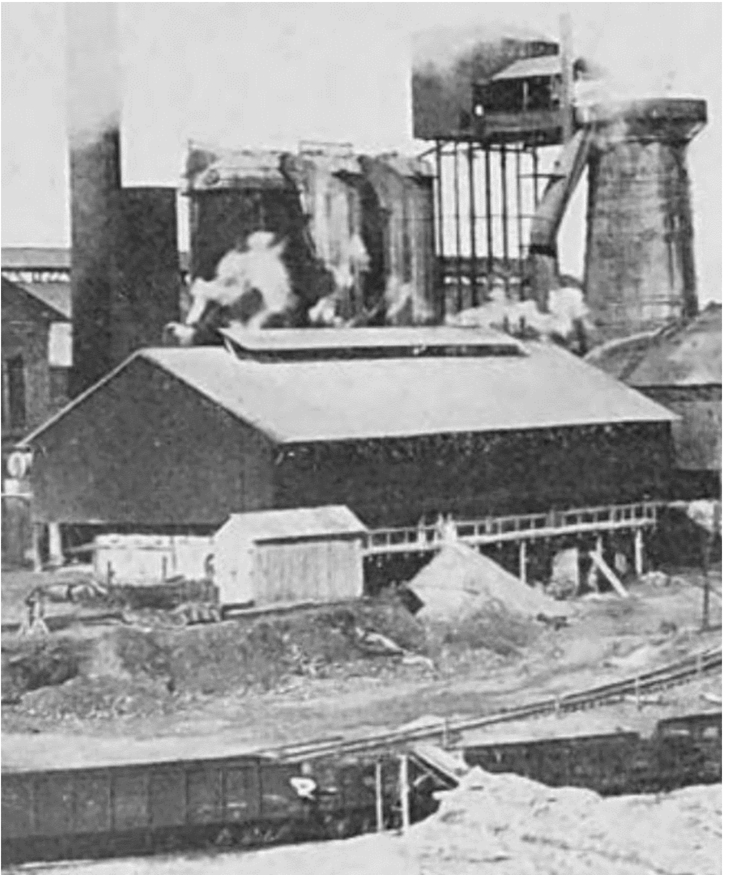
Figure 82A. A detail of the boiler house, the “Eng. Ho.,” the chimney, the elevator and the furnace. 324 Revised 24 September 2024.
