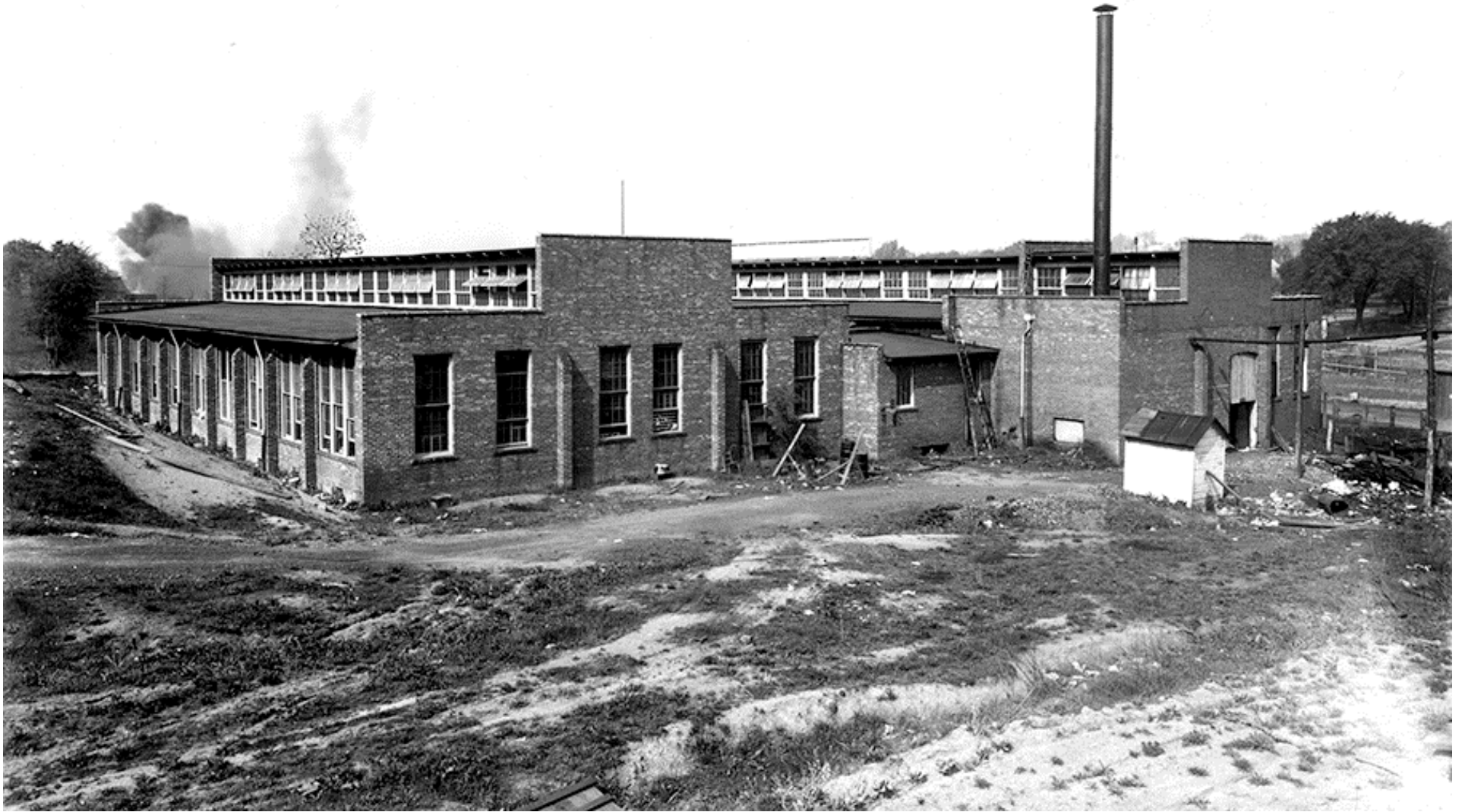
Figure 19. "New Street Plant, Johnson City Mills" looking northwest. 83 The "Knitting Mill" is on the left and the "Dye Ho." is on the right. Note the overhead steam pipe, attached to the "Dye Ho." on the right. This pipe was connected to the boiler house of the Tennessee Box Company. The small, light-colored, building housed a "D.H." (Dry Hydrant? Double Hydrant?), see Map 12D.
