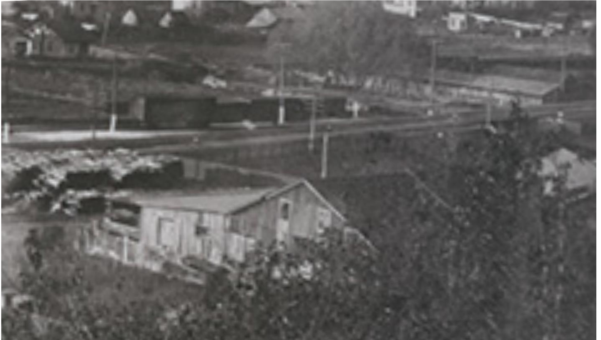
Figure 3A. A detail of the “Store Ho.,” which was depicted on Sanborn Insurance maps from 1891 to at least 1920. This building initially belonged to the Stratton & Stratton operation, begun by 1887, and renamed the Watauga Lumber Company by 1890. This building had been built by January 1891. 14 The Watauga Tannery purchased this store house by 2 May 1895, according to the Johnson City Comet .
