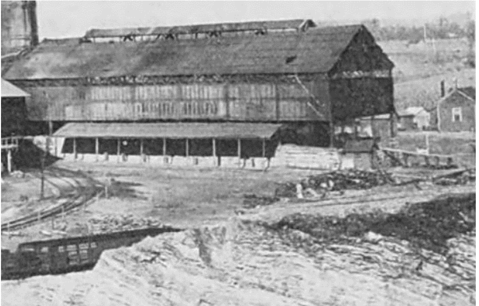
Figure 82B. A detail of the “Cast Ho.” Note that the small building against the right side of the “Cast Ho.” appears to be the “Scale Off.” with the tramway nearby. Two “Car Shed” or “shed roofs have been added to the stock [should read “Cast”] house... to cover the trams that carried ingots out to the railroad spur track”, see Map 31B. 325
