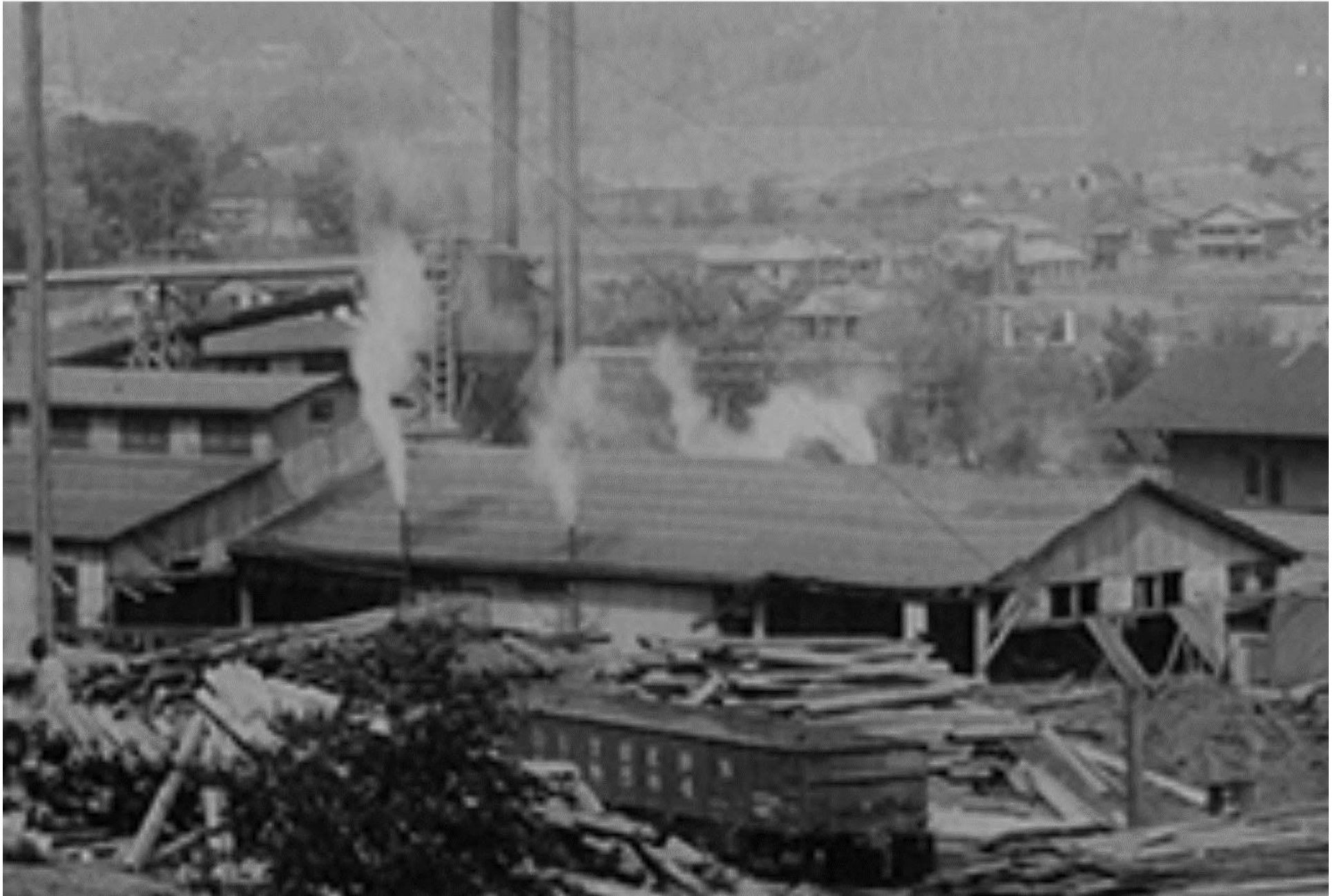
Figure 29C. Another detail of the Southern Bending Company. This one depicts the “Saw Mill”.
