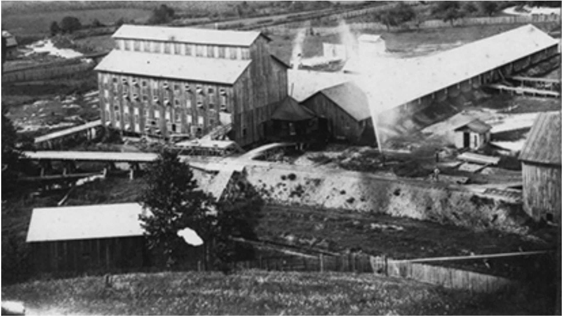
Figure 1A. A detail of the Watauga Tannery. The building in the left foreground appears to be the “Hair House” (labeled “N” on Map 3A), which has a platform leading across the railroad to the multi-story building (labeled “F”). This multi-story building had “Rolling & Finish’g” on the “1 st ” floor and “Drying” on the “2d”. The long building (labeled “D”), to the right of the multi-story building, appears to be the “Yard Ho.” The roof of the “Beam Ho.” (labeled “E”) appears between the multi-story building and the Yard Ho.” The small building to the right of the “Yard Ho.” appears to be the brick one, which is not labeled on Map 3A. The mainline of the E.T.V. & G. railroad is also visible behind the multi-story building. Note that the buildings labeled “A”, “B”, and “G” on Map 3A, dated January 1891, should be visible in this photograph, but are not present; consequently, this photograph appears to predate 1891.
