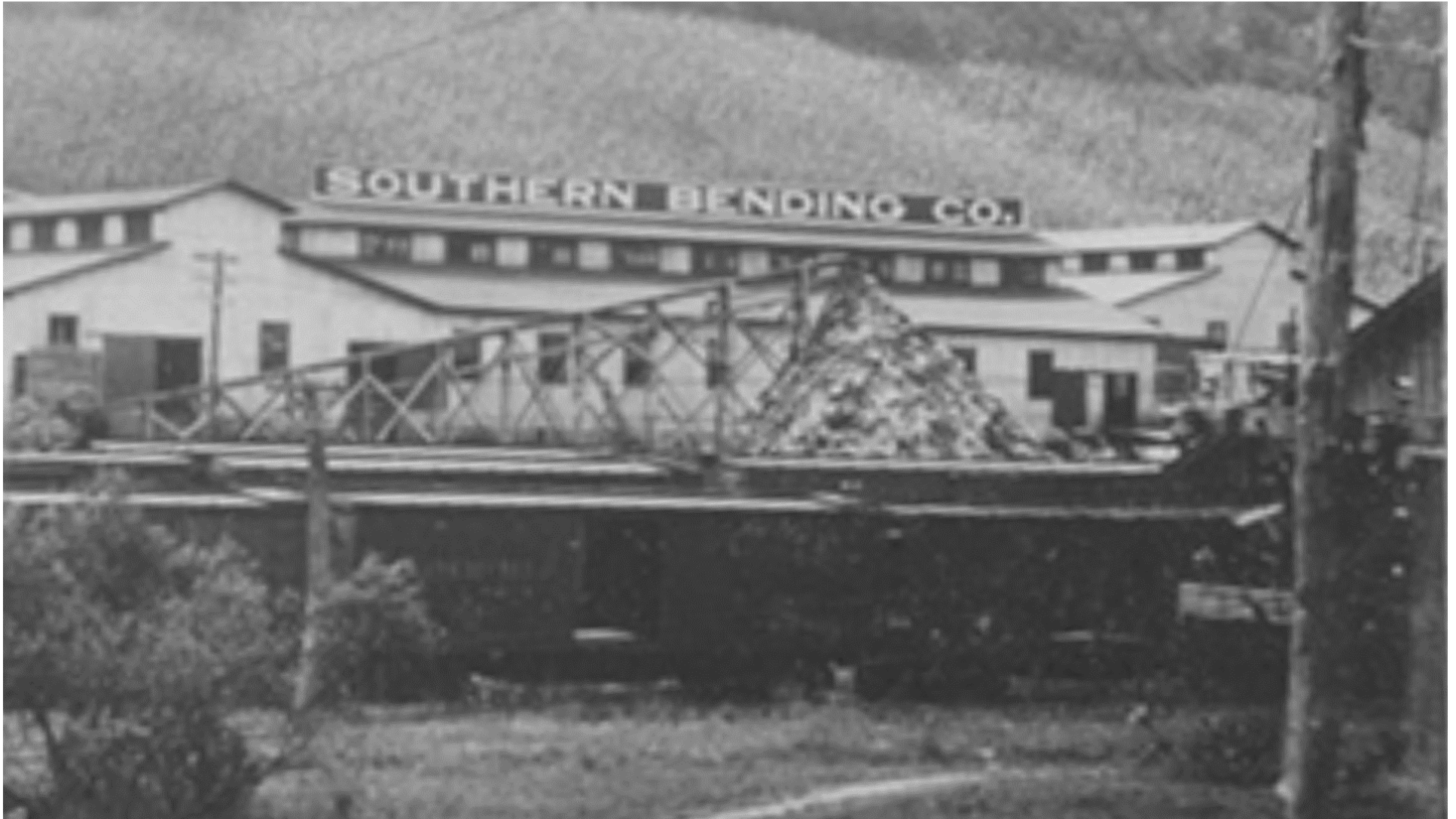
Figure 27A. The iron clad building on the left and in the center of this photograph contains the “Rim Dep’t.” and “Wood Working Machinery”. The iron clad building on the right contains the “Pearson Loom Supply” and “Bobbin Co. Mill.” Note that the structure partially visible on the right appears to be the east end of the old Clinchfield Freight Depot. Also note the “Waste Conveyer” in front of the “Rim Dep’t.” in the center of this photograph. See Map 15C. This photograph appears to date to between 1920 and 1924.
