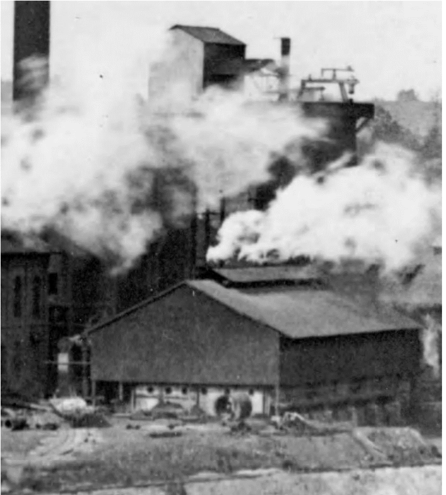
Figure 80C. A detail of the boiler house (with three boilers) with the ore elevator to the top of the 75' furnace behind it.
