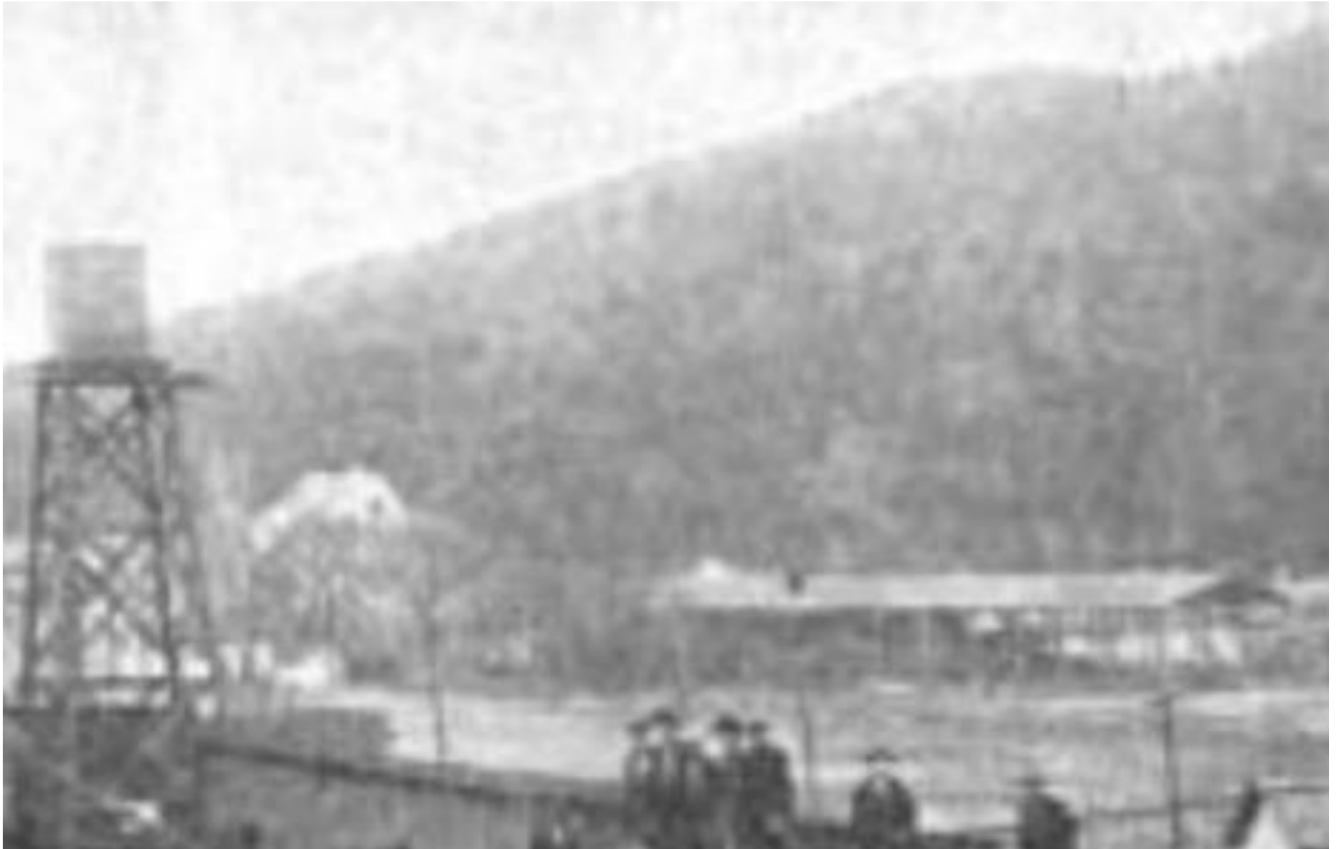
Figure 4. It appears that this photograph, taken by 1904, looks over the American Cigar Box Lumber Company and along Division Street, north across the E.T. & W.N.C. Railroad mainline, toward the Gildersleeve residence (the light-colored building to the right of the water tower) and Bark Shed No. 3 of the Watauga Tannery, on the right, see maps 5 and 6. 15
