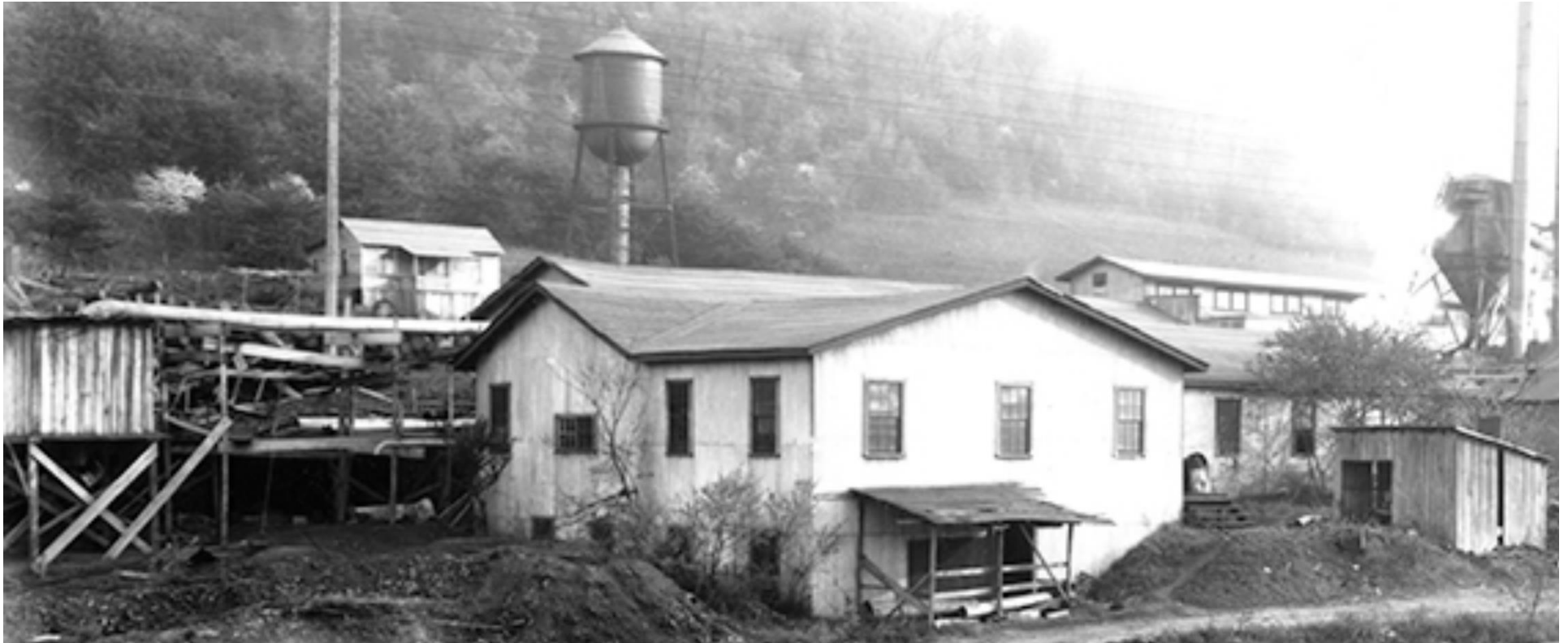
Figure 28C. A detail of the Southern Bending Company, depicting the iron clad building that housed “Machine & Saw Filing”, as well as a “280 amp dynamo” on the left. Note the platform to the left of this building, with the “Log Derrick” behind it. Also note the water tower “40,000 [gallon] gravity W.T. on steel trestle, total height abv. Sprklr heads 60” and the building to the left of it, which was not depicted on Map 15A. The tall building in the right background contained the “Bending Dep’t.”. The boiler house and black smith shack are also visible on the right. This photograph appears to date to between 1920 and 1924.
