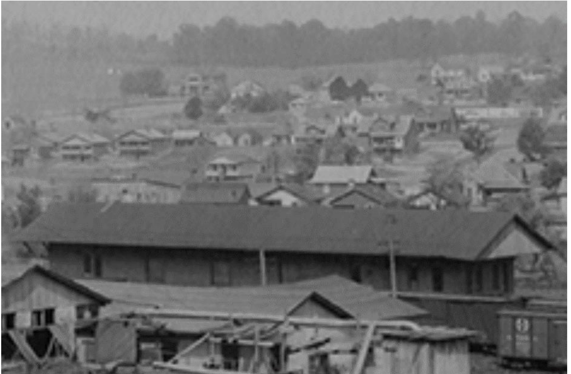
Figure 29F. A detail that includes the south and east sides of 3 C's freight station/S. & W. station/C.C. & O. freight depot, note the Santa Fe boxcar on the right. It appears that this image dates to between 1920 and 1924.
