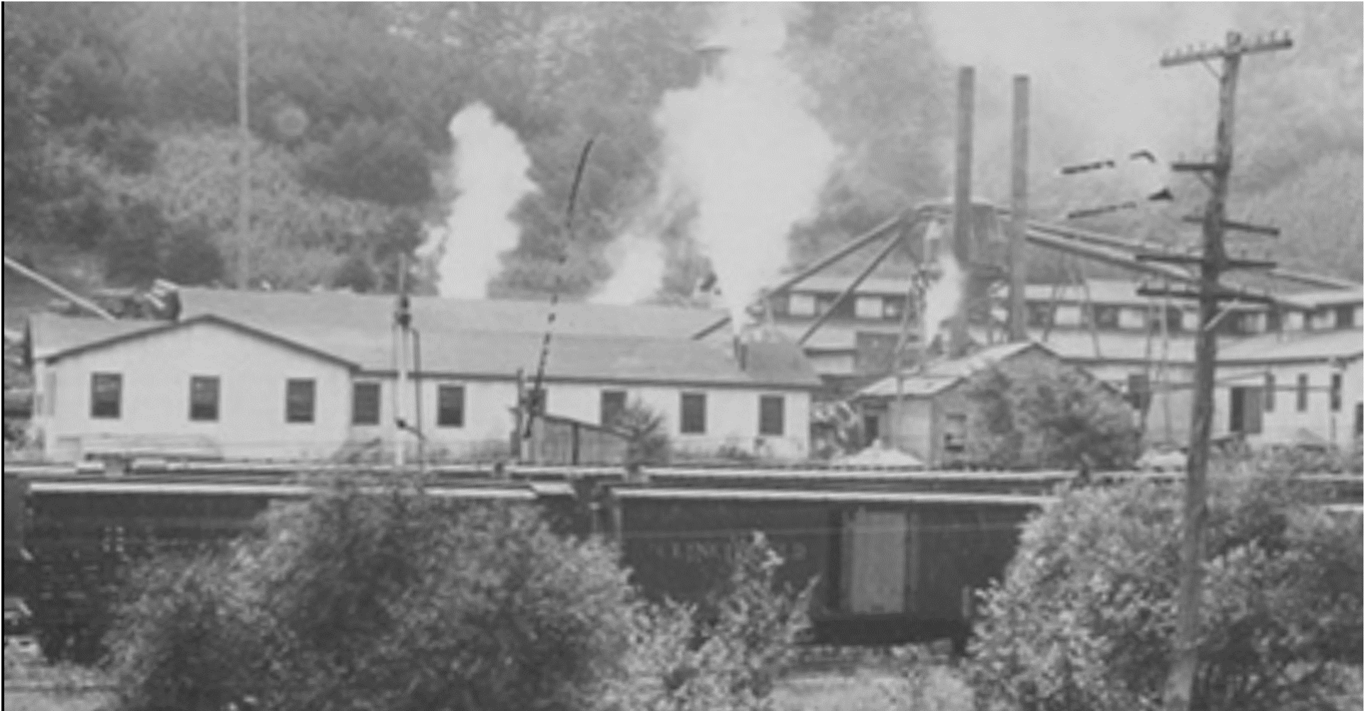
Figure 27C. A detail of the Southern Bending Company, depicting the iron clad building that housed “Machine & Saw Filing”, as well as a “280 amp dynamo” on the left. The right side of this image includes the boiler house (with cyclone) and the “Bending Dep’t.”. Note Clinchfield boxcar, in the central foreground, and the four dust conveyors leading into the cyclone on the boiler house. Note the pole behind the building on the left, this pole was a “Log Derrick” and was used for moving logs around the yard. Also note the shack in front of this building, which was used for black smithing. The Sanborn map of February 1920 indicates only one dust conveyor leading to this cyclone, which indicates that this photograph was probably taken after the map from February 1920 was made. The Unaka Flooring Company had acquired this facility by 1924, consequently, this photograph appears to date to between 1920 and 1924.
