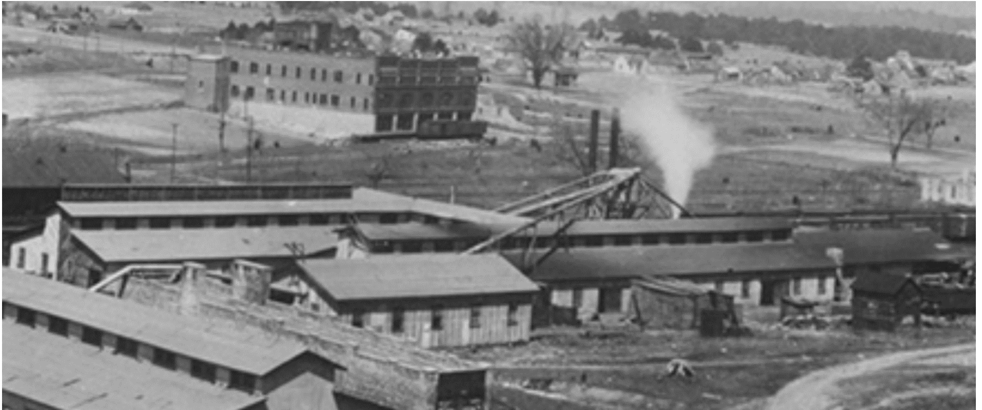
Figure 30B. A detail. The iron clad building, with the clerestory roof on the left, contained the “Rim Dep’t” and “Wood Working Machinery”. The relatively small, detached building was also iron clad and contained the “Bobbin Fact’y” and was connected to the cyclone with a “metal dust conveyor.” The building with the clerestory roof just behind and to the right of the small detached building contained the “Bending Dep’t” and “Wood Working Machinery” under the portion with the “Raised Vent”, with the “Saw Mill” in the portion, to the right, without the “Raised Vent”. Note that the brick boiler house is behind the “Bending Dep’t.” This photograph appears to date to between 1920 and 1925.
