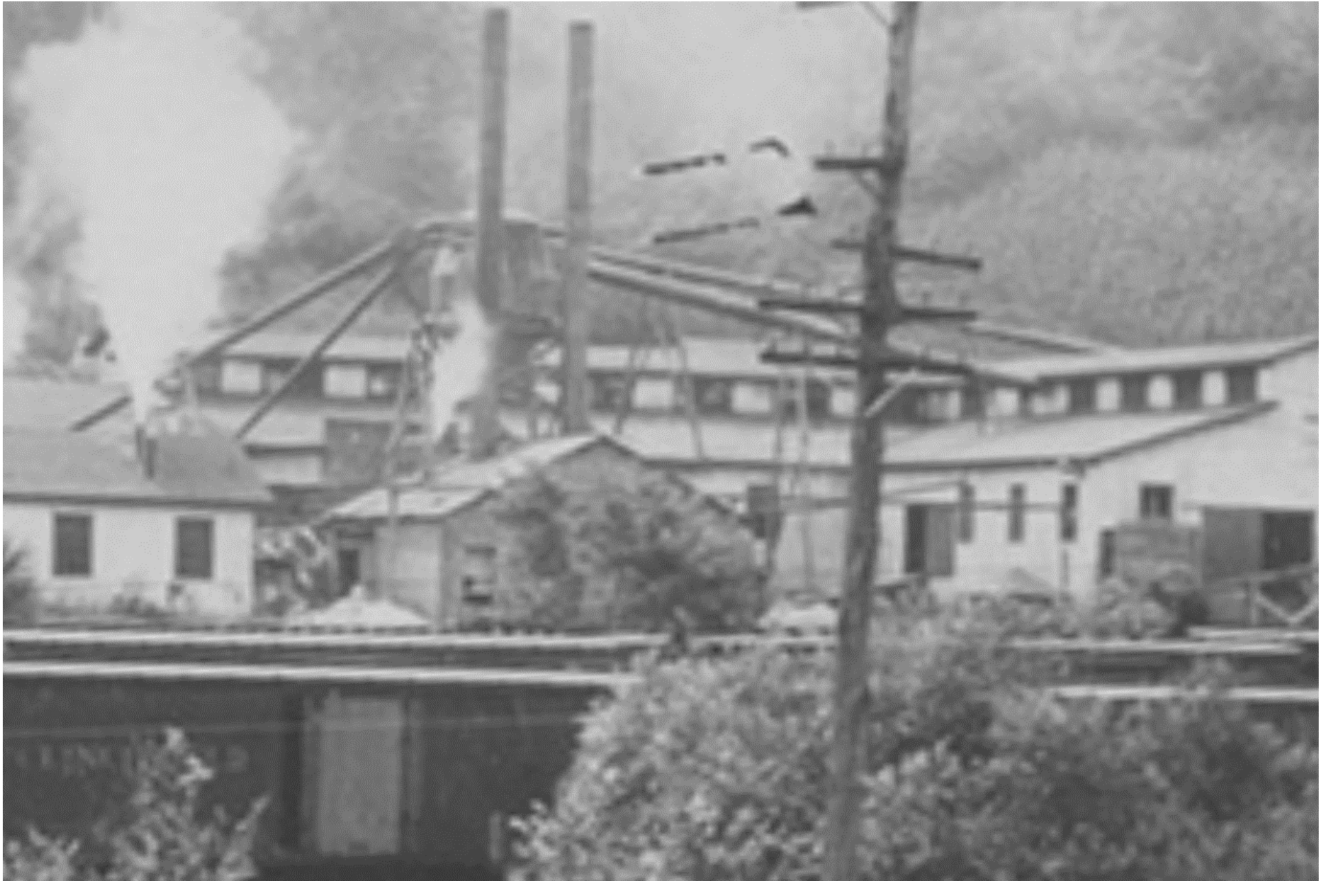
Figure 27B. A detail of the boiler house and the cyclone of the Southern Bending Company, see Map 15C.
