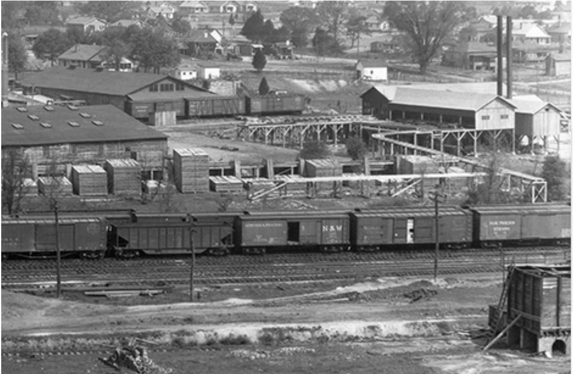
Figure 53E. A detail of what appears to be the McCorkle Lumber Company, which, from 1925 to 1928, occupied the land previously occupied by the Hotel Carnegie. Note the structure in the lower right of this image, which appears to be part of the Johnson City Shale Brick Company.
