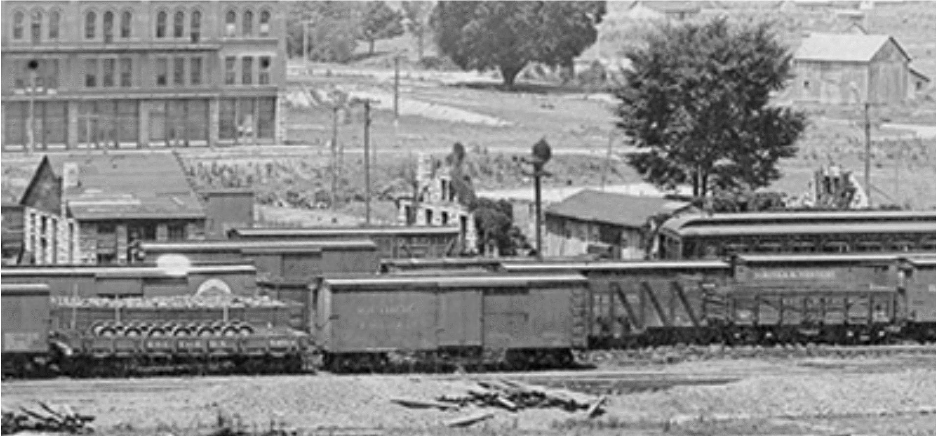
Figure 51A. A detail of the unfinished the 3 C's depot, looking north. It appears that the stone building, on the left, was roofed over by the South & Western Railway in 1905 for use as a carpenter shop. Given that the Hotel Carnegie burned down in 1910, this image appears to date to between 1905 and 1910.
