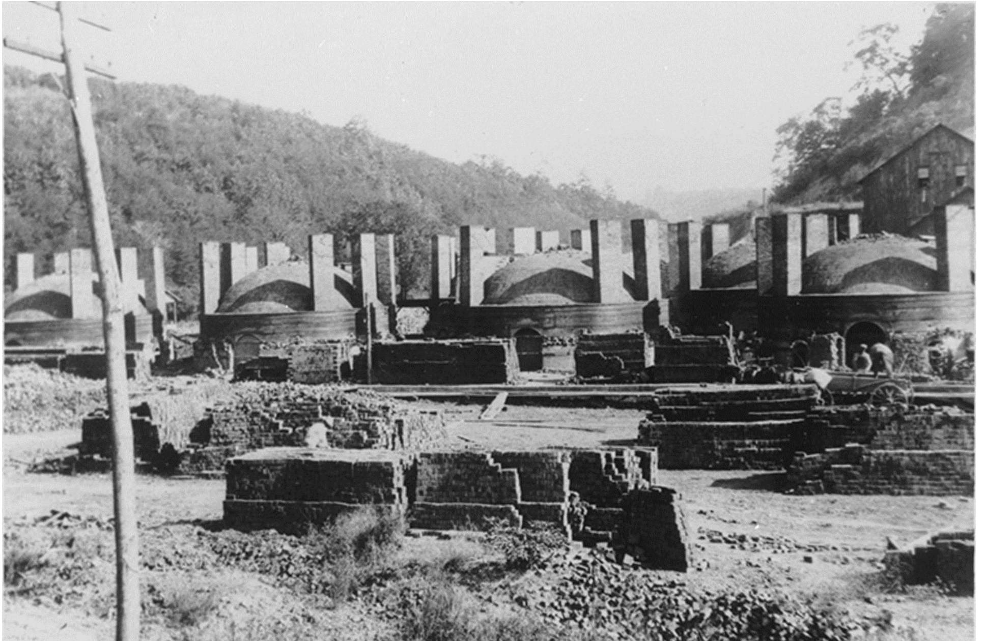
Figure 37. "General Shale, Johnson City Plant, 1928," note that the Johnson City Shale Brick Company expanded in 1928 and became the General Shale Products Corporation. 174
