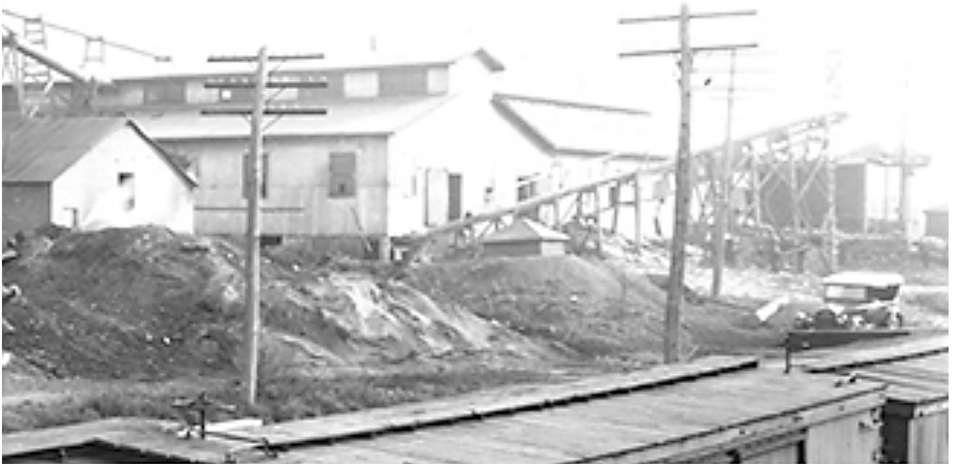
Figure 28A. A detail of the Southern Bending Company, which depicts the boiler house, the “Rim Dep’t.” and the “Waste Conveyor”, from left to right. Note that only two dust conveyors enter the cyclone, indicating that this photograph was taken after the Sanborn map of February 1920 was produced, but before the images in figures 27 and 30 were taken, consequently, this photograph appears to date to between 1920 and 1924. Also note the early model car on the right.
