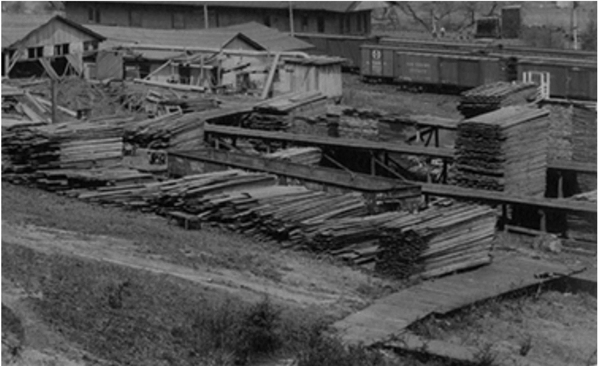
Figure 29A. A detail of the Southern Bending Company. This one depicts the lumber yard and platforms on the right, “Average height of lumber & Piles 12”, note the gondola in the lumber yard. On the left is the “Saw Mill” and to its right can be seen the iron clad building that housed “Machine & Saw Filing”, as well as a “280 amp dynamo”. Also note the “Old C.C. & O. R.R. Depot” in the background, as well as what appears to be a Santa Fe boxcar. This photograph appears to date to between 1920 and 1924.
