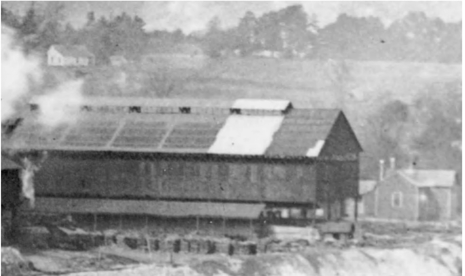
Figure 80D. A detail of the “Cast Ho.,” with what appears to be a “Car Shed” (added between 1908 and 1909) beside it, and the “Laboratory” (on the right side of this image). Note that the “Cast Ho.” is open to the elements at its base and appears to have a relatively new section of corrugated roofing. Revised 24 September 2024.
