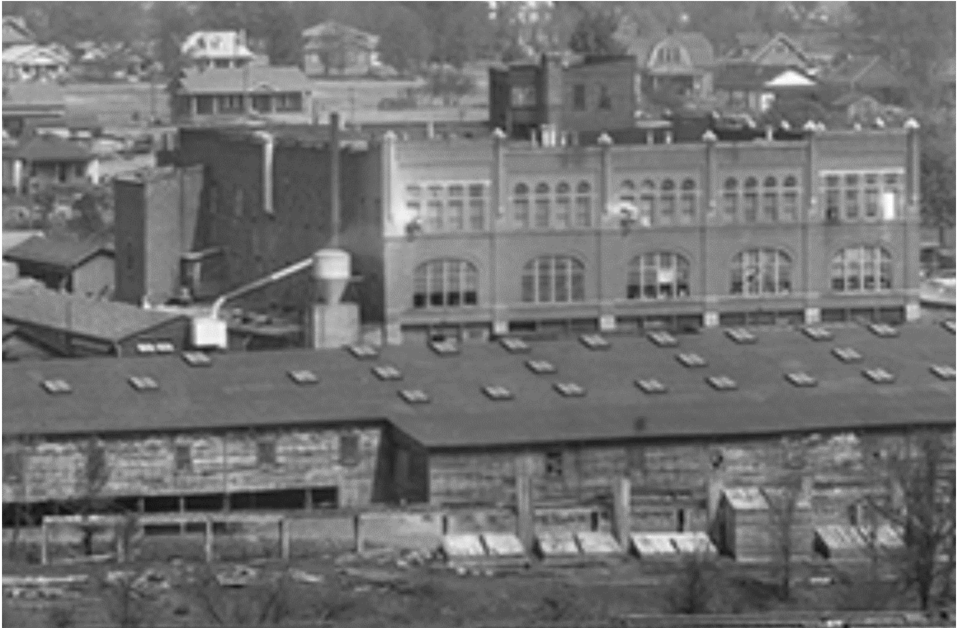
Figure 53C. A detail of the Empire Chair Company, which occupied the Wilder Block during the period when this photograph was taken, 1925 to 1928. The low building in the foreground appears to be part of the Empire Chair Company. 258
