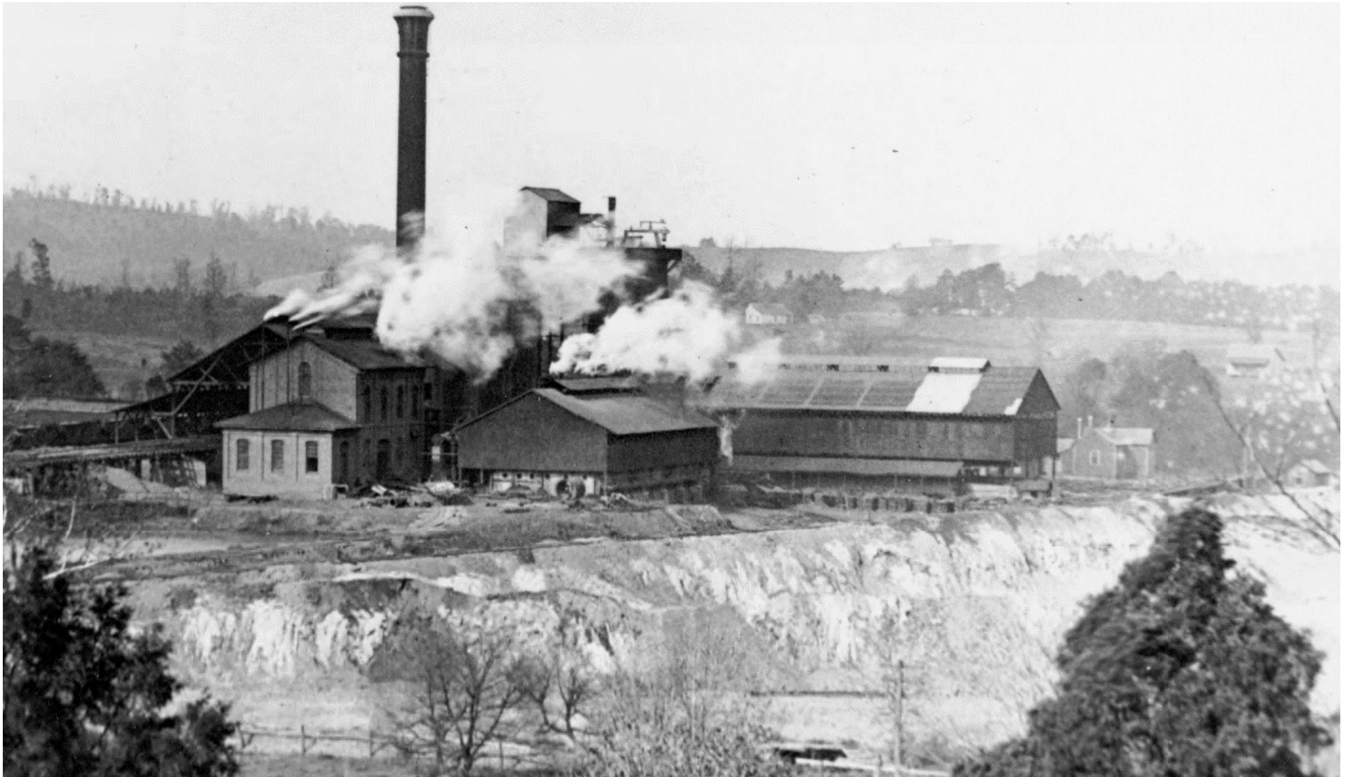
Figure 80A. A detail of the Cranberry Furnace. This image depicts, from left to right, the two-track trestle leading into the “Stock Shed”, the engine house (containing two or three “Steam Blast Engines”, the 160’ chimney, the boiler house (with three boilers) with the ore elevator to the top of the 75’ furnace behind it, the “Cast Ho.” with what appears to be a “Car Shed” (added between 1908 and 1909) beside it, the “Laboratory”, and the small “Oil Ho.” Note that the “Eng. Ho.” and “Shed”, depicted on Map 31B (dated February 1920) have been removed. Also note what appears to be a relatively new section of corrugated roofing on the “Cast Ho.” This photograph appears to post-date Figure 82, which dated to 1919 – 1921. Revised 24 September 2024.
