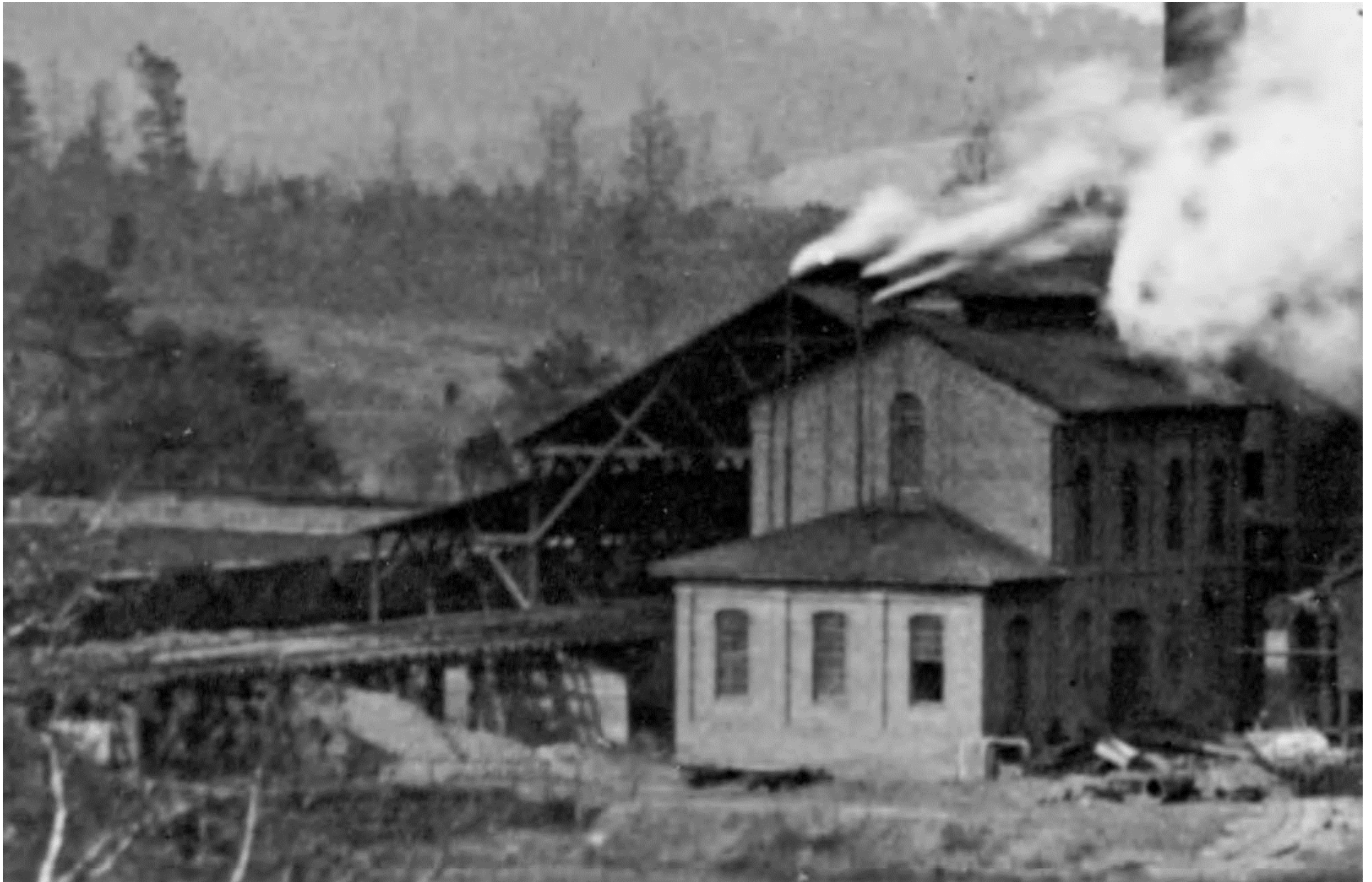
Figure 80B. A detail of the “Stock Shed” and the engine house (containing two or three “Steam Blast Engines”). Note the dual-gauge track and flatcar on the right side of this image.
