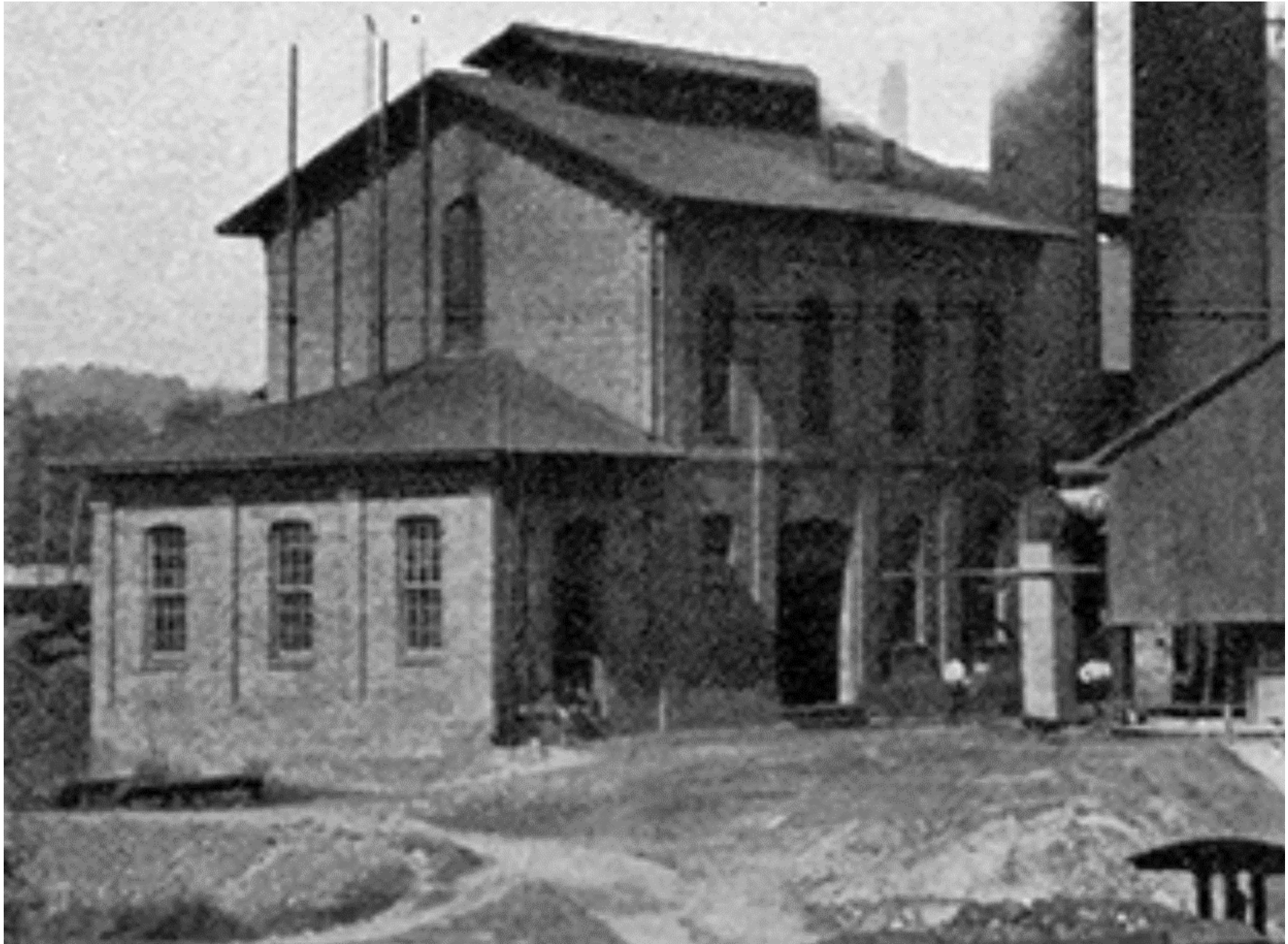
Figure 81A. A detail of the engine house, containing two or three “Steam Blast Engines”.
