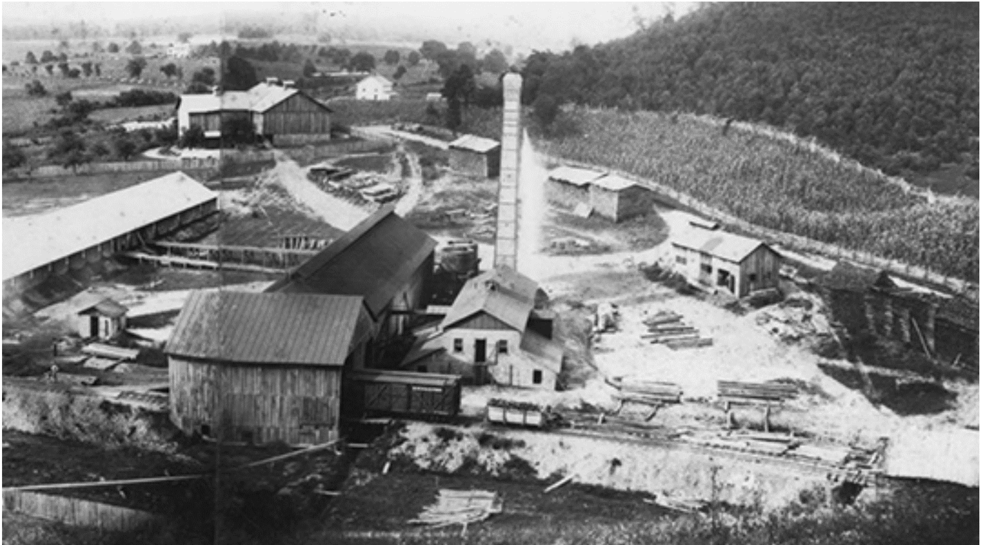
Figure 1B. Another detail of the Watauga Tannery. The building, in the left foreground, with the railroad track through it, appears to be the “Leach Ho.” (labeled “H” on Map 3A), note that it does not appear to be as long as it was at the time the map was made and also note that only two (not three) elevated water tanks are present in this photograph, to the right of the “Leach Ho.” The building to the immediate right of the “Leach Ho.” appears to be a boiler house (labeled “J”), which had an 85’ high brick chimney, note that Map 3C indicates that this building has been changed since this photograph was taken. “These buildings were probably painted barn red, like most tanneries.” 11 The light-colored building to the right of the boiler house appears to be the “Carp’t’r” building (labeled “K”). The barn in the left background is partially depicted on Map 3A, but the buildings between it and the “Carp’t’r” building are not, perhaps indicating that they had been removed by January 1891.
