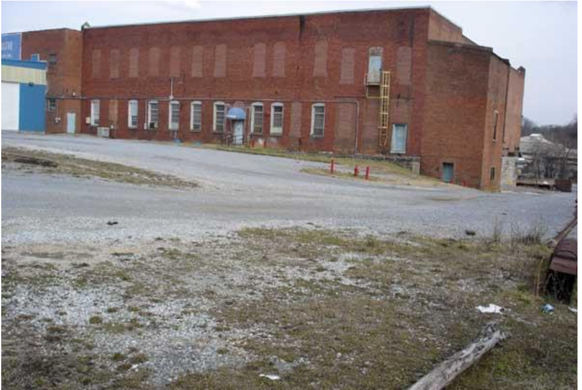
Figure 61. A “recent” view of the east face of the Wilder block. The “Remaining portions of this building were demolished in 2008.” 266
