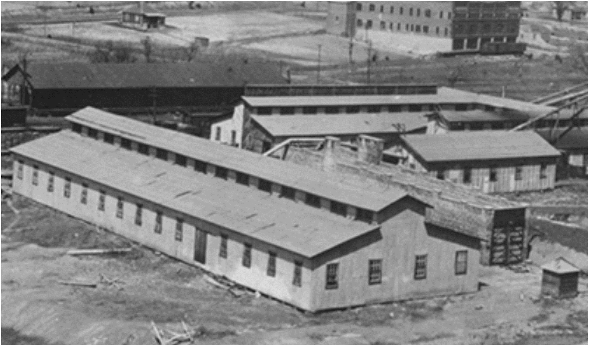
Figure 30A. A detail. In 1920, the “iron clad” building in the left foreground contained the “Bobbin Co. Mill” and “Pearson Loom Supply”. The structure to its right was built of brick and contained the “Dry Kiln”. The small building in the lower right corner appears to have contained 100’ of 2½” fire hose, see Map 15B. The iron clad building with the clerestory roof, closest to the “Old C.C. & O. R.R. Depot”, contained the “Rim Dep’t.” and was attached to the iron clad building that contained the “Bending Dep’t.” The smaller detached building, between the “Dry Kiln” and the buildings with the clerestory roofs, contained the iron clad “Bobbin Fact’y.”, see Map 15C. This photograph appears to date to between 1920 and 1925.
