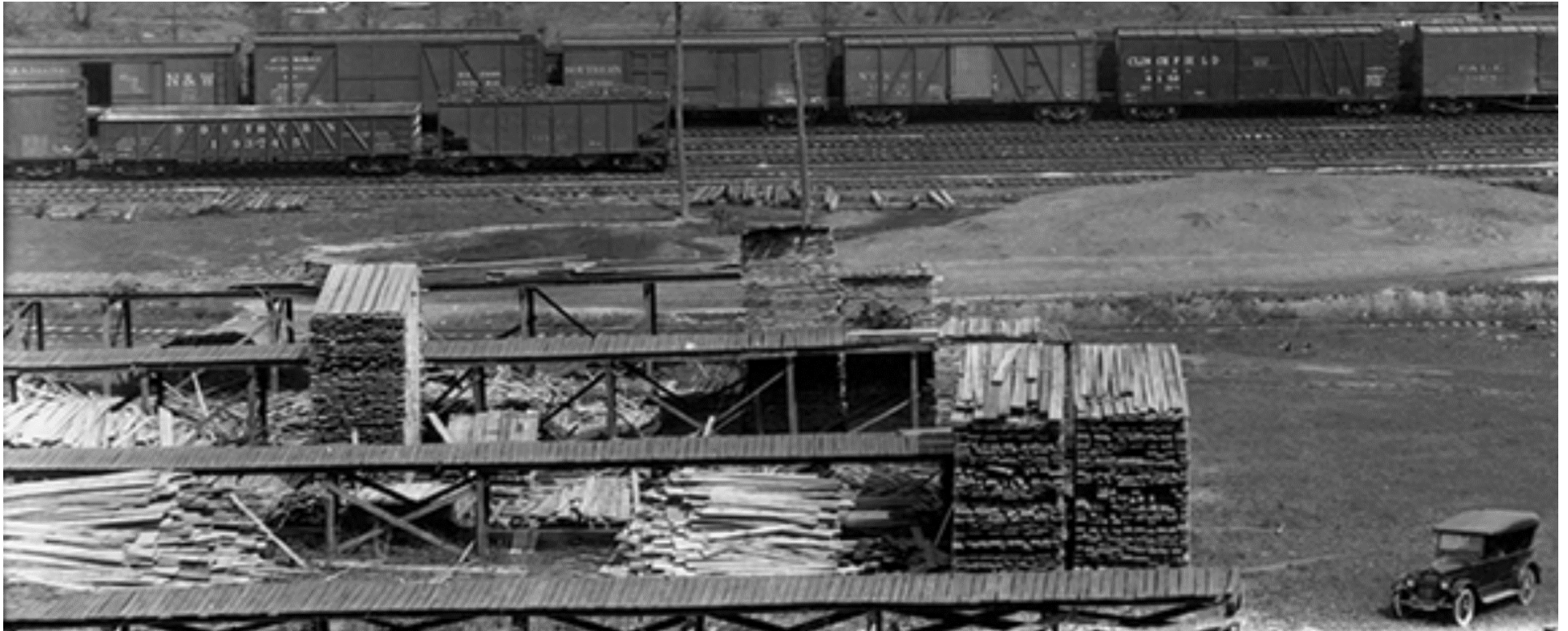
Figure 53A. A detail of what appears to be the lumber yard and platforms on the east side of the Unaka Flooring Company (previously the Southern Bending Company). Note the early model automobile, as well as the N&W, Southern and Clinchfield freight cars in the background. This photograph appears to date to the time between 1925 and 1928.
