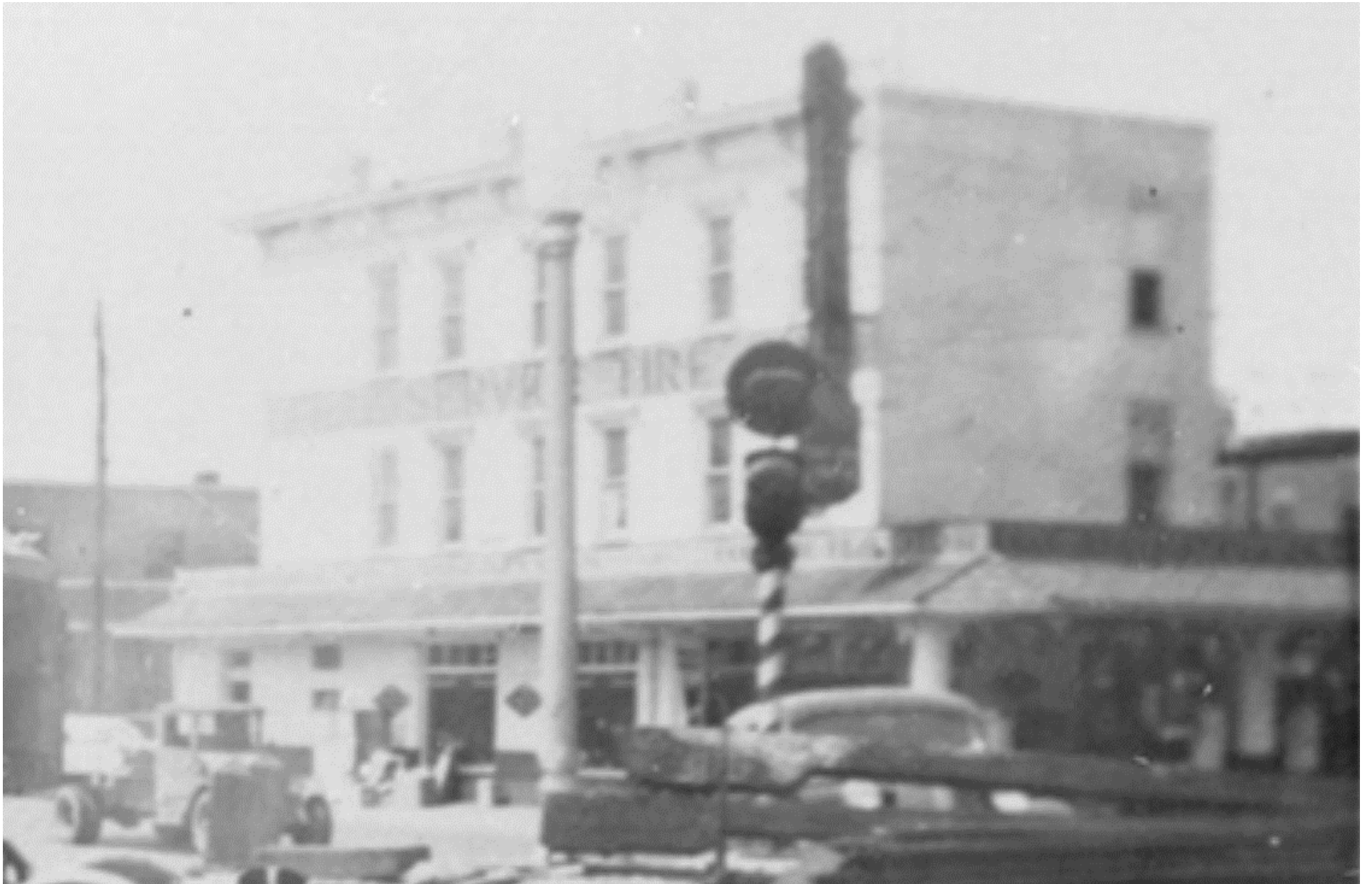
Figure 17. A detail of the Free Service Tire Company. This photograph was taken in September 1946 or later. 28
