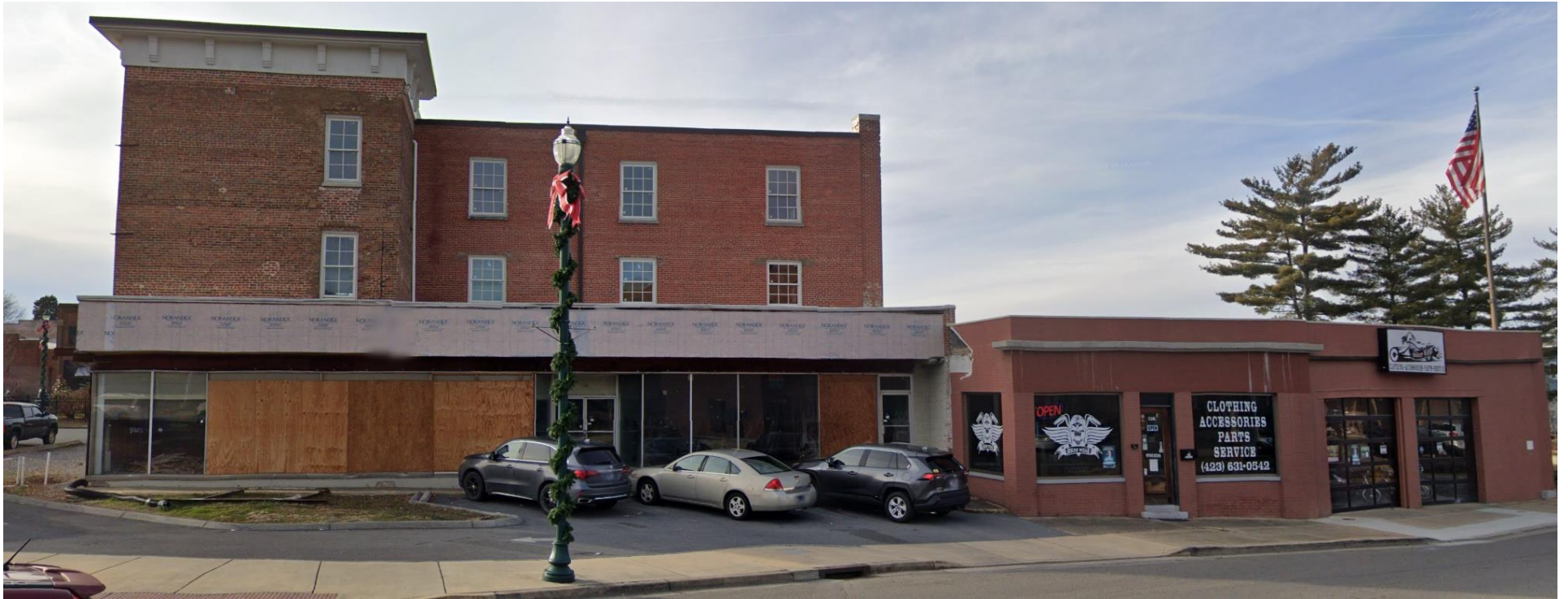
Figure 28. A view of the eastern side of the building formerly occupied by the Free Service Tire Company, in September 2018.
