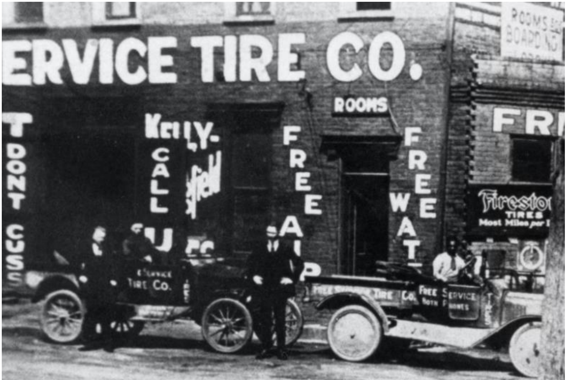
Figure 18B. Another detail, this one of the vehicles. Note the sign at the top right which appears to read in part “Rooms... Boarding...”
