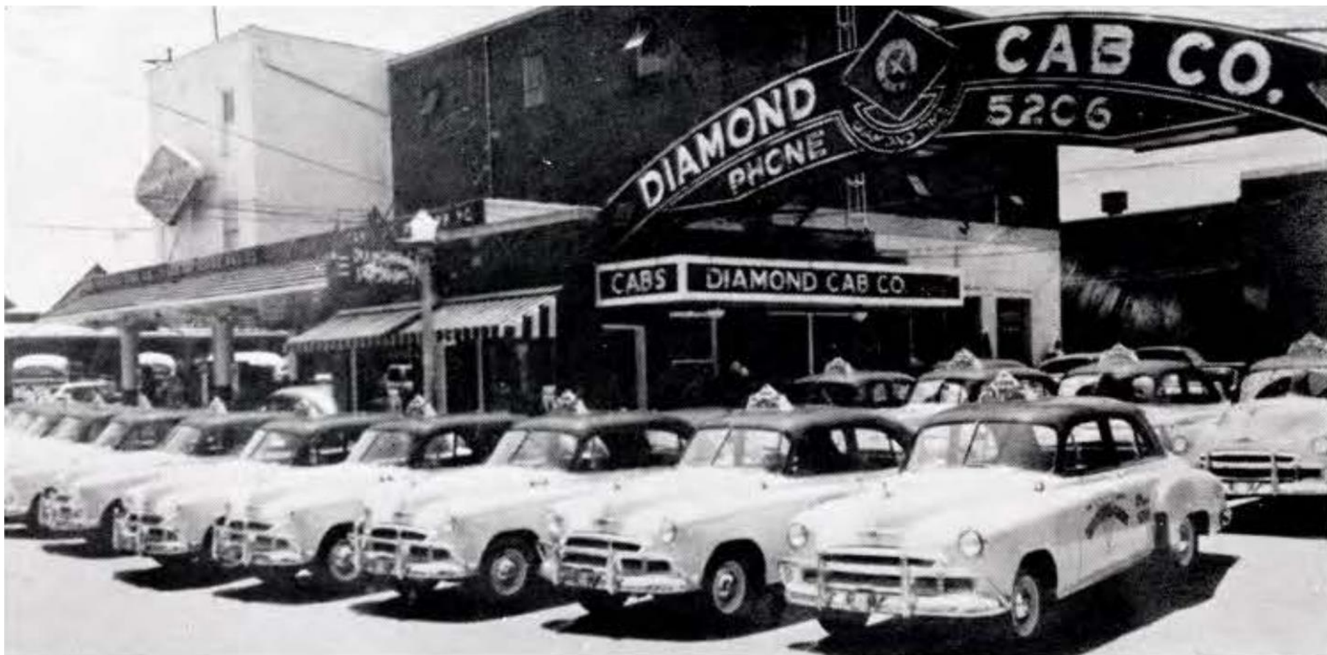
Figure 21. This photograph depicts the Diamond Cab Company, which was at 116 Buffalo Street. Note the view of the north side of the Free Service Tire Company building, which appears to have a Goodyear sign on its east side between the second and third floors. Also note the three-story building between the Free Service Tire Company and the Diamond Cab Company, which appears to have been an addition that was built on top of a single - story building that was attached to the Fire Service Tire Company building between 1941 and 1946. The Diamond Cab Company was at this location by 1942 and remained here until at least 1959. This photograph dates to 1952 or earlier. 32 See Figure 6A.
