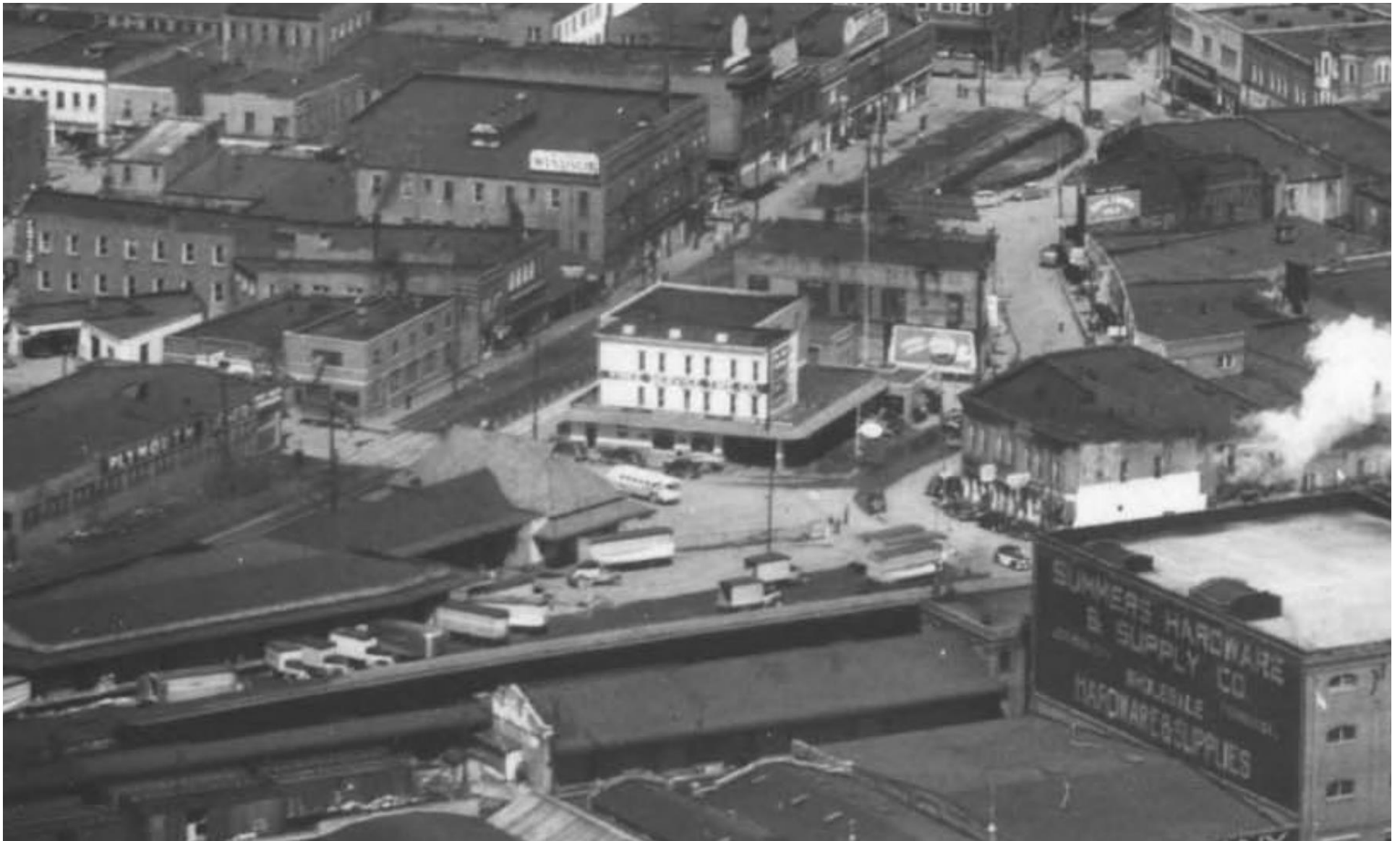
Figure 4. An aerial view of the Summers Hardware & Supply Company building, Clinchfield depot (just behind Summers Hardware), E.T. & W.N.C. depot (surrounded by tractor trailers), the Automobile Sales and Service Company (with the Plymouth and Desoto sign, on the left), Free Service Tire Company (the light-colored building near the top center of the image), the W.O. Phillips building (behind and to the right of the Free Service Fire Company, by what appears to be a Pepsi-Cola sign), and the William Harr building (just above Summers Hardware), on 1 March 1947. 10
