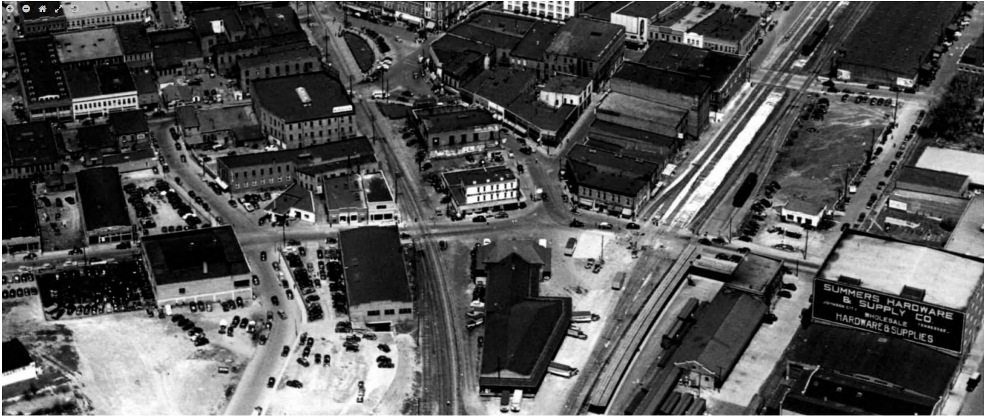
Figure 3. This aerial view, looking northeast, includes (along the bottom of the image from left to right) the “Automobile/Auto Sales and Service Co. 103 Wilson Ave... Distributors for De Sotos and Plymouths” (just to the left of the Southern Railway mainline), the E.T. & W.N.C. depot, the Clinchfield depot, now with a curved platform to its left, and the Summers Hardware & Supply Company. Near the middle of the image is the light-colored Free Service Tire Company building (just above/behind the E.T. & W.N.C. station), the W.O. Phillips building (behind the Free Service Tire Company building), and the William Harr building, to the right. This photograph was taken on 19 April 1941. 9
