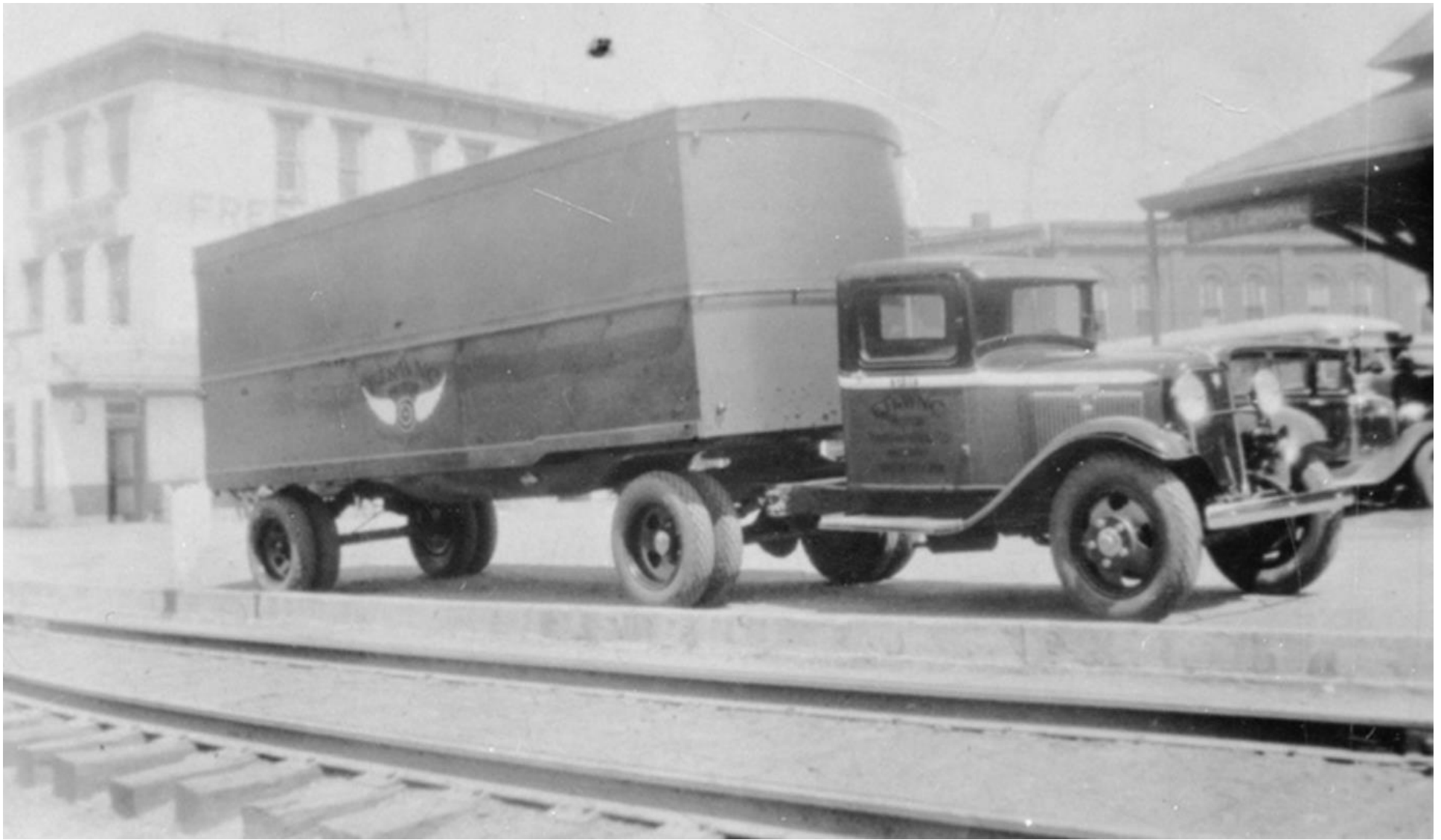
Figure 7. A tractor (which appears to be No. 125) with a trailer. Note the Free Service Tire Company building on the left, and the William Harr building and E.T. & W.N.C. depot on the right. Tractor No. 125 was acquired in August 1934 and was wrecked on 31 July 1938, which would indicate that those photograph dates to between 1934 and 1938. Since the tractor looks new, this photograph may have been taken about the time of the tractor's arrival in 1934. 14 See Map 6A.
