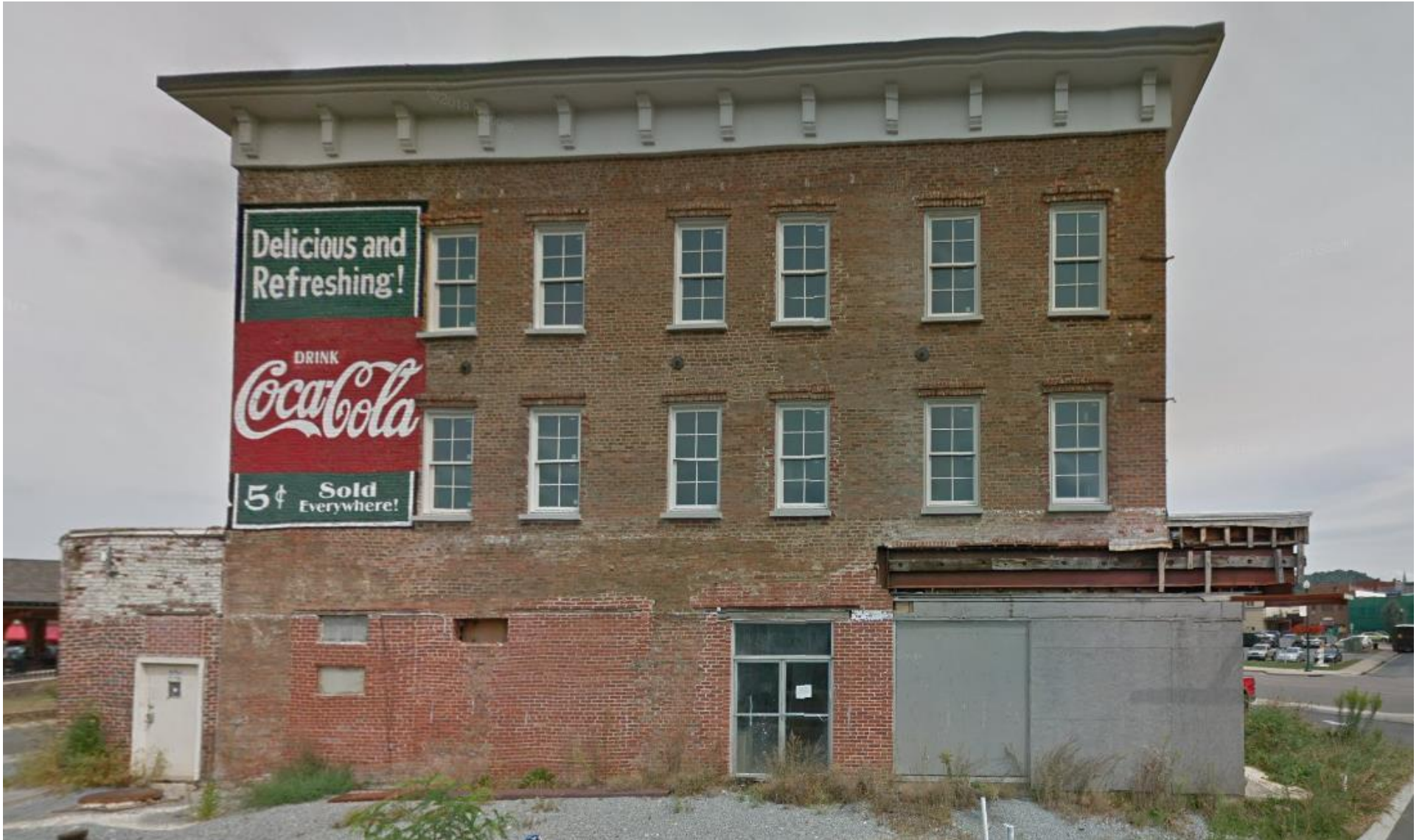
Figure 25. A view of the southern side of the building formerly occupied by the Free Service Tire Company, in September 2018. Note that the windows on the second and third floors have been restored. Also note that the trim along the roofline have been restored since the image in Figure 24 was taken in 2012. Finally, note that the white paint has been removed.
