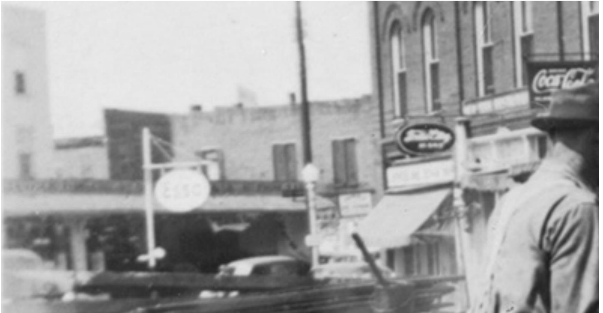
Figure 98. This view shows, from left to right, a portion of the Free Service Tire Company building, the W.O. Phillips building (with its shutters closed), and the William Harr building, after September 1946. Note the Esso sign near the center of the image, as well as what appears to be the “New York Restaurant” sign to the left of the Coca-Cola sign. 80
