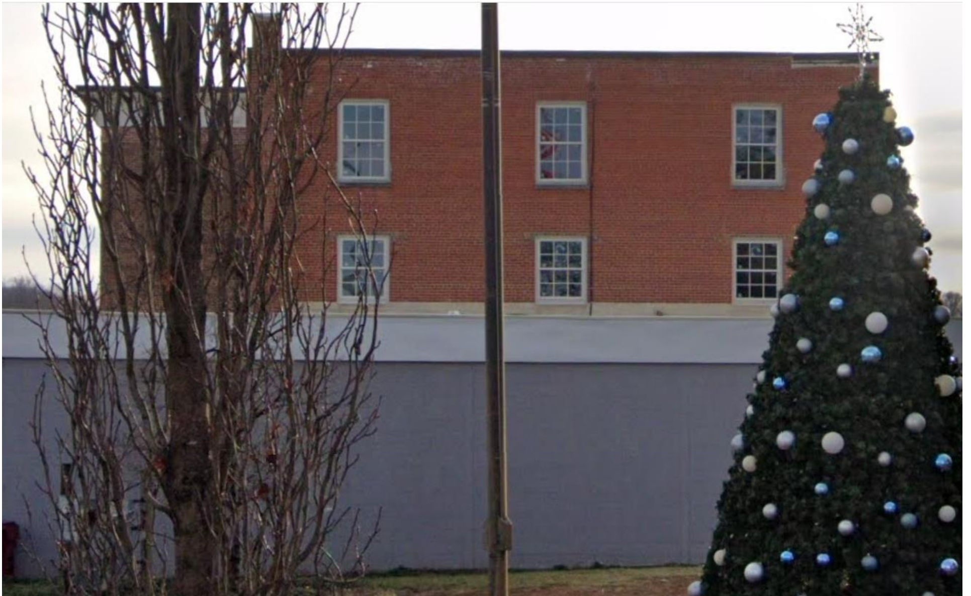
Figure 30. A view of the northern side of the three-story addition to the building formerly occupied by the Free Service Tire Company, in January 2024.
