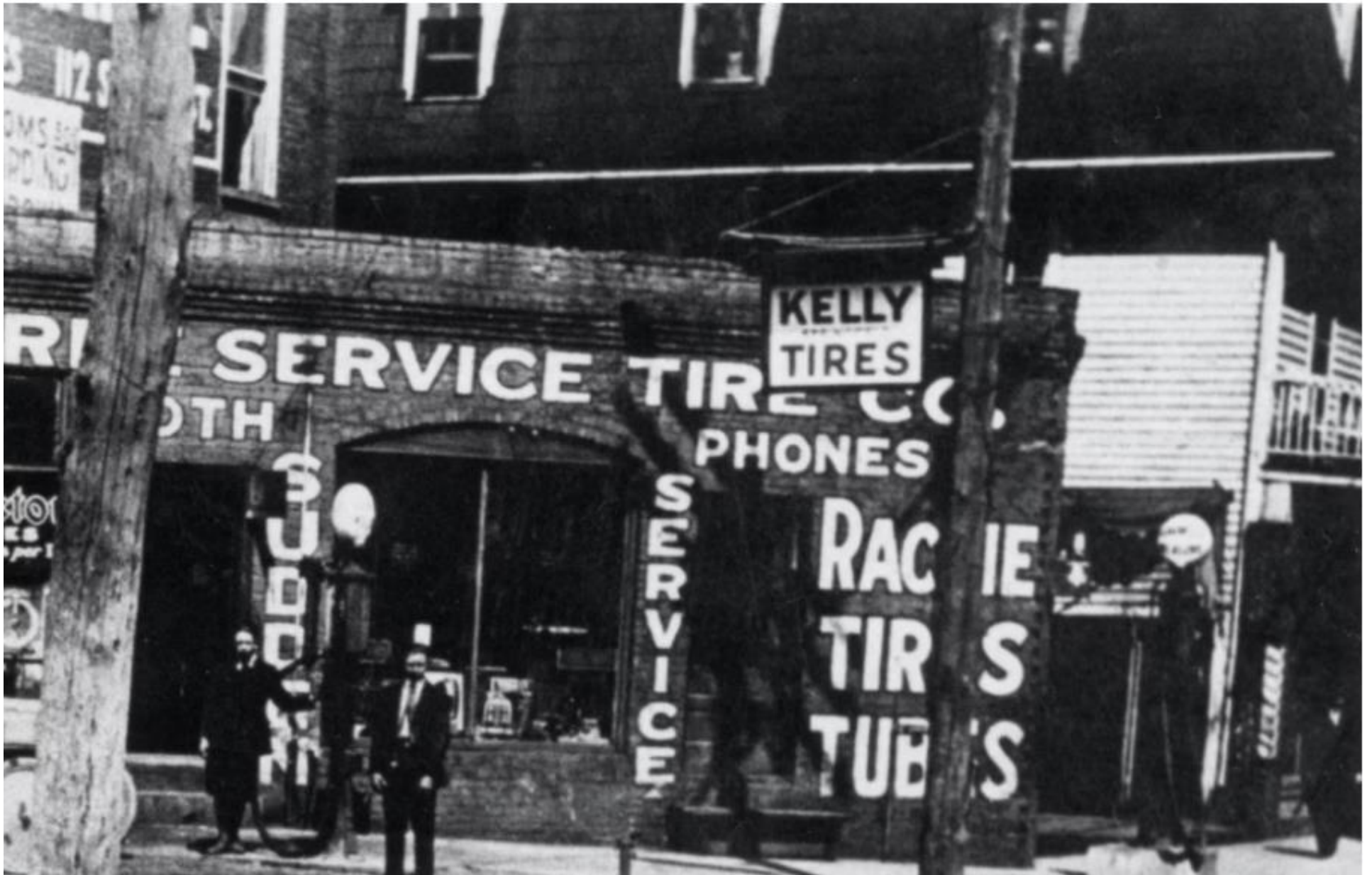
Figure 18D. A detail of the portion of the Free Service Tire Company building at the corner of Wilson and Buffalo streets. The building in the right background appears to be the Western Hotel, formerly the Hotel Piedmont, which was demolished in 1927. Reportedly, this photograph dates to the early 1920s.
