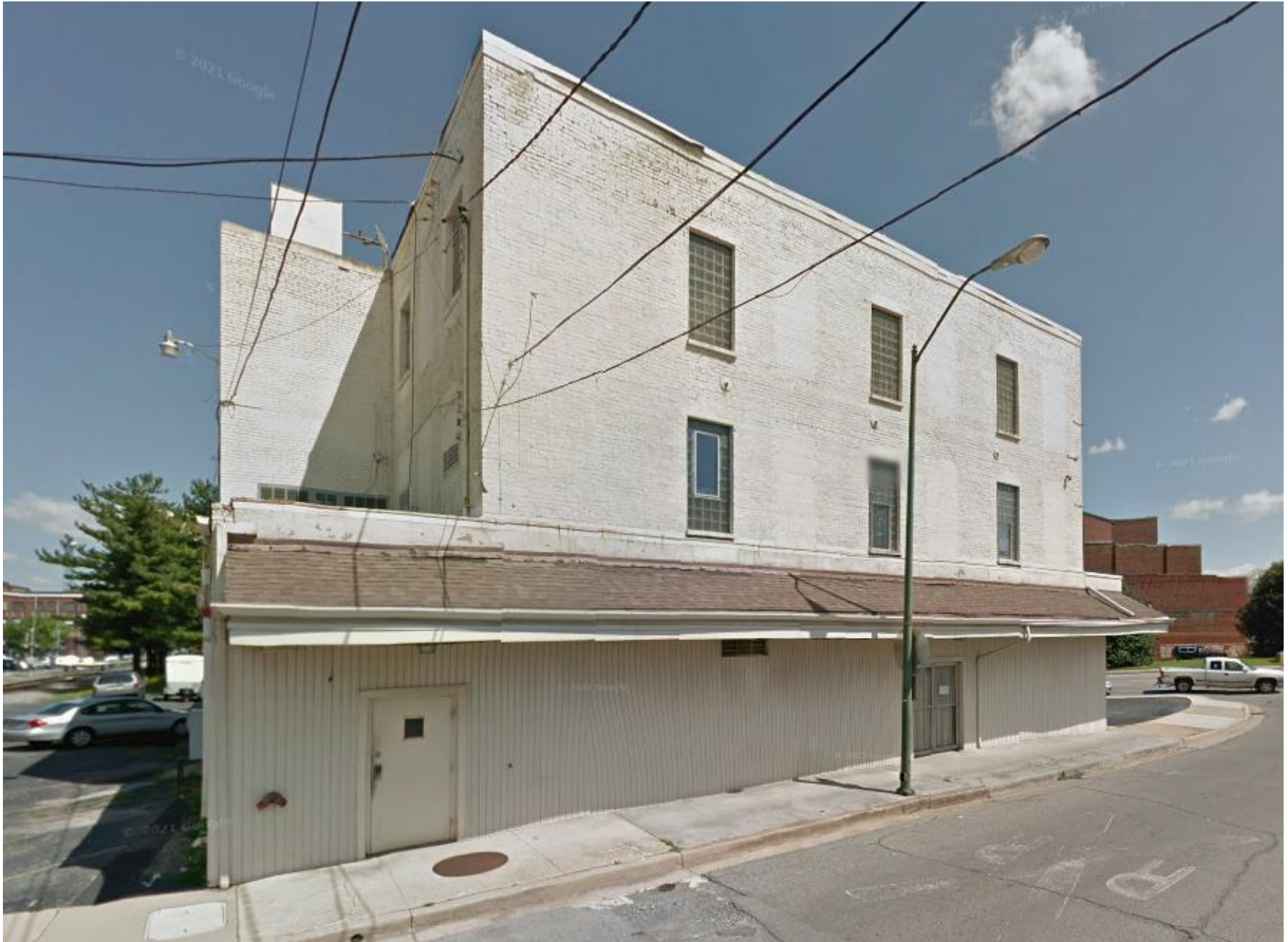
Figure 24. A view of the southern side of the building formerly occupied by the Free Service Tire Company, in April 2012.
