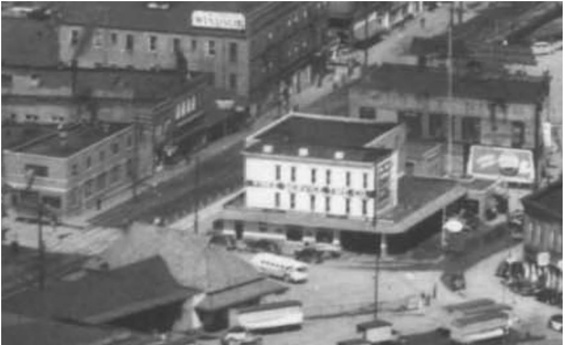
Figure 4A. A detail, note that there is a three-story addition to the Free Service Tire Company building and what appears to be a single-story building on the ground that was previously occupied by the Hotel Piedmont. 11 Apparently, this building was occupied by the Diamond Cab Company at this time. Also note the building across the railroad tracks from the Free Service Tire Company, at 100 Wilson Avenue, which housed their recapping plant.
