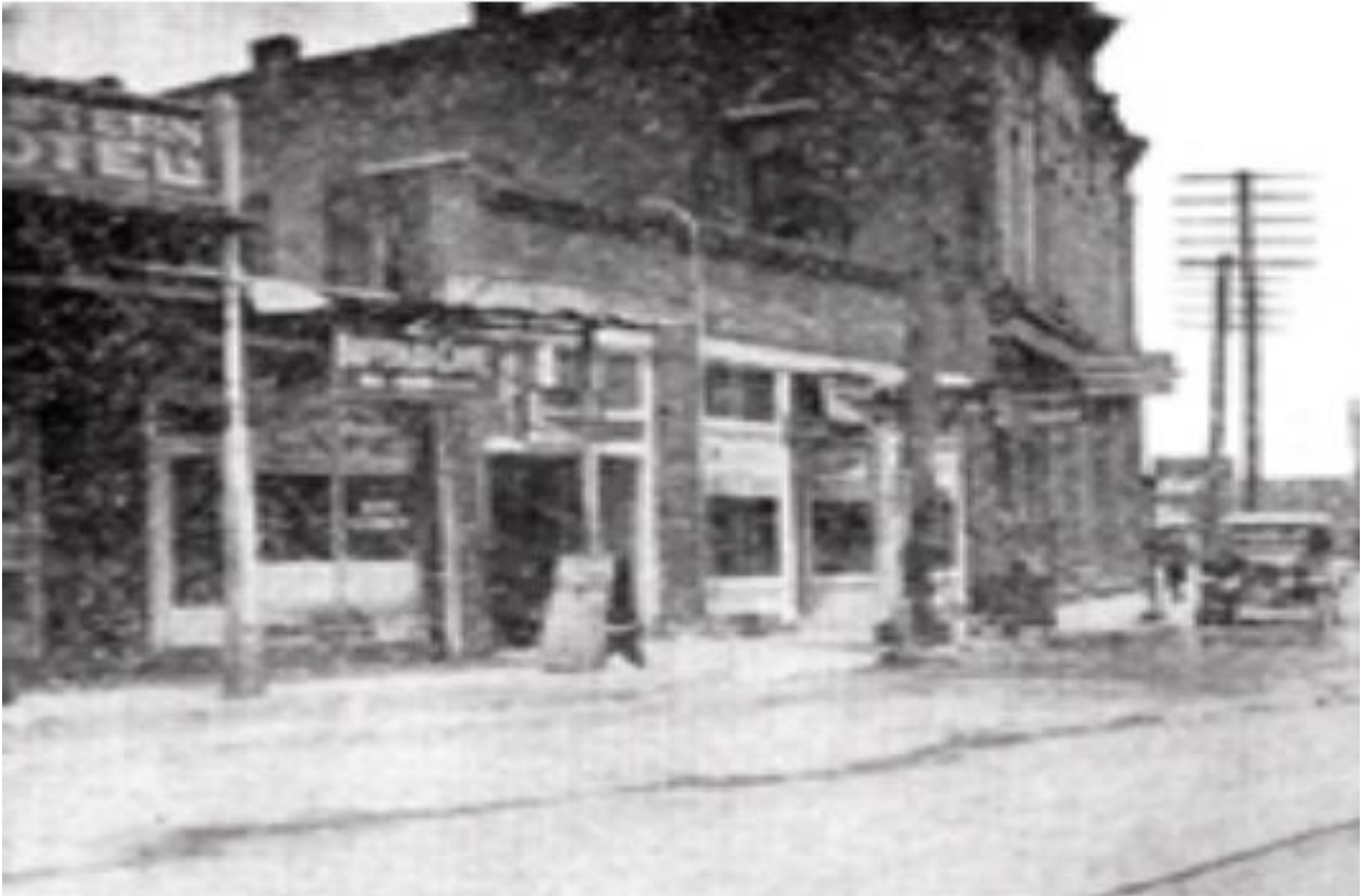
Figure 65A (reproduced here for convenience). The portion of the two-story building visible in this image is of the south and east sides of the W.O. Phillips building. The road on the right is Buffalo Street.
