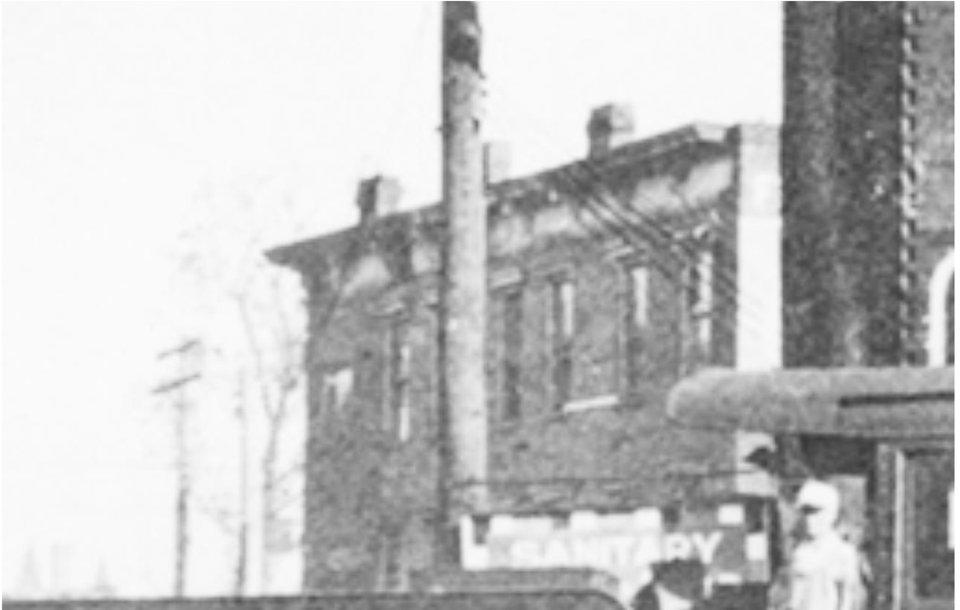
Figure 13A. A detail of the Free Service Tire Company building. The Sanborn Fire Insurance Company map for this area in February 1920, shows a barber shop at 213 Buffalo Street (northeast corner of Buffalo and Jobe streets). In 1923, Old Hickory included an advertisement for the “Sanitary Barber Shop... Buffalo Street – Near C.C. and O. Ry. Station”, with other advertisements appearing until at least 1925. 23
