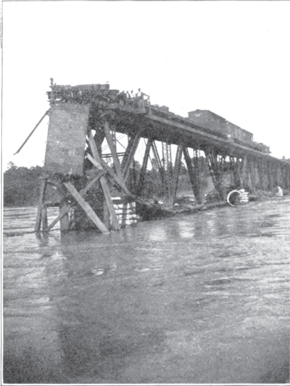
WRECK OF BRIDGE ON THE SOUTHERN RAILWAY OVER THE CATAWBA RIVER; PART STANDING WAS SAVED BY RUNNING LOADED CARS UPON IT.
