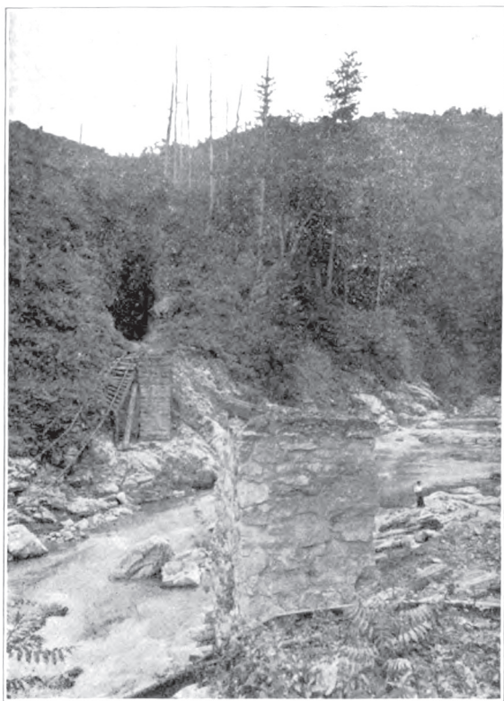
WRECK OF A RAILROAD BRIDGE, DOE RIVER, TENN.
