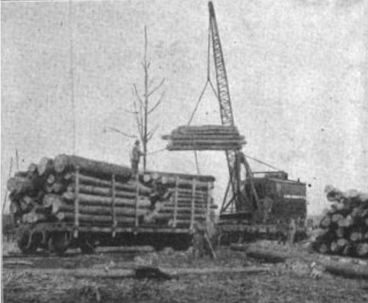
Figure D – 1. “The Raymond Gasolene Log Loader”, American Lumberman , 19 July 1919. 123
