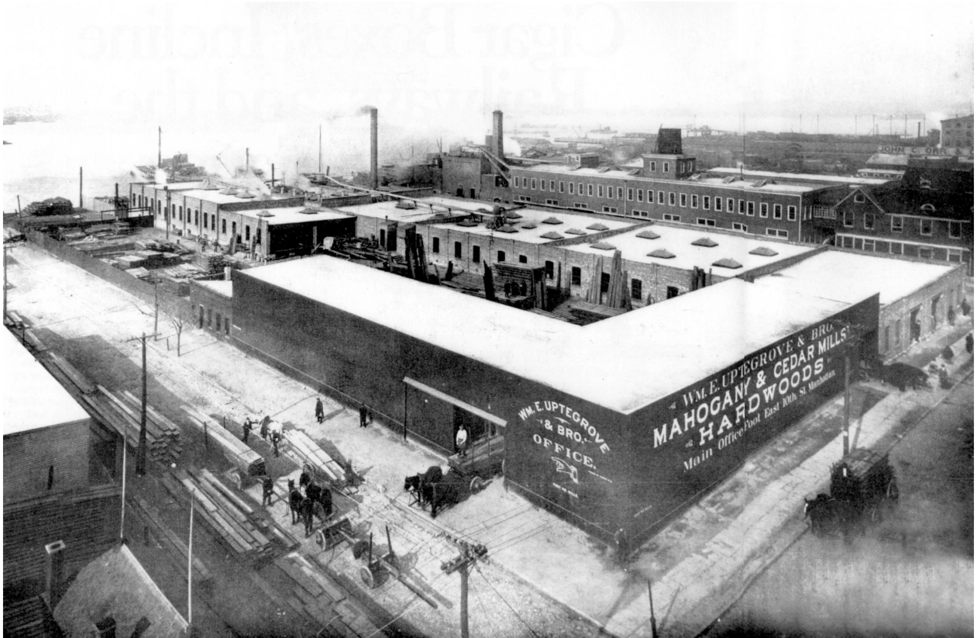
Figure G-4. "Uptegrove's Brooklyn manufacturing plant occupies a full city block on the waterfront. It includes a sawmill, kilns, and warehouses. Photo from The American Lumberman , May 23, 1903, courtesy of Mac Connery." 302
