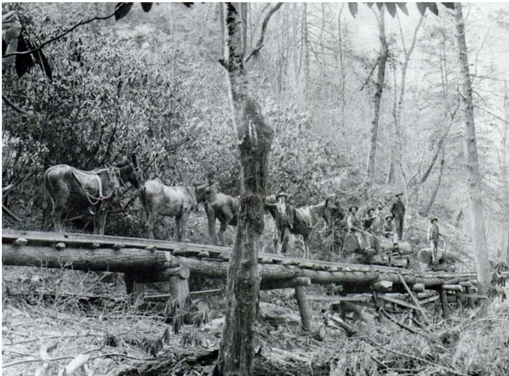
Figure H-3. “Timber operators built tram roads into the dense laurel thickets on Unaka Mountain in order to access certain types of trees. The wooden rails of this tram road rest on a low trestle that spans the uneven terrain. Notice that the mules and horses used to pull the railcars loaded with logs. (Courtesy of Chuck McInturff.)” 324
