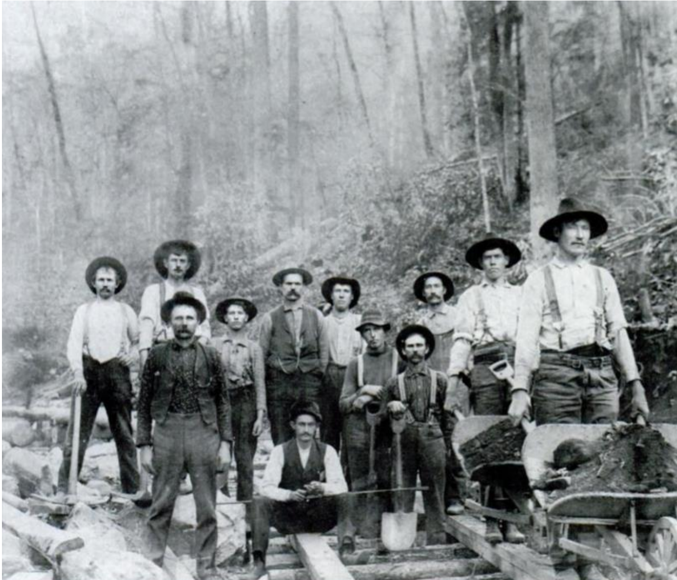
Figure H-2. “Hauling timber off Unaka Mountain required building rail spurs into the woods. Often these narrow-gauge spurs, winding across steep hillsides and over ravines, were constructed of wood, as pictured here. Laborers dug the track bed with picks and shovels, and hauled the dirt away in wheelbarrows with wooden wheels. (Courtesy of Chuck McInturff.)” 323 Of note, neither this figure, nor the following four, were specifically attributed to the Uptegrove operation, based at Unicoi. They are included only because they might be representative of the Uptegrove operations.
