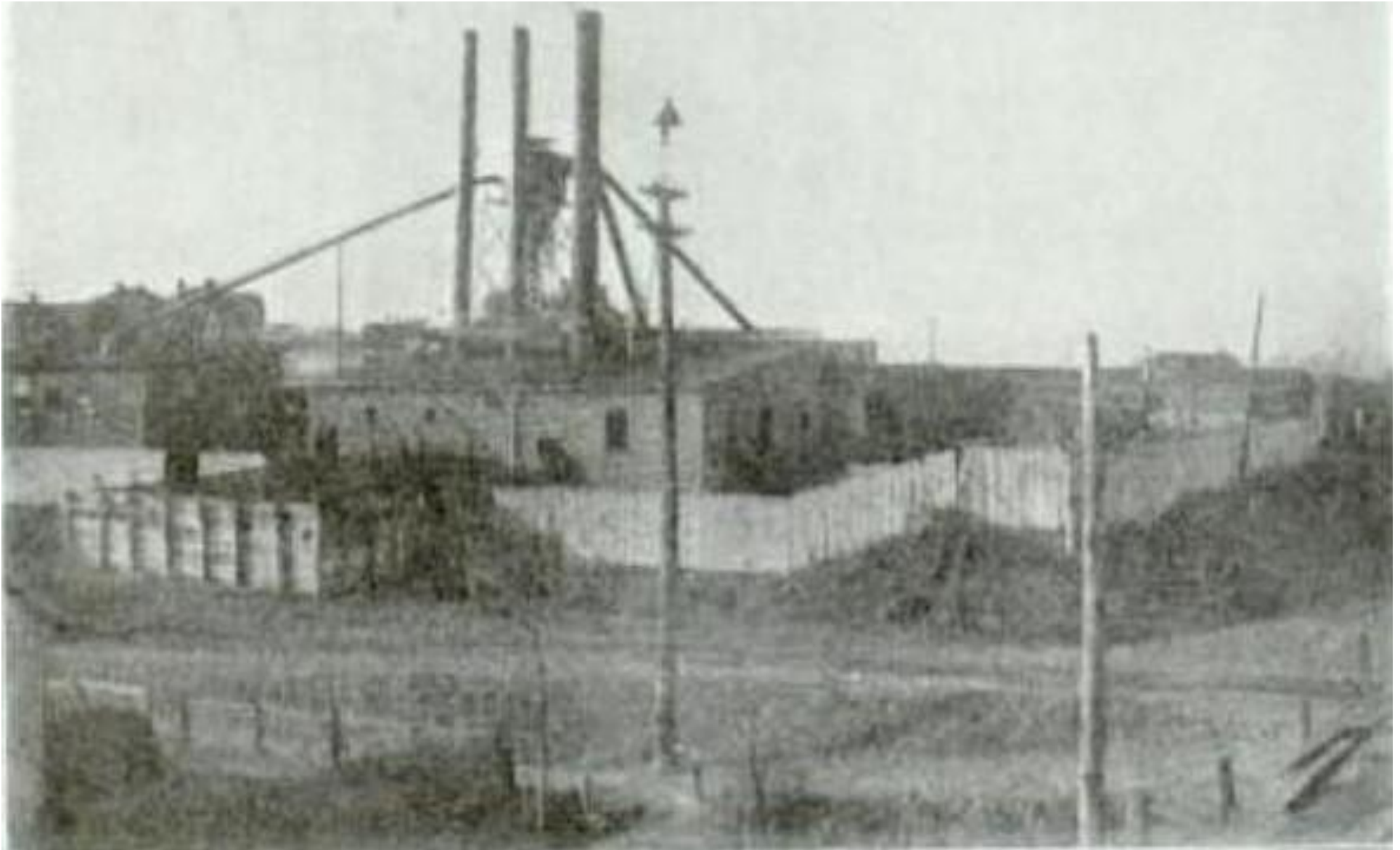
Figure 31. “Plant of the American Cigar Box Lumber Company”, by 1909. 120 This appears to be a view of the plant after the 1906 fire and the resulting reconstruction. This view seems to be looking west, across Division Street at the boiler room (center, with the three smokestacks), a coal bin, and the “Shook Department” (left), see Map 6A, as well as figures 51 and 52.
