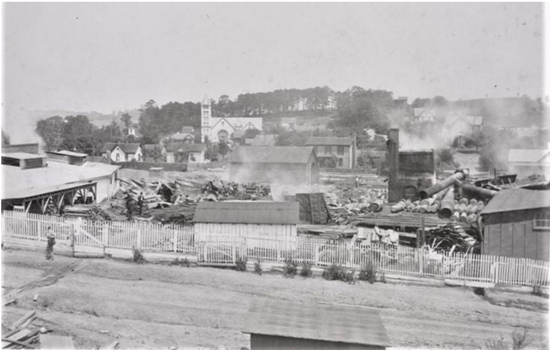
Figure 28. This photograph appears to show the remains of the American Cigar Box Lumber Company after the fire of 12 July 1906. Note the two-stall E.T.&W.N.C. R.R. engine house, the E.T. &W.N.C. R.R. mainline, and the First Christian Church, on East Main, between S. Roan and Division streets. Also of interest is what appears to be the remains of a boiler or furnace. 110 See also Map 4 and figures 12, 13, 17, and 58.
