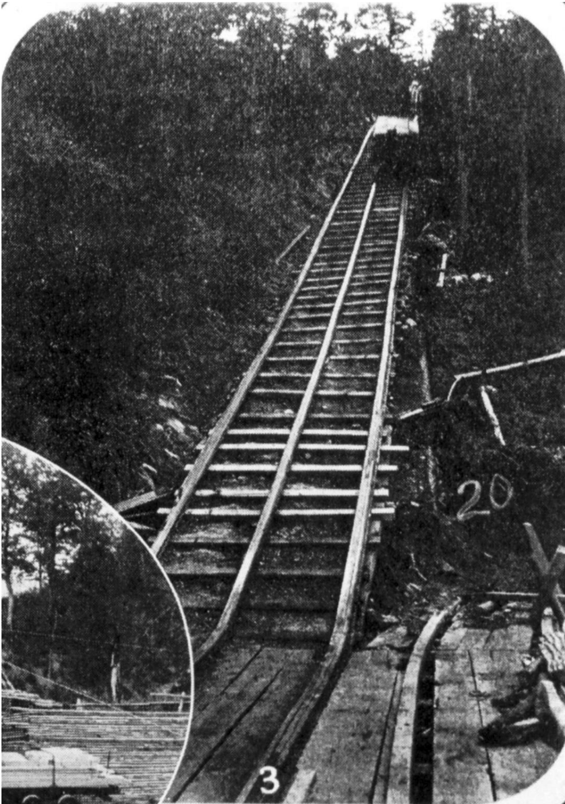
Figure 8. “(3) a car loaded with lumber being lowered down one of the upper sections of the incline railway”, apparently on wooden rails. Historian Thomas Feters captioned this photo: “The 3-railed upper incline has a loaded car descending...” 59 Note that the rails on the incline appear to be made of wood, rather than iron.
