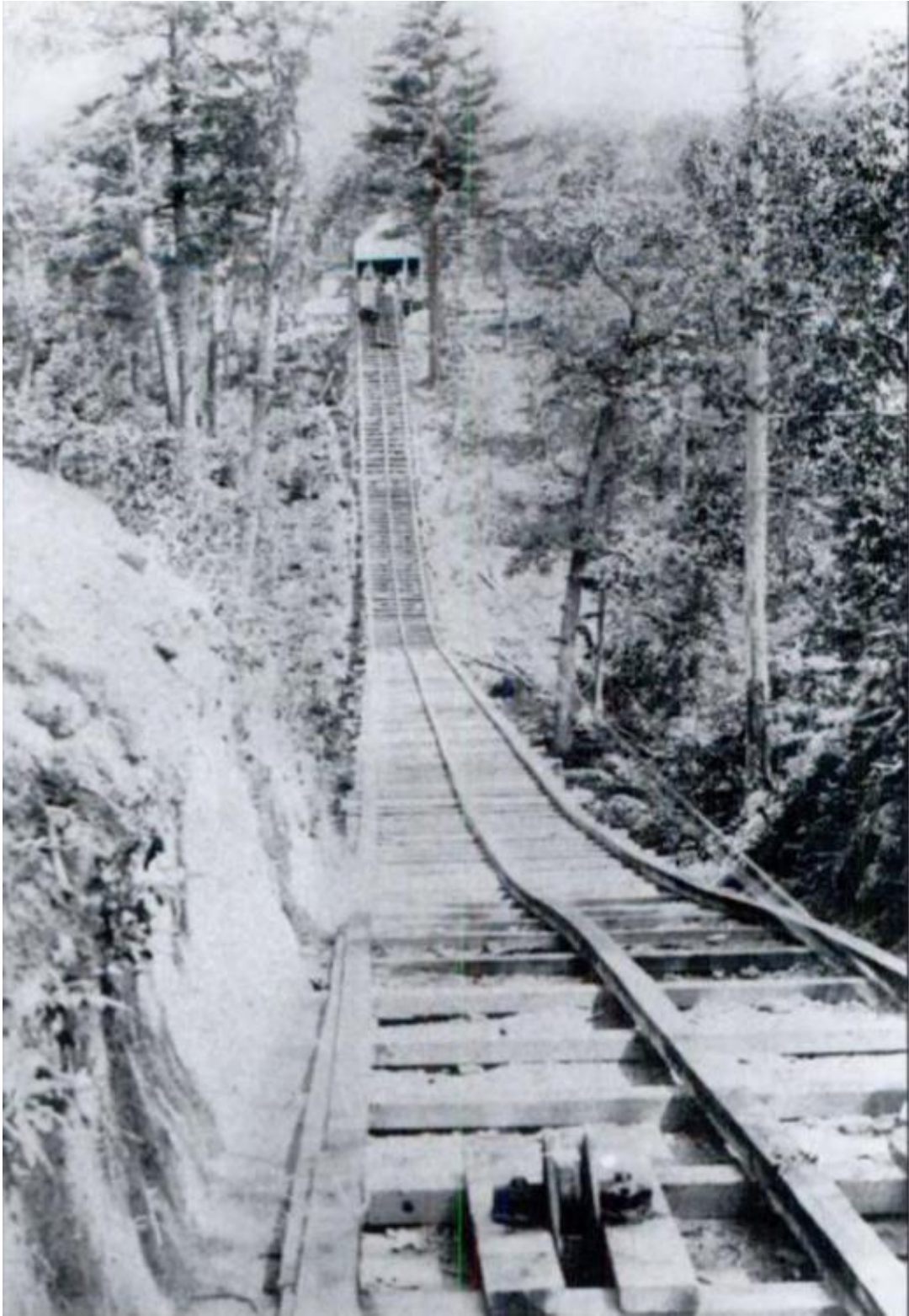
Figure H-4. “The Unaka Mountain timber operations required constructing railway inclines such as this one up the steep mountainsides. The tiny building at the head of the incline is the same building shown in the picture below, even though the curve at the top of the incline is not apparent from this perspective. Notice the cable pulley at the end of the rails pictured here. Cables were used to pull loads of lumber up steep inclines and to lower loads of lumber down them. (Courtesy of Archives of Appalachia, East Tennessee State University.)” 325 Note that the rails appear to be made of wood.
