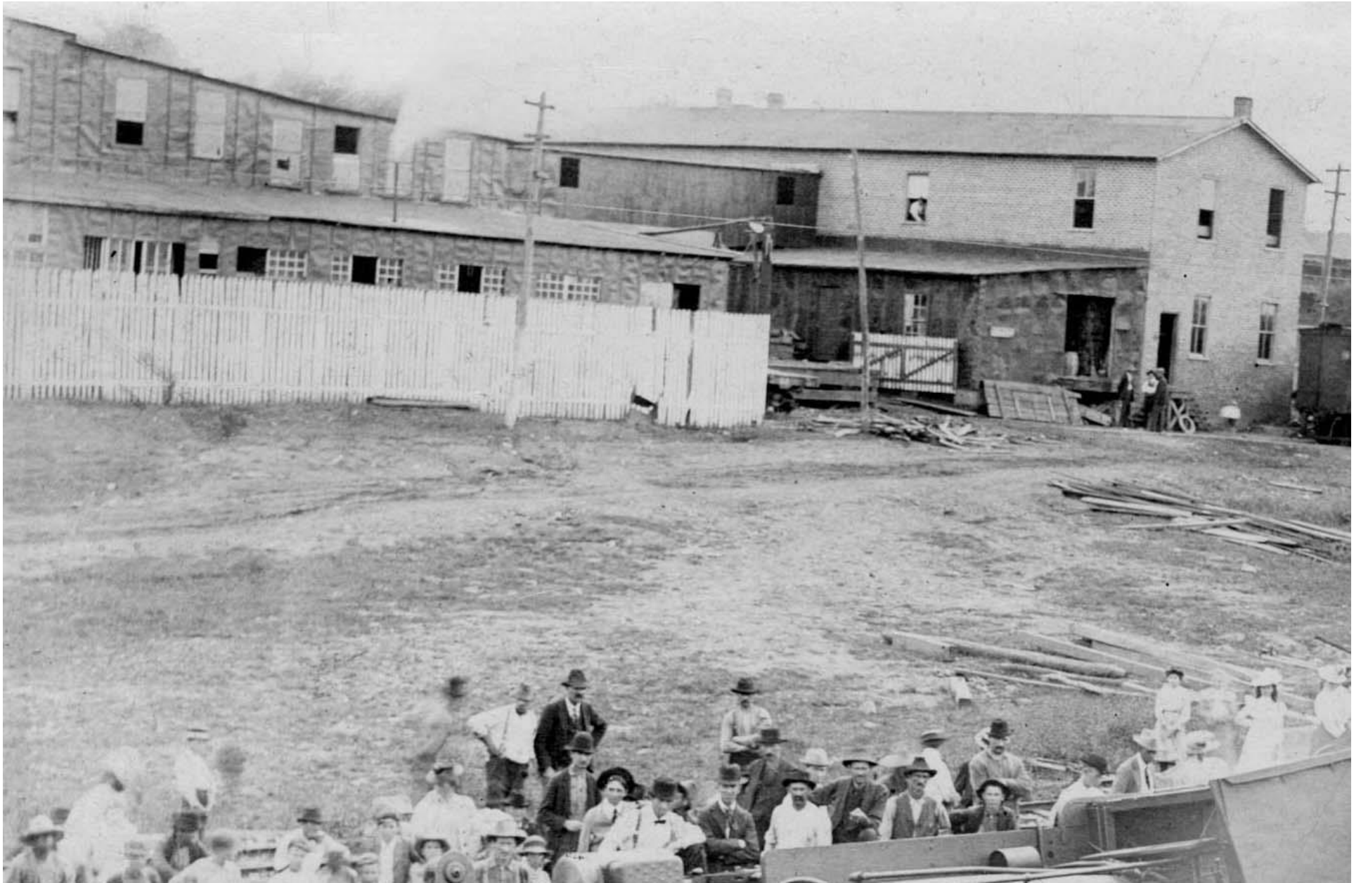
Figure 12A. A detailed view of the American Cigar Box Lumber Company's mill (left) and office/warehouse (right). The second floors of these two buildings were joined by a hallway (which is visible in this photograph). See Map 4.
