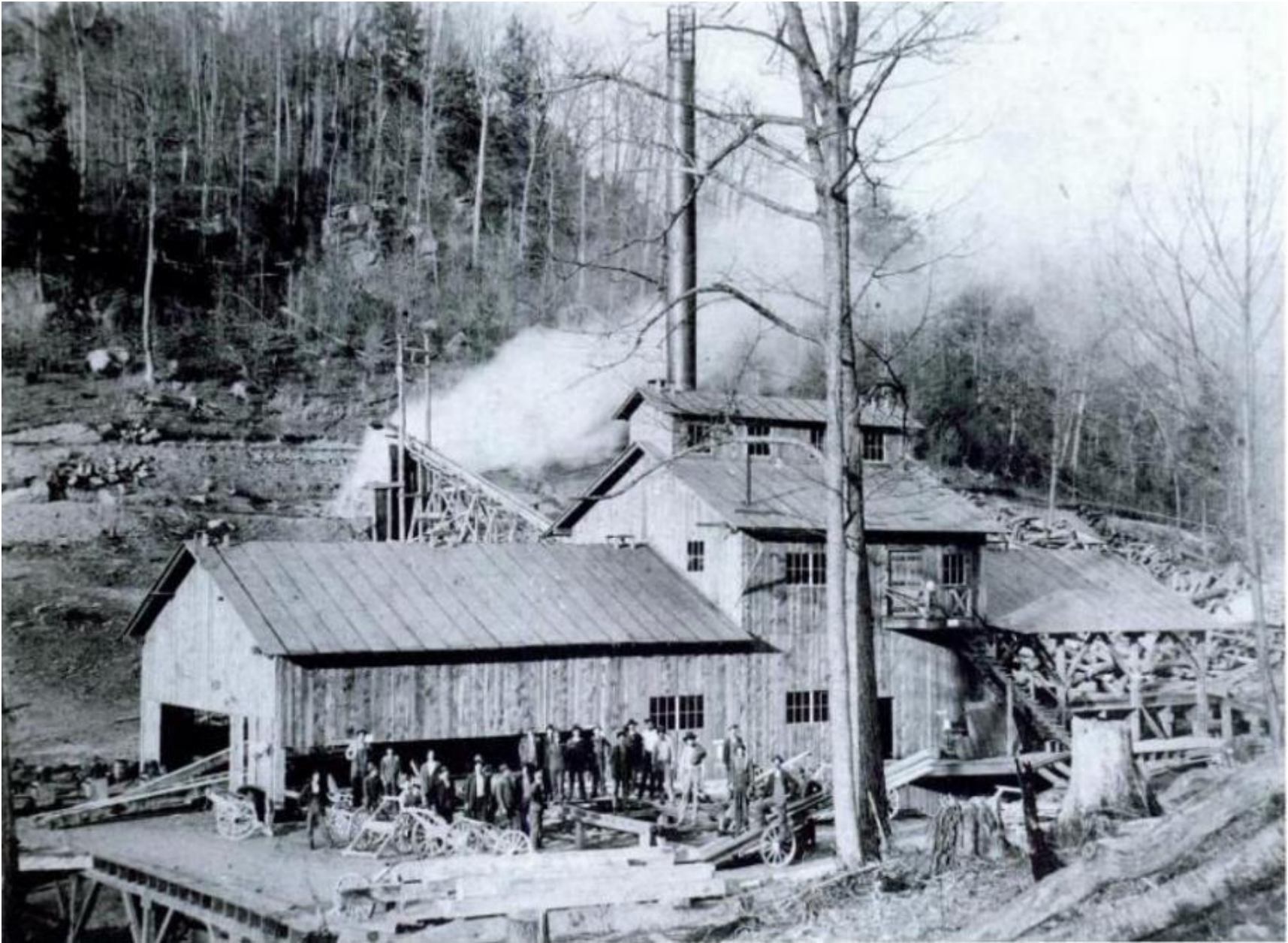
Figure 16. “Twenty-seven employees of H.S. [H.L.?] White Lumber Company pose outside the company’s small single-band mill, c. 1920 [should probably read “1911, or so]. The mill is located on Elk River three miles north of Elk Park. Photo by John Strickland, Bill Richardson Collection. (Copy photo by Cliff Ward).” 48
