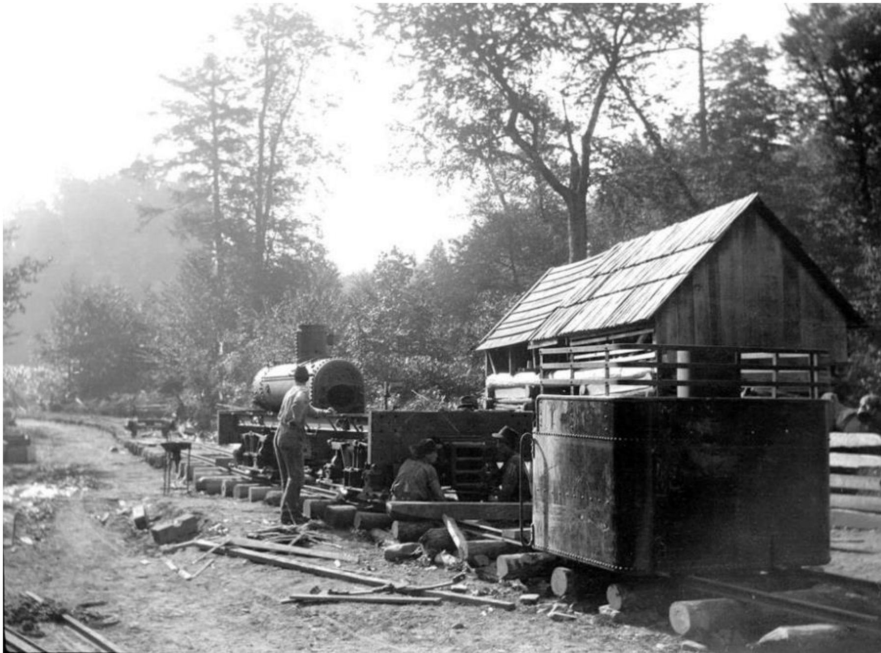
Figure 7. This and the following four photographs appear to be of White Lumber Company #1 (a Shay locomotive with Shop Number 2195). 28
