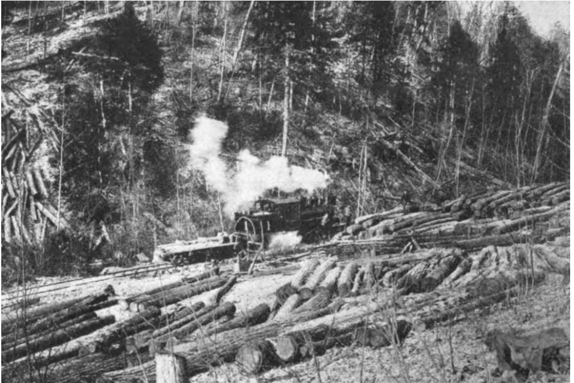
Figure 13. 24 March 1906. American Lumberman : “Whiting Manufacturing Company – hardwood logs and logging engine”, Climax #1 (Shop Number 608) working to supply logs to the Whiting band mill at Abingdon, Virginia. 31
