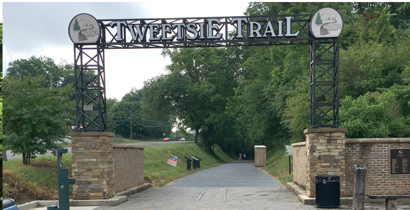
Trail Head next to Legion Street in Johnson City. Note the short section of rails in the trail.
