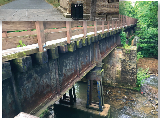
Buffalo Creek Bridge heading towards Bemberg.
